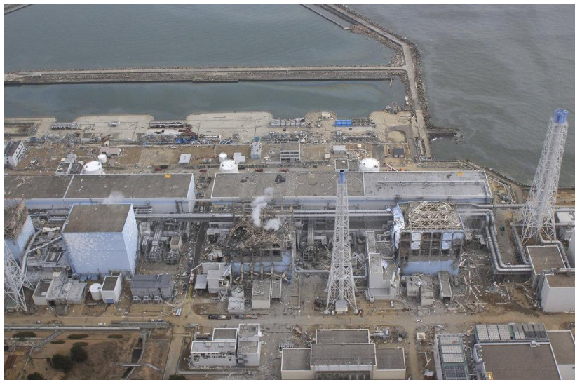
This March 20, 2011 image taken by the Air Photo Service UAV shows a wide shot of the crippled Fukushima Daiichi nuclear power plant, from left; Unit 1 (partially seen), Unit 2, Unit 3 and Unit 4.
