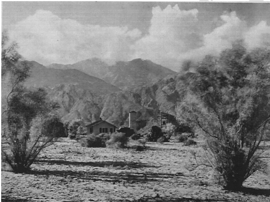
A view of the Araby Tract office and water tower as featured in the Araby Tract sales brochure, Our Occidental Araby . A key selling feature of the tract was the 10,000 feet of water pipe improvements that delivered good water pressure. Source: Palm Springs Historical Society.
