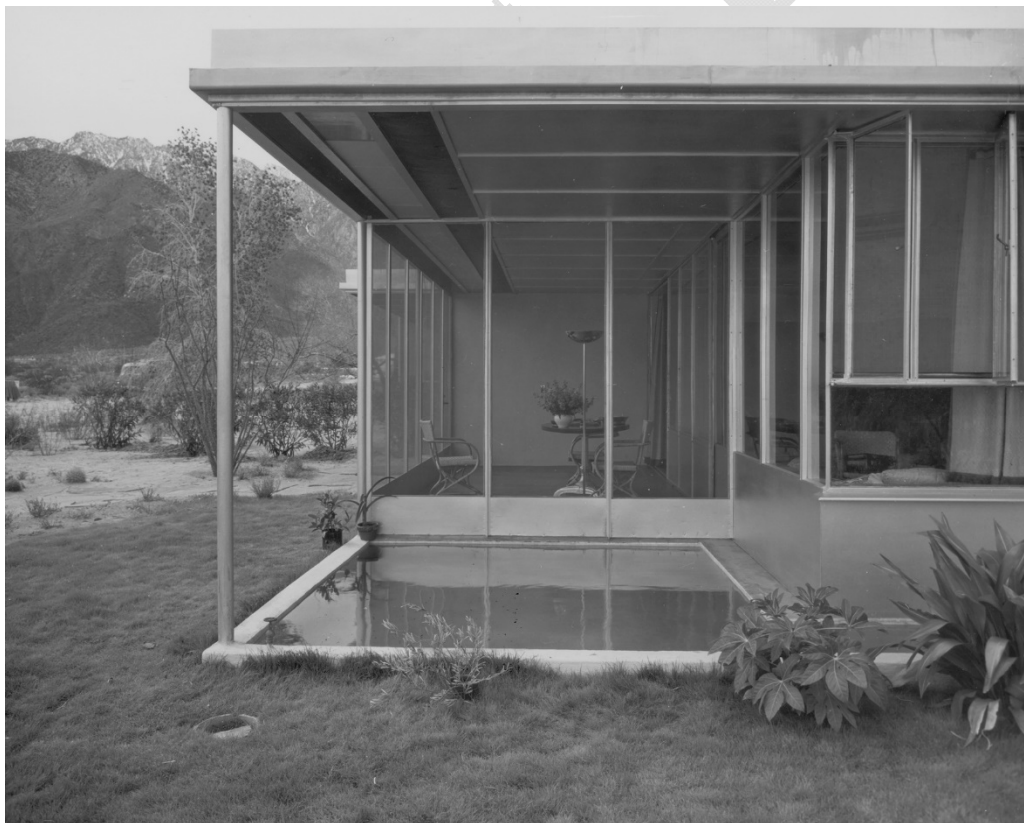
Grace Lewis Miller House (1937, Richard Neutra). Photographed by Julius Shulman. Source: Getty Research Institute.
