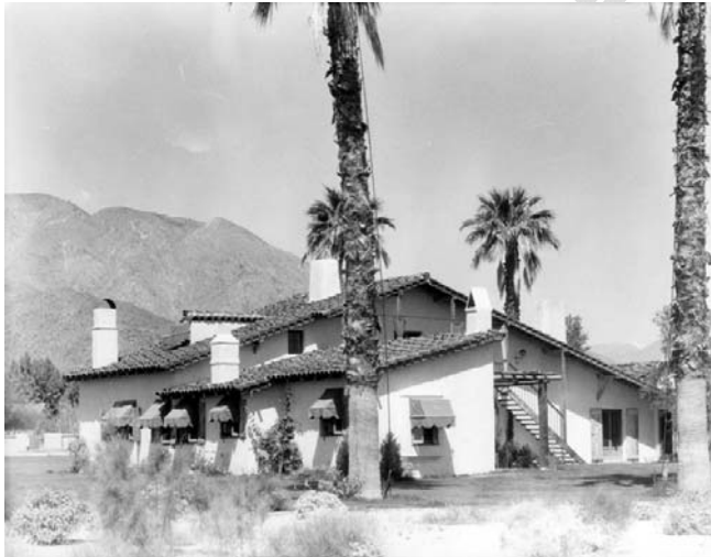
Designed in 1927 by architect John Byers, this was the longtime residence of Cary Grant, who purchased it in 1954. Source: Los Angeles Public Library.
