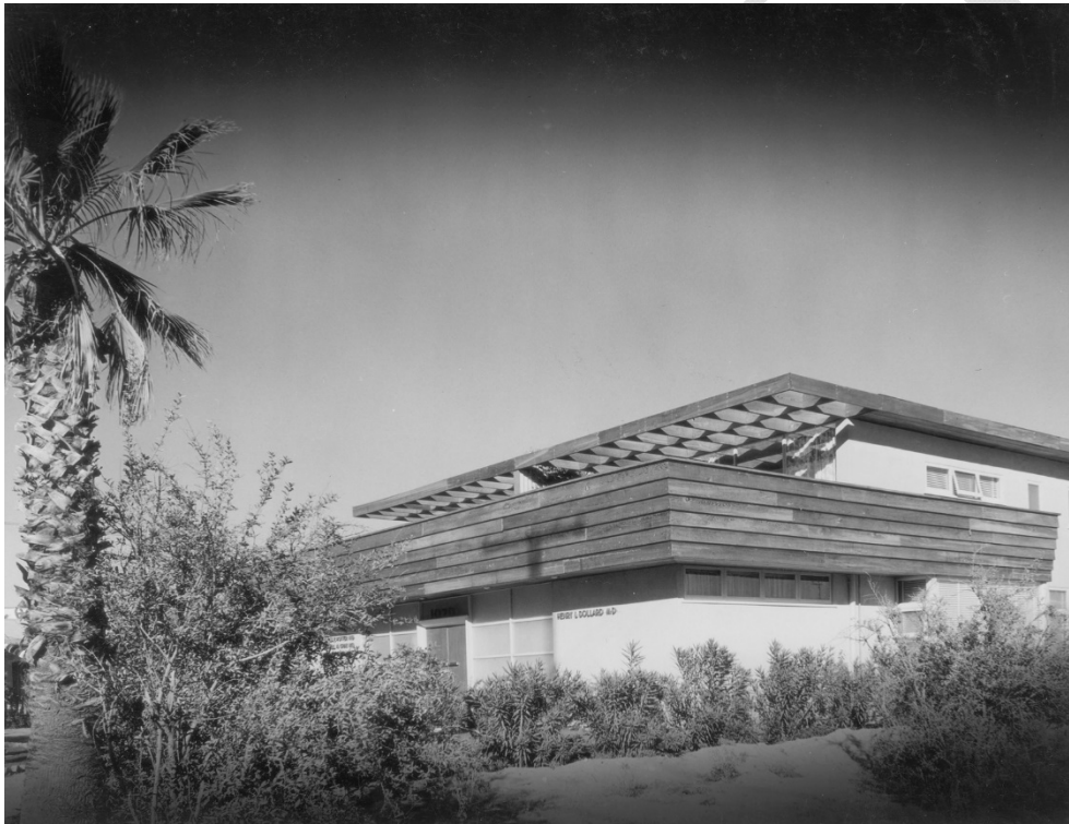
Potter Clinic (1947, Williams, Williams and Williams) located at 1020 N. Palm Canyon Drive. The combination retail and residential apartment building was, according to Julius Shulman, where architect E. Stewart Williams lived in 1949. Photograph: Julius Shulman. Source: Getty Research Institute.
