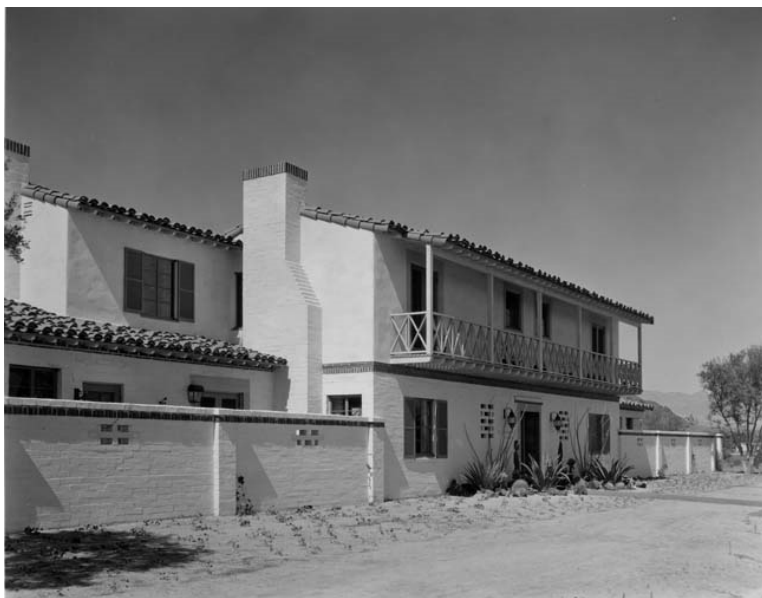
The two-story El Encanto Apartments (1928, Marshall P. Wilkinson) at 415 S. Palm Canyon Drive in an elegant Monterey Revival style. Source: Mott Collection, California State Library.
