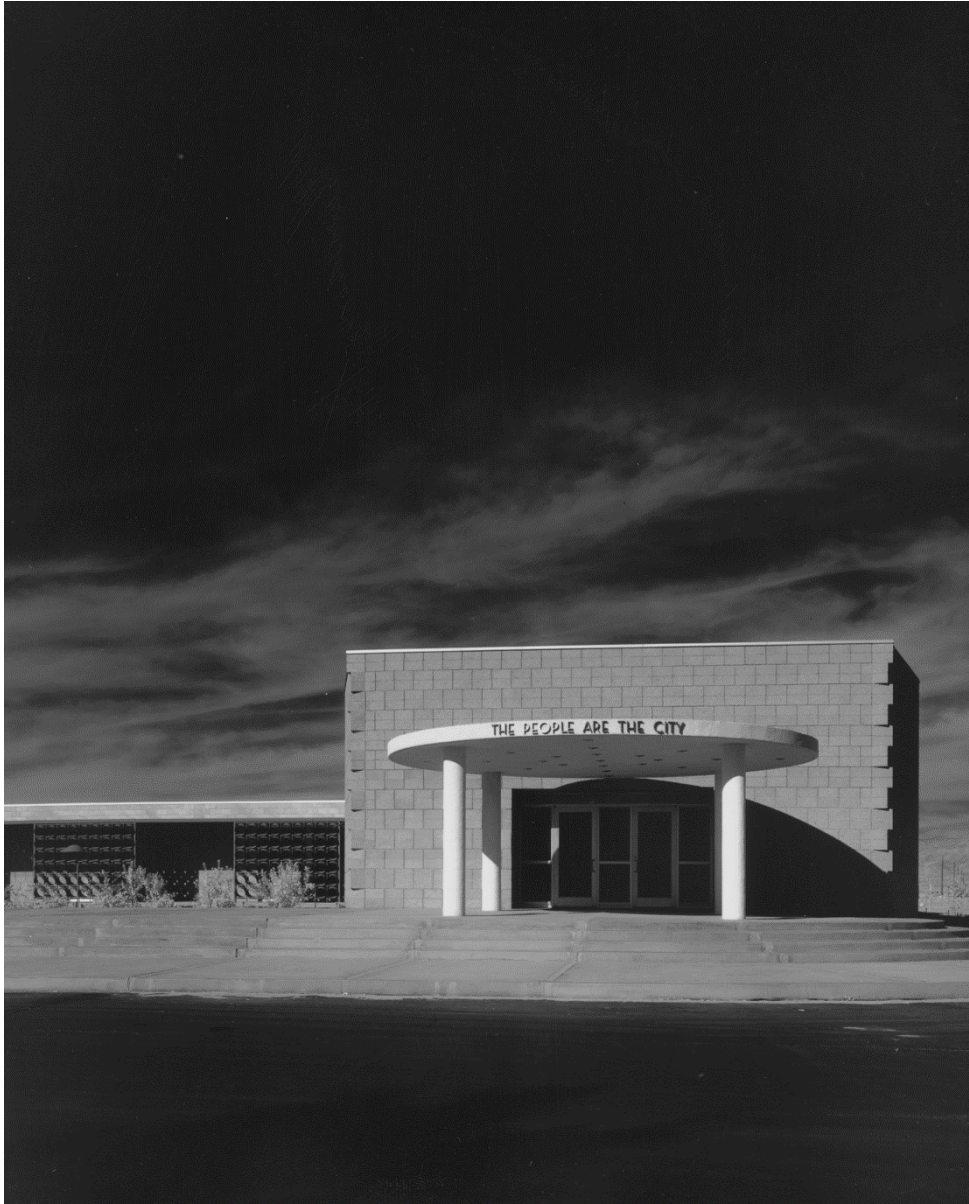
Palm Springs City Hall (1952, Clark, Frey & Chambers). Photographed by Julius Shulman, 1958. Source: Getty Research Institute.
