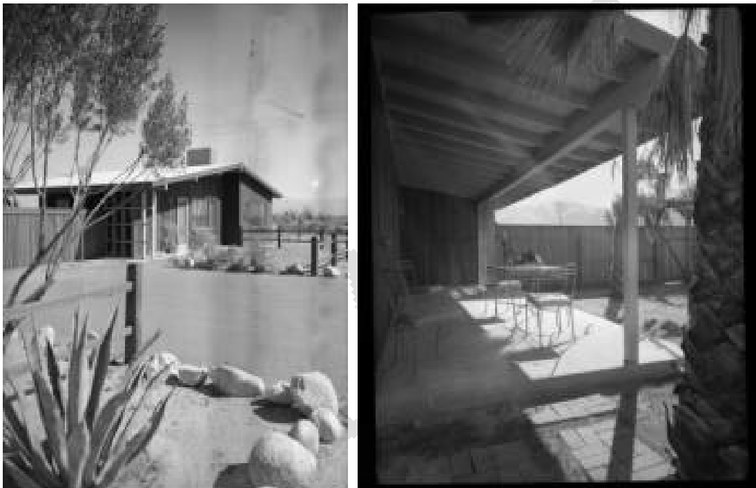
L: Exterior of one of the Tahquitz River Estates models by architect Allen G. Siple; Edward Huntsman Trout, landscape architect; interiors by Neblett & Williams. R: Rear porch of one of the Tahquitz River Estates models. Photographed by Maynard Parker c. 1950. Source: The Huntington Digital Library.
