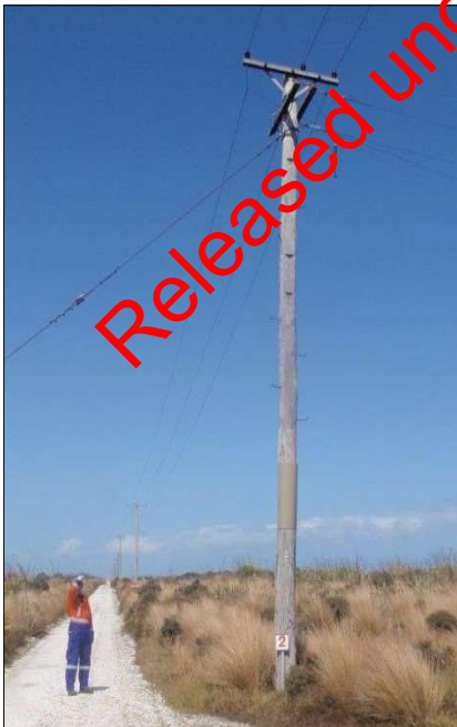
Figure 4: Fire potential from a burning possum dropping to the ground after scaling a power pole on the Peninsula
