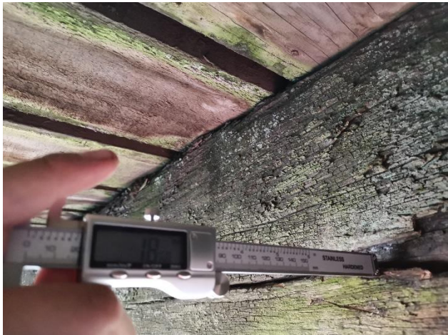
Figure 3 Timber Stringer No. 3 Defects
