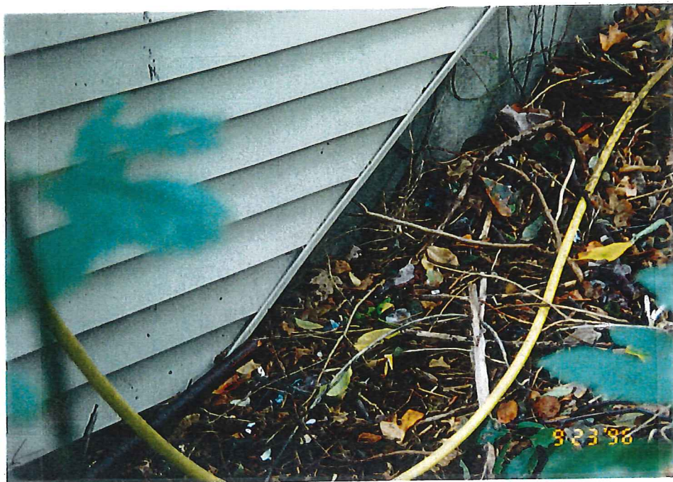
HIGH GRADE AT PRIMARY STAIR ENCLOSURE.
