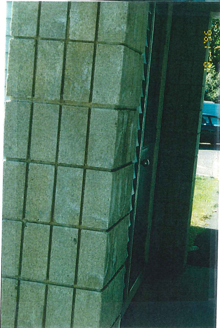
MINOR EFFLORESCENCE AT MASONRY PIERS.
