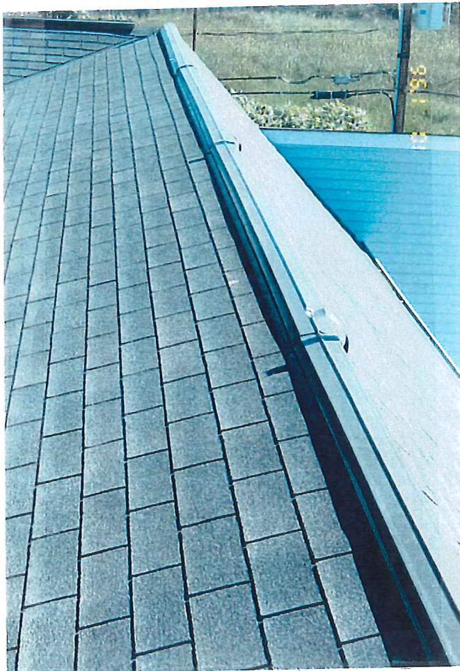
LOOSE JOINT COVERS AT ROOF RIDGE VENT.
