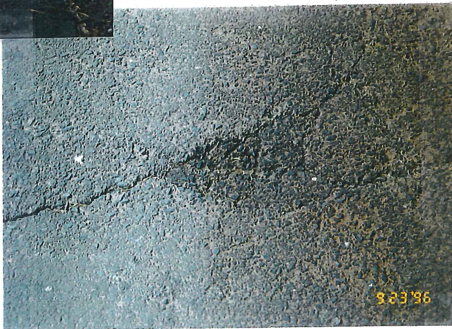
CRACKED PAVING.
