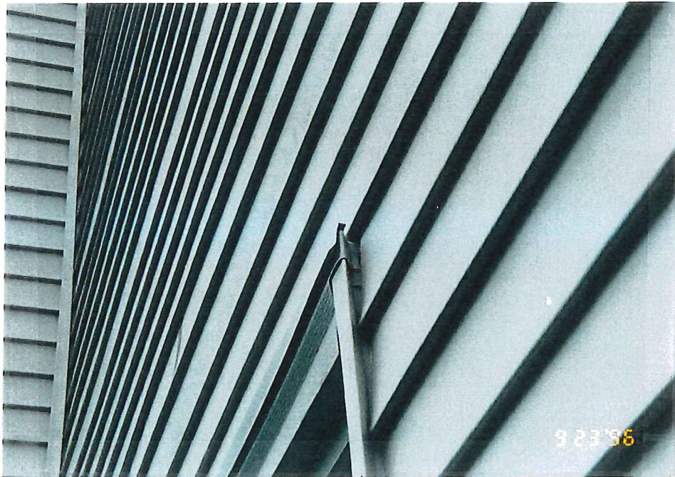
WINDOW HEAD FLASHINGS APPEAR TO BE PROPER.
