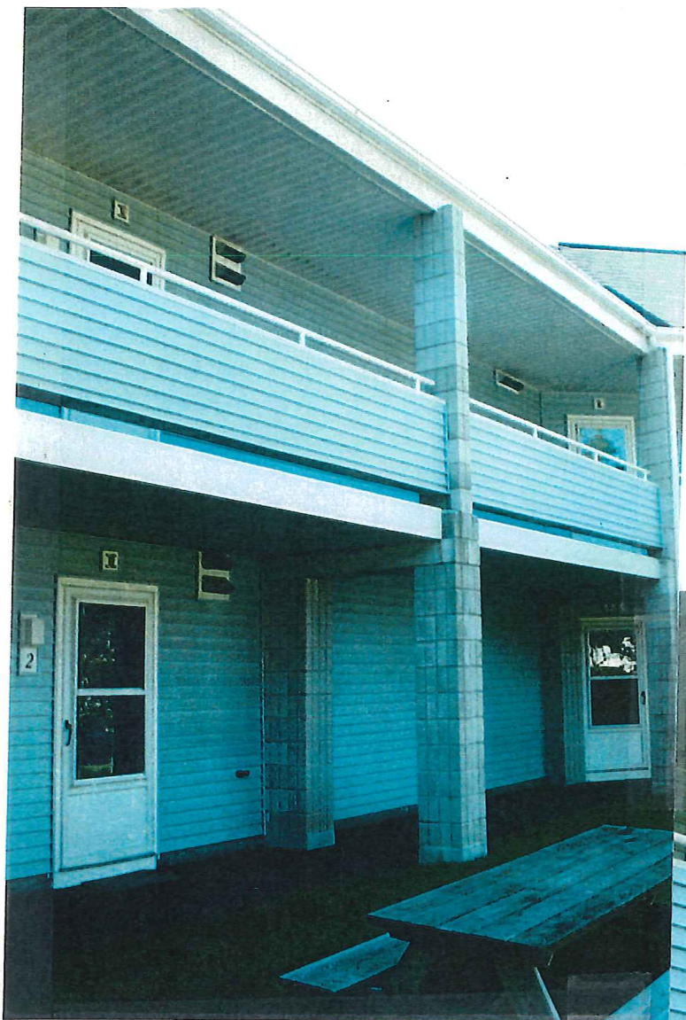
← MASONRY PIERS & BEAMS. THIS IS NOT PART OF A FIRE WALL & IS NOT
