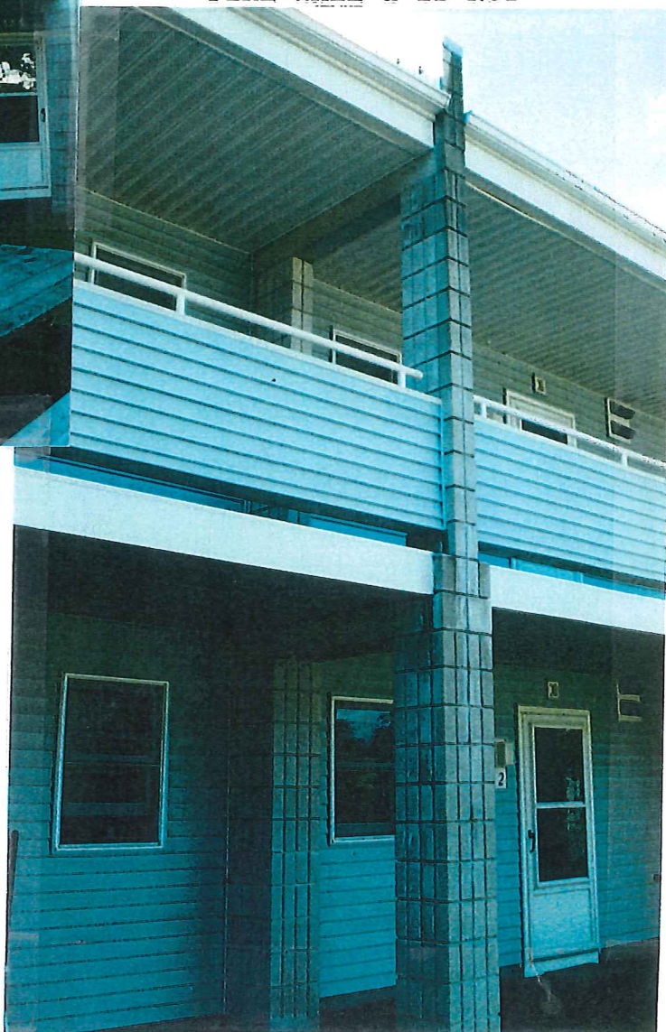
← MASONRY PIERS & BEAMS. THIS IS NOT PART OF A FIRE WALL & IS NOT
