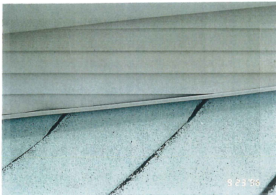
JOINT AT CHANGE IN ROOF HEIGHT.
