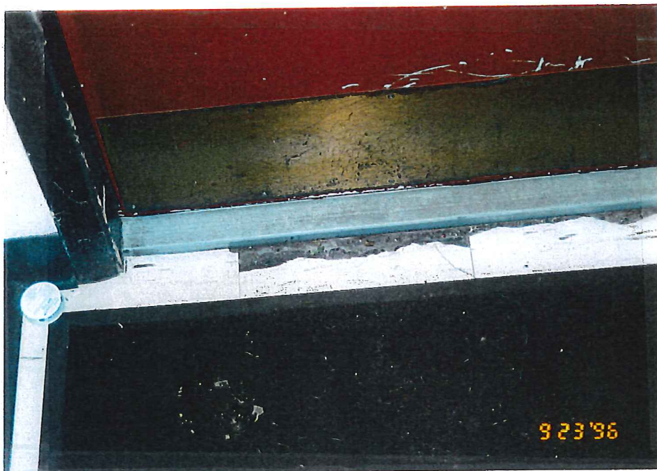
CHIPPED RESILIENT FLOORING IN PRIMARY STAIR ENCLOSURE.
