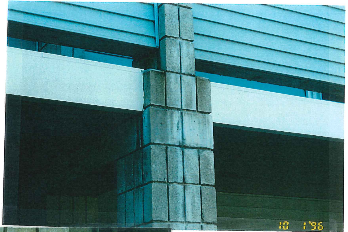
MINOR EFFLORESCENCE AT MASONRY PIERS.
