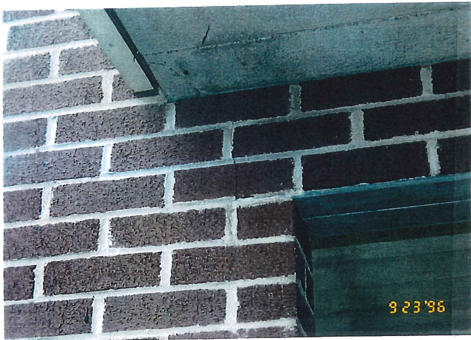
CRACK IN BRICK UNDER SECOND FLOOR WALKWAY, AT END OF STEEL LINTEL.
