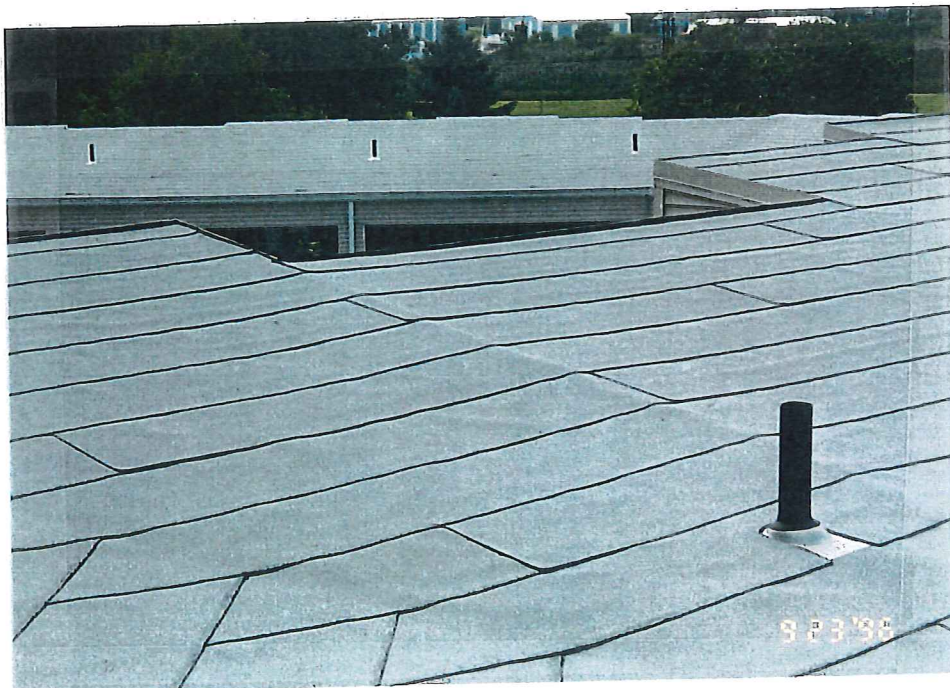
PUCKERED SURFACE OF ROOFING.
