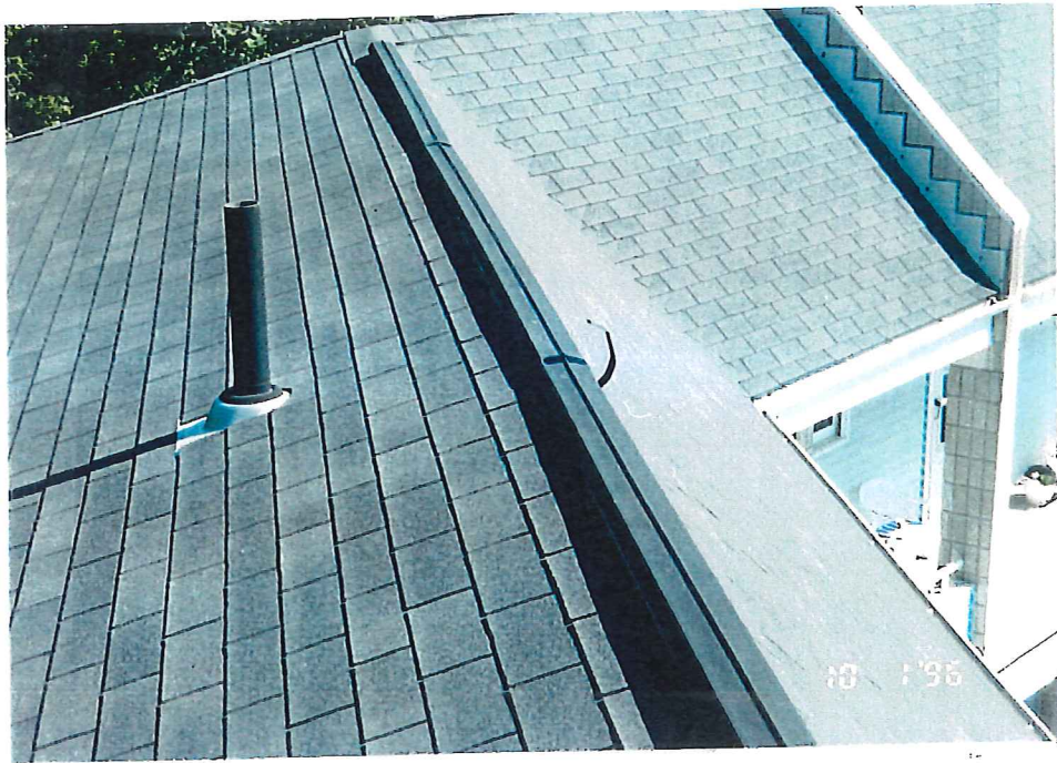
LOOSE JOINT COVERS AT ROOF RIDGE VENT.
