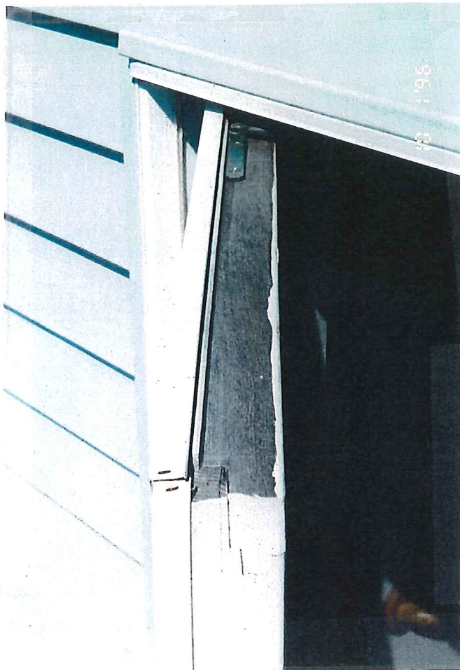
MOISTURE CONTENT 25% AT LOOSE CORNER TRIM.
