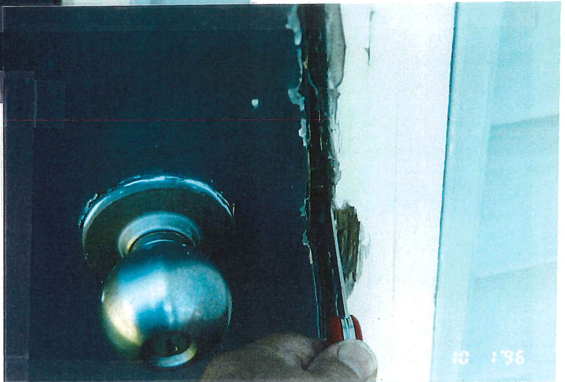
DOOR LOCK EASILY "LOIDED" WITH KNIFE.
