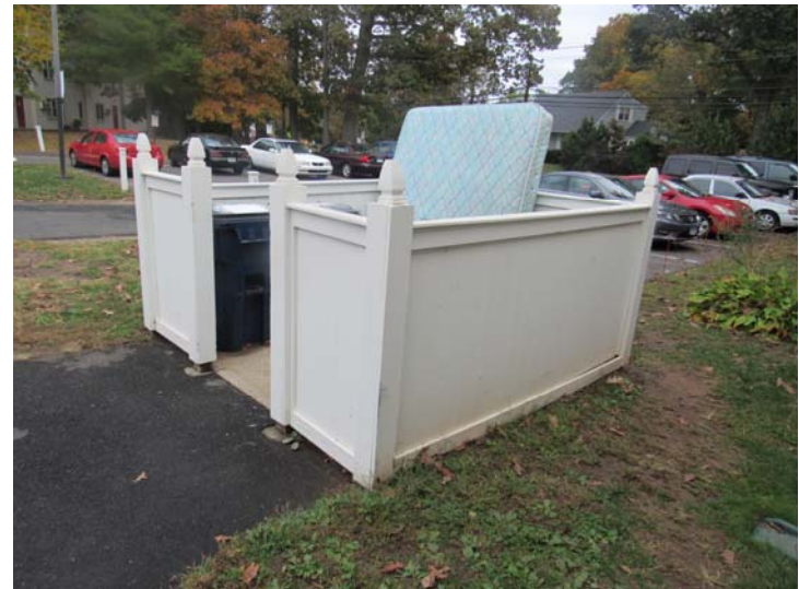
View of dumpster enclosure conditions – 1 of 4 serving development
