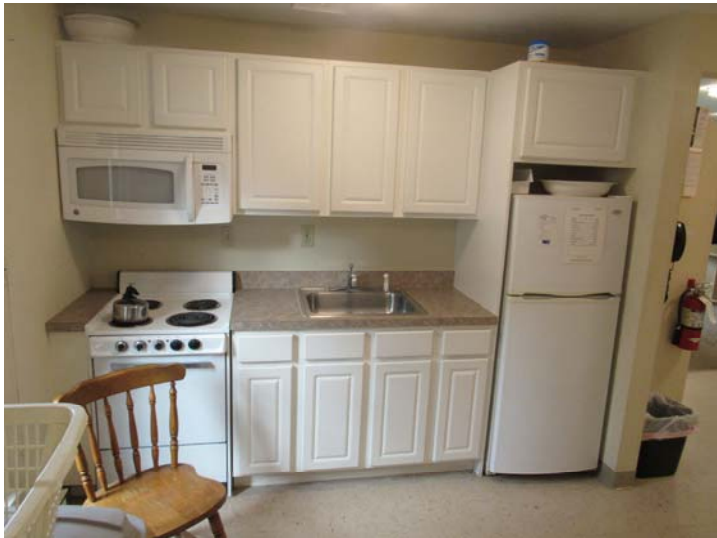
View of community kitchen finishes and equipment
