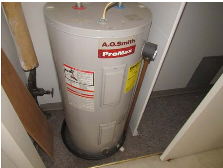
View of unit-level electric domestic water heater – varying ages and models
