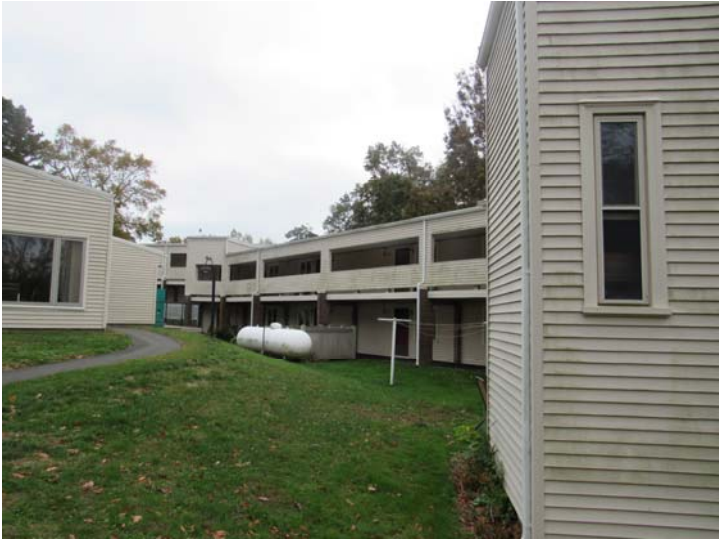
View of typical residential building architecture as seen at balcony/patio facade
