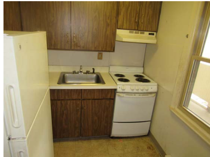
View of unit kitchen finishes and equipment – note original cabinet set
