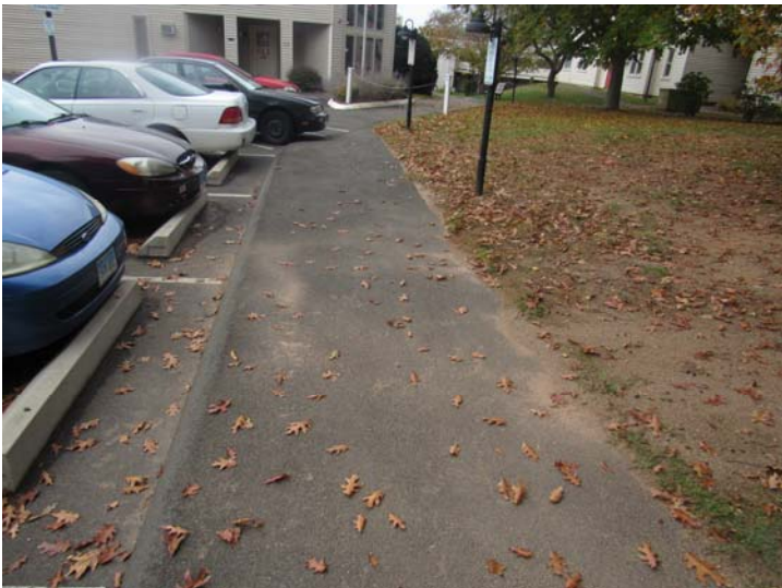
View of sample of asphalt walkway conditions – good overall conditions
