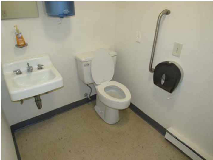
View of one of two common restrooms and fixtures
