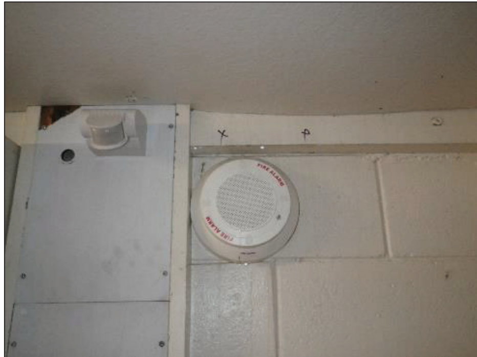
Water leaks from corridor roof drip onto alarm services, ceiling linings swollen and sagging.
