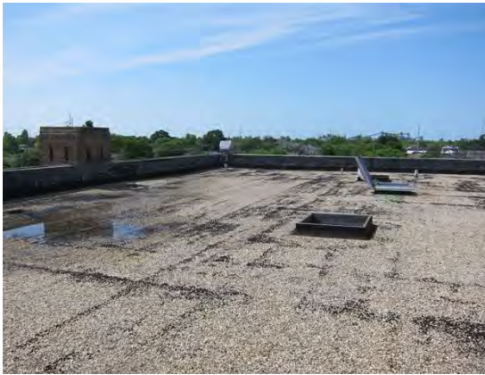
A201 Roof Looking South
