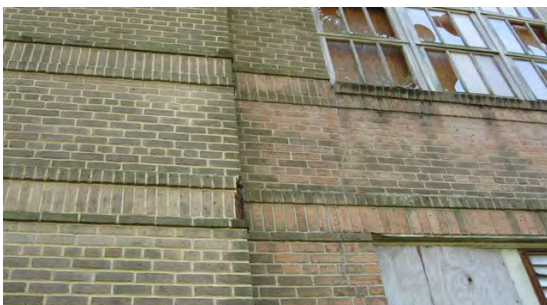
A23 Exterior Joint at Addition
