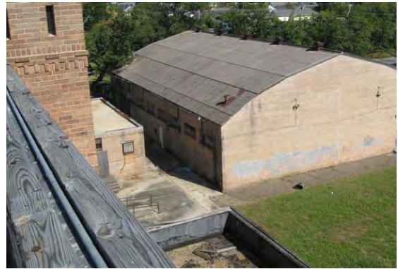
A41 Gym from Roof of Main Building
