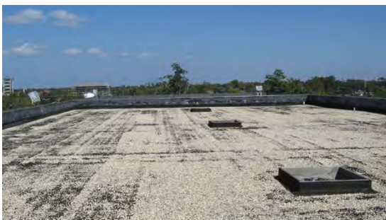
A209 Roof at Main Building
