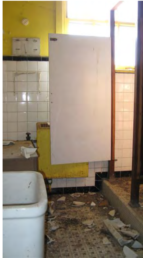
A143 Toilet Room Second Floor
