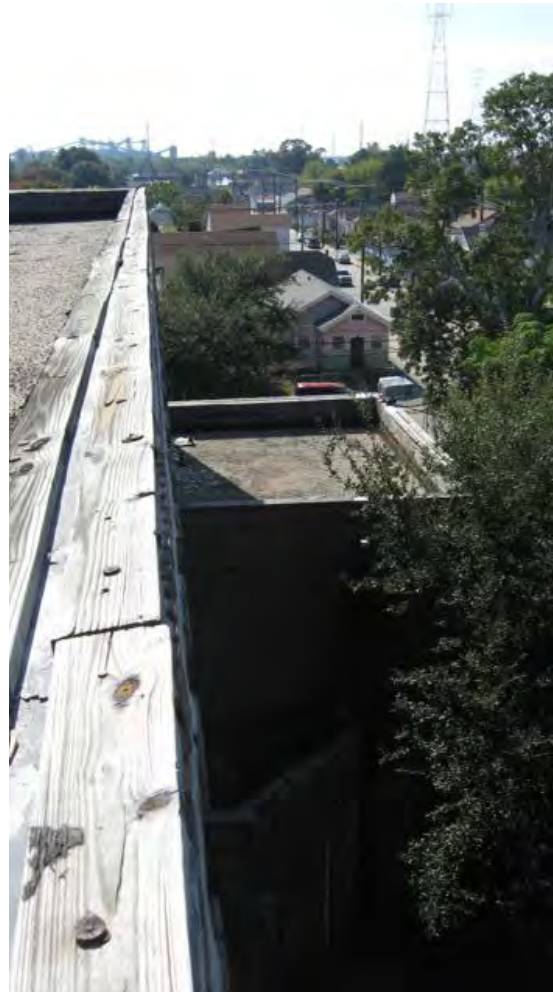
A206 Main Entry and Southwest Wing from Roof
