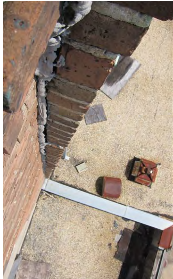
A52 Joint at Addition Looking Down from Roof
