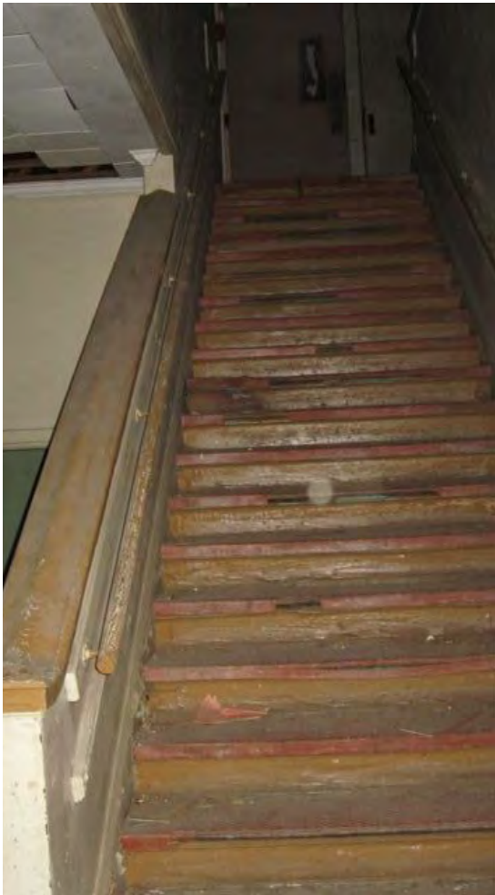
A112 Existing Stair at Main Entry
