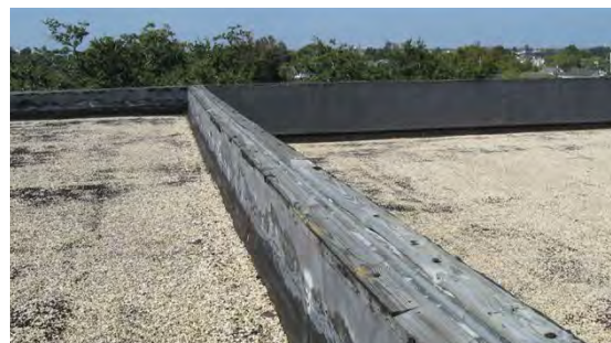
A208 Parapet Condition at Joint Between Addition and Original Building
