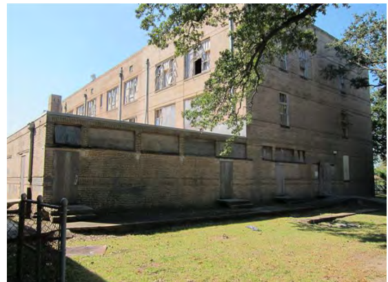
A55 Northeast Corner
