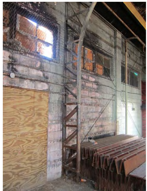
A305 Steel Framing at Gym
