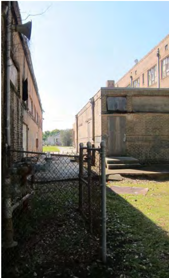
A53 Area Between Gym and Main Building Facing Southwest
