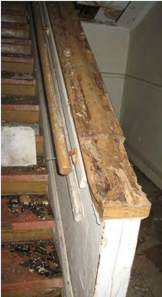
A126 South Stair at Second Floor
