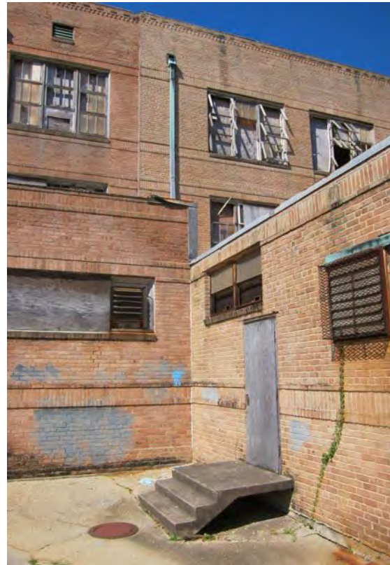
A35 Southeast Façade at Addition
