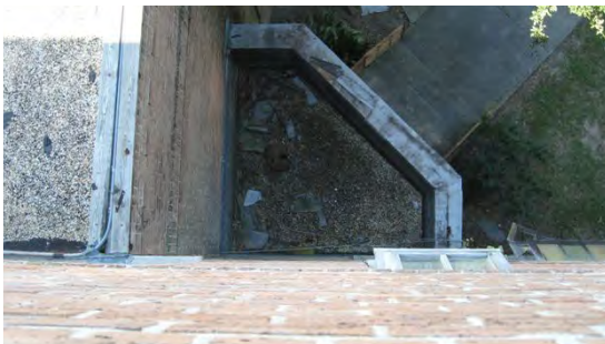
A207 Main Entry Roof from Above
