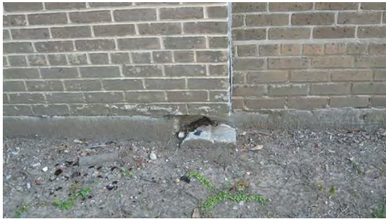
A5 Joint at Addition on Northwest Side-Ledge
