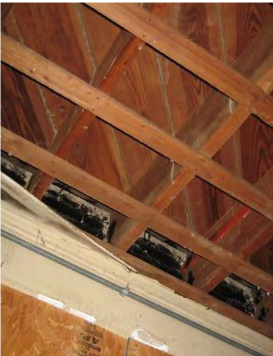
A133 Typical Wood Floor Framing
