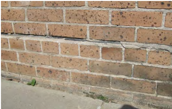
A38 Watertable Course in Masonry at Main Building
