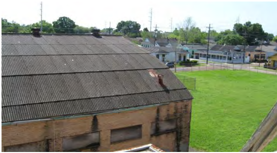
A33 Gym Roof
