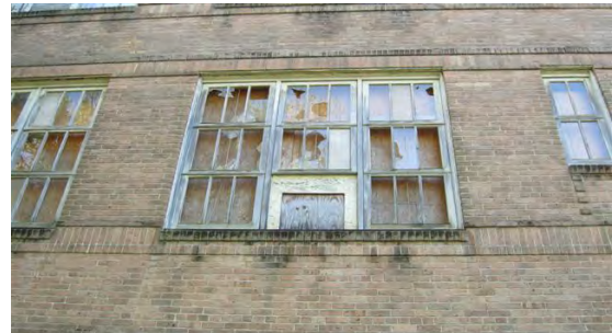
A25 Exterior- Typical Wood Window
