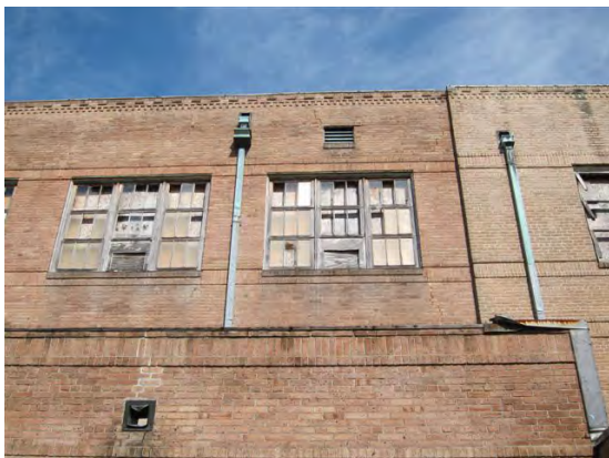
A31 Wood Windows and Copper Downspouts- Leaderheads
