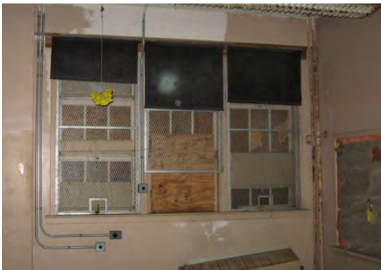
A105 Typical Window Condition
