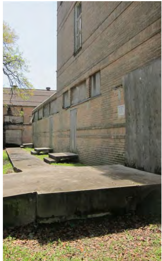
A49 Paving at Northeast Side
