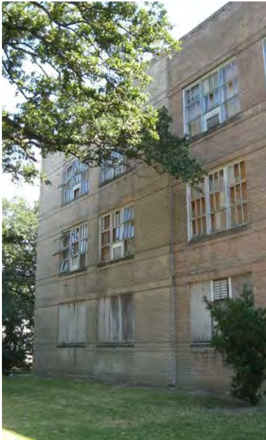
A8 Northwest Façade at Addition
