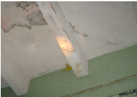
A109 Sprayed Finish at Concrete Addition
