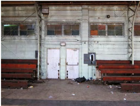
A301 Gym Interior Facing Northwest
