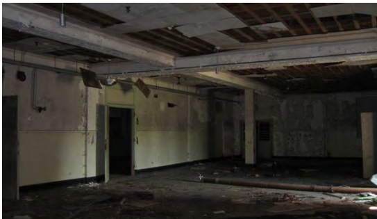
A120 Transfer Beam Under Loadbearing Corridor Wall at Floors Above
