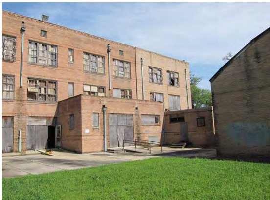
A50 Southeast Façade
