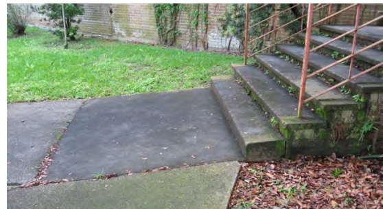
A26 Paving at Main Entry
