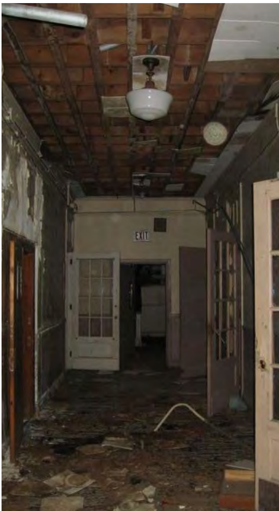
A125 Second Floor Corridor Facing South
