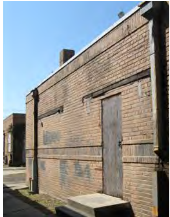
A43 Southeast Façade at Addition
