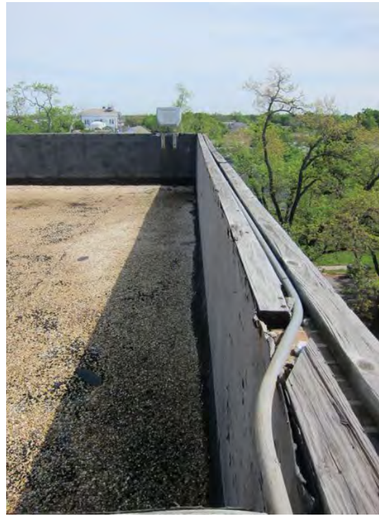
A202 Parapet at Addition Looking Northeast
