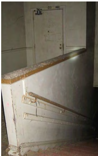
A130 South Stair to Main Entry
