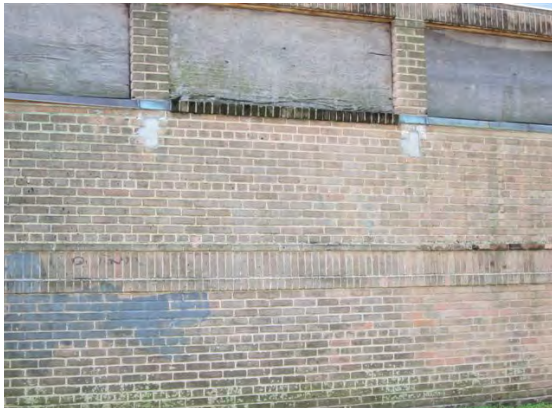
A48 Exterior- Northwest Side
