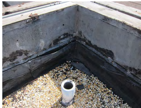
A204 Existing Gravel-Ballasted Low Slope Roof
