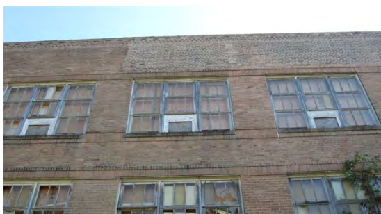
A11 Rebuilt Brick Parapet at Northwest Side
