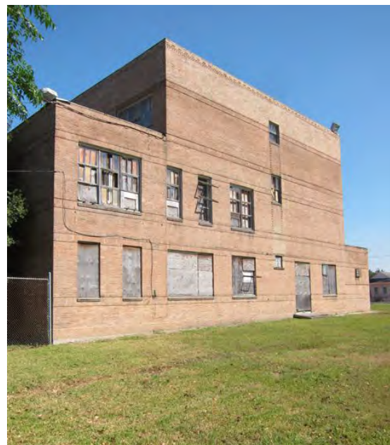
A15 Southwest Façade
