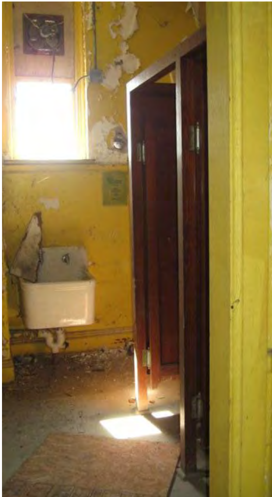
A128 Second Floor Toilet Room
