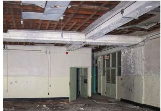
A104 Cafeteria Facing Southwest
