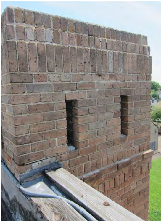
A205 Masonry at Boiler Stack
