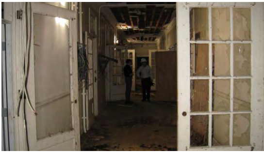
A140 Third Floor Corridor Facing North
