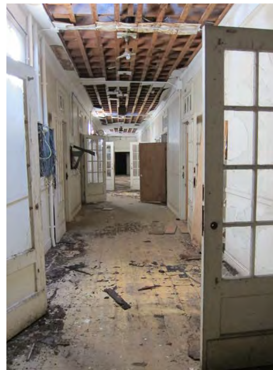
A139 Third Floor Corridor Facing South
