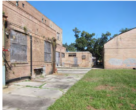
A37 Area Between Gym and Main Building Facing Northeast
