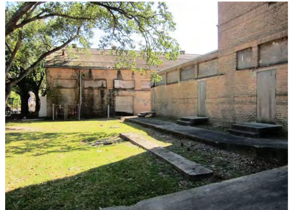
A54 Northeast Corner Facing Gym
