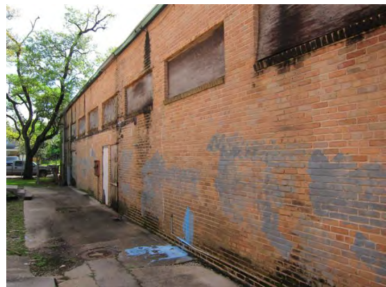
A32 Northwest Façade of Gym
