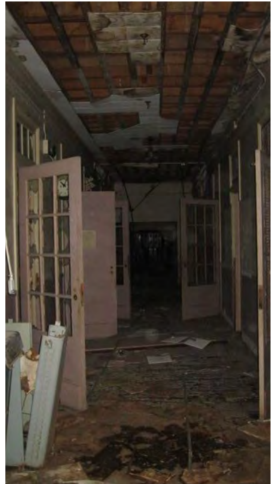
A124 Second Floor Corridor Facing North
