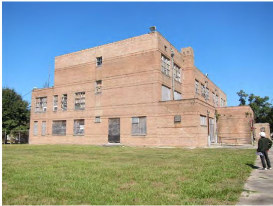
A16 Southwest Façade
