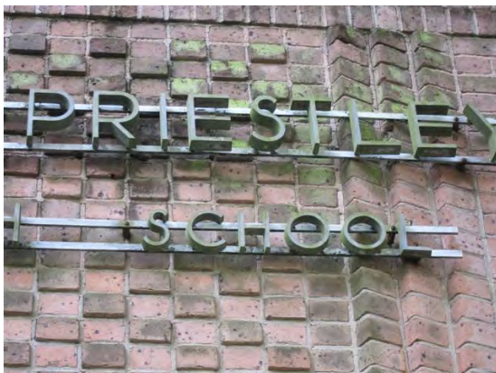
A20 Patterned Brick and Building Sign above Main Entry
