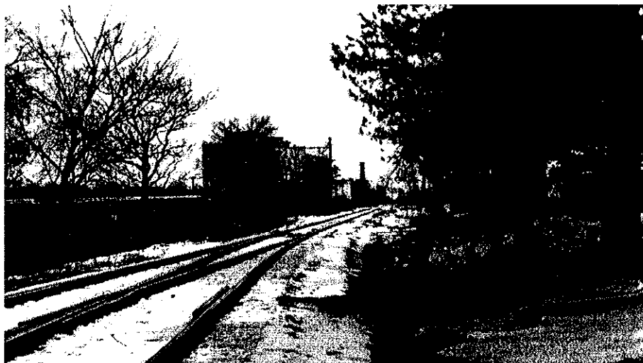
Photo 3. Picture of the railroad line running southward from downtown and separating the South Elm Street site from the adjacent St. James neighborhood.
