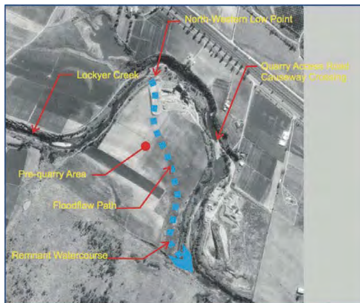
Figure 5.15: Image of u-shaped bend before the quarry pit was excavated Source: Exhibit 144, Dr John Macintosh, Expert Hydrology Report – 10 January 2011 Flood – Circumstances and Contributing Factors , 11 August 2015 [p96: Figure 10.6(a)].
