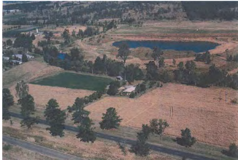
Figure A11: 2000 Oblique aerial photo provided by Ms Mallon Source: Statement by Charmaine Mallon, 1 July 2015 [ ]; Exhibit 131, Mr David Starr, Grantham quarry – geotechnical investigations and expert opinion on formation of earthworks , Revised 28 August 2015 [p37 Plate 27a]
