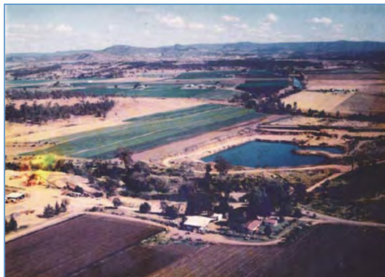
Figure A6: 1985 oblique aerial photo provided by Ms Gearing Source: Exhibit 131, Mr David Starr, Grantham quarry – geotechnical investigations and expert opinion on formation of earthworks , Revised 28 August 2015 [p35: Plate 25]
