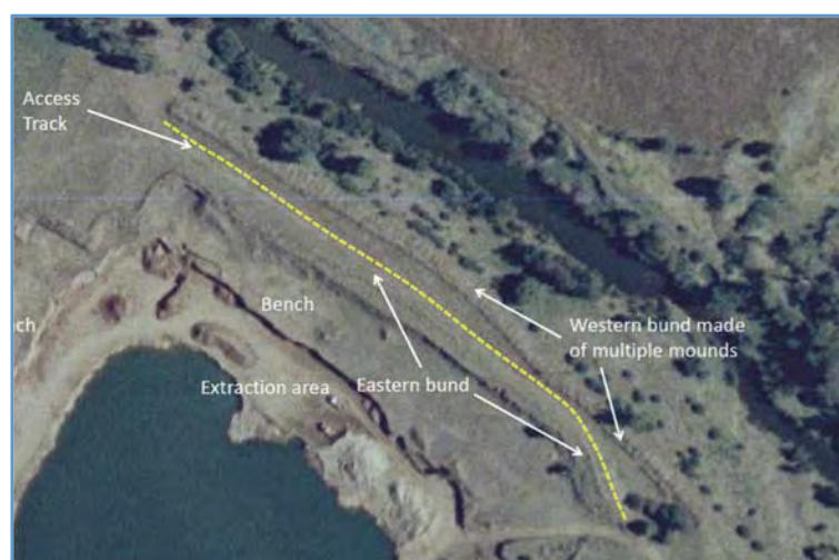
Figure A12: 2001 aerial photo provided by the DNRM (annotations by David Starr). Source: Exhibit 131, Mr David Starr, Grantham quarry – geotechnical investigations and expert opinion on formation of earthworks , Revised 28 August 2015 [p43: Plate 32b]
