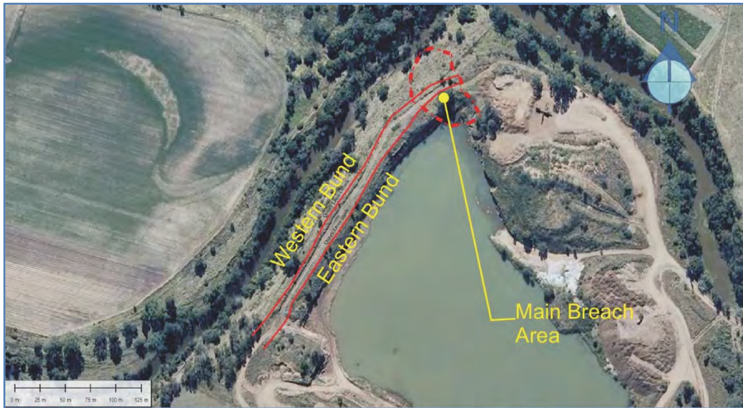
Figure 4.3: Image showing location of pre-flood bunds and the location of the main breach Source: Exhibit 144, Dr John Macintosh, Expert Hydrology Report – 10 January 2011 Flood – Circumstances and Contributing Factors , 11 August 2015 [p70: Figure 8.15] (amended).
