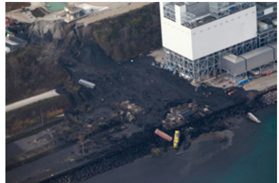
Photograph of Oak Creek coal ash bluff collapse. Mark Hoffman/Milwaukee Journal Sentinel.
