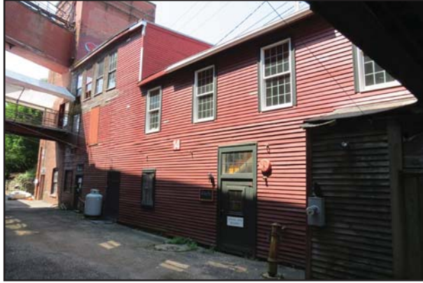
Building 14: Drafting Room and Storehouse Construction Date: 1858-64
