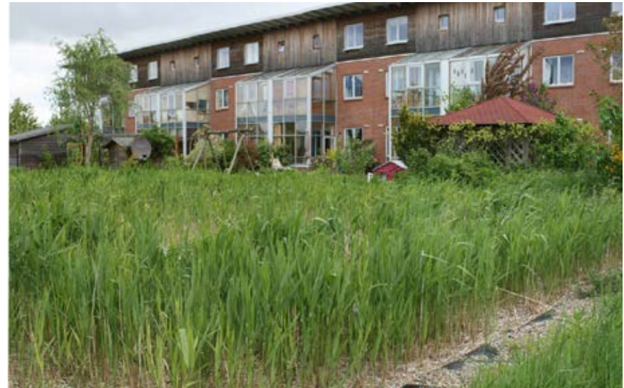
ABOVE: Constructed wetlands are artificial wetlands that not only help retain and infiltrate wastewater or stormwater, but can also treat pollutants in the water before it returns to the groundwater or freshwater supply.
