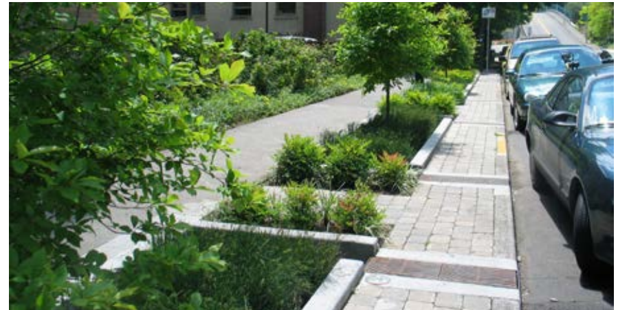
ABOVE: Streetside stormwater collection planter boxes (CarbonTalks CA).
