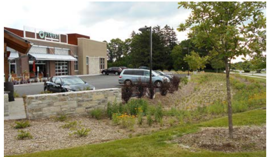
ABOVE: Vegetated rain gardens and bioswales help filter and treat stormwater runoff from large impervious surfaces (i.e. parking lots).
