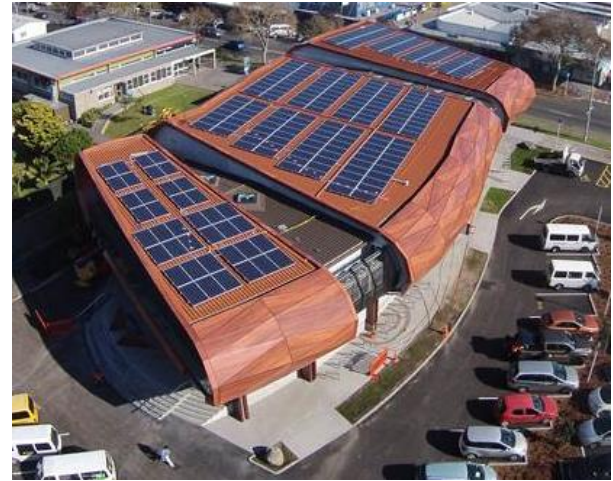
The 68kW solar PV array on Te Oro, Glen Innes' new music and arts centre.
