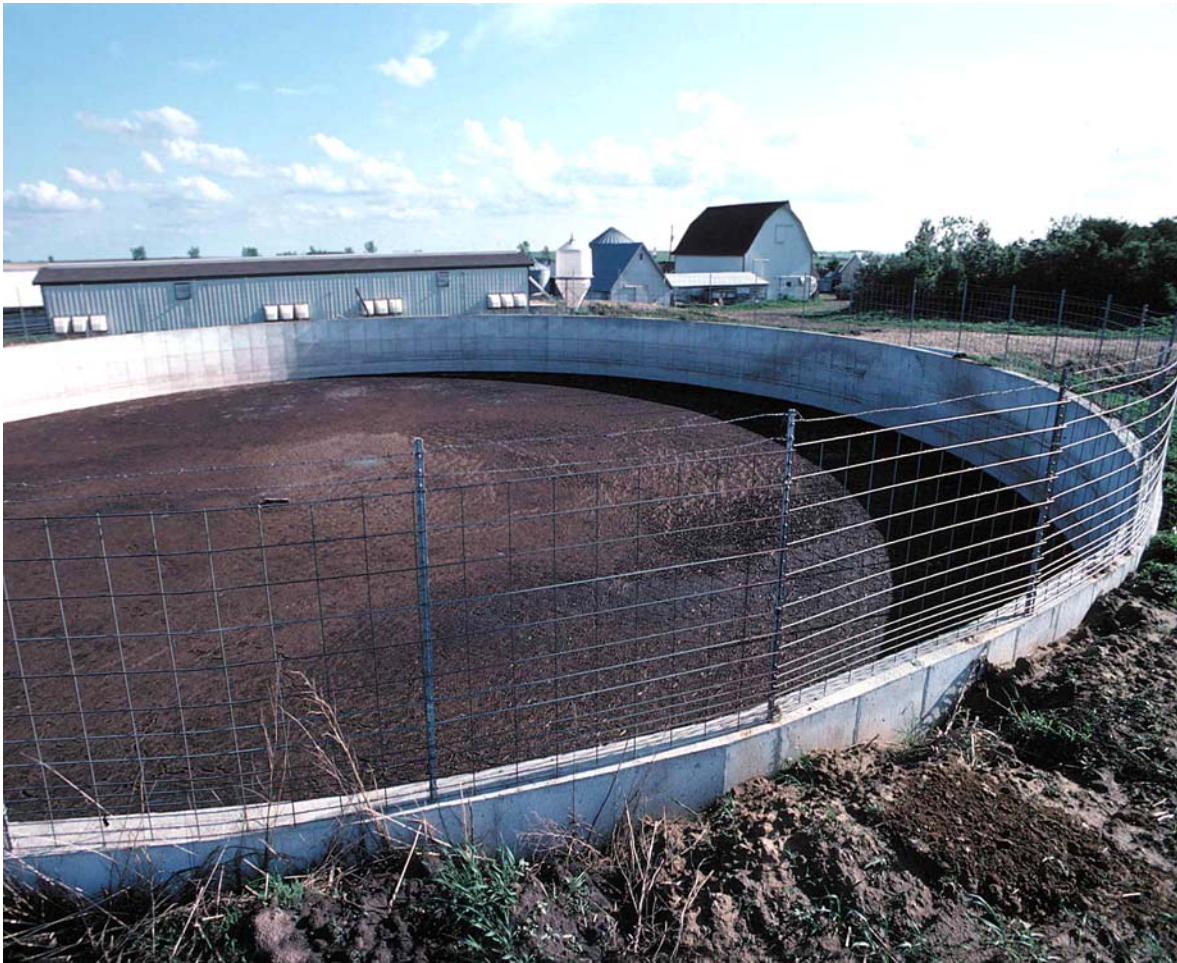
Figure 5.4. Concrete manure storage tank. Structures of this type will prevent leakage of waste into groundwater.
