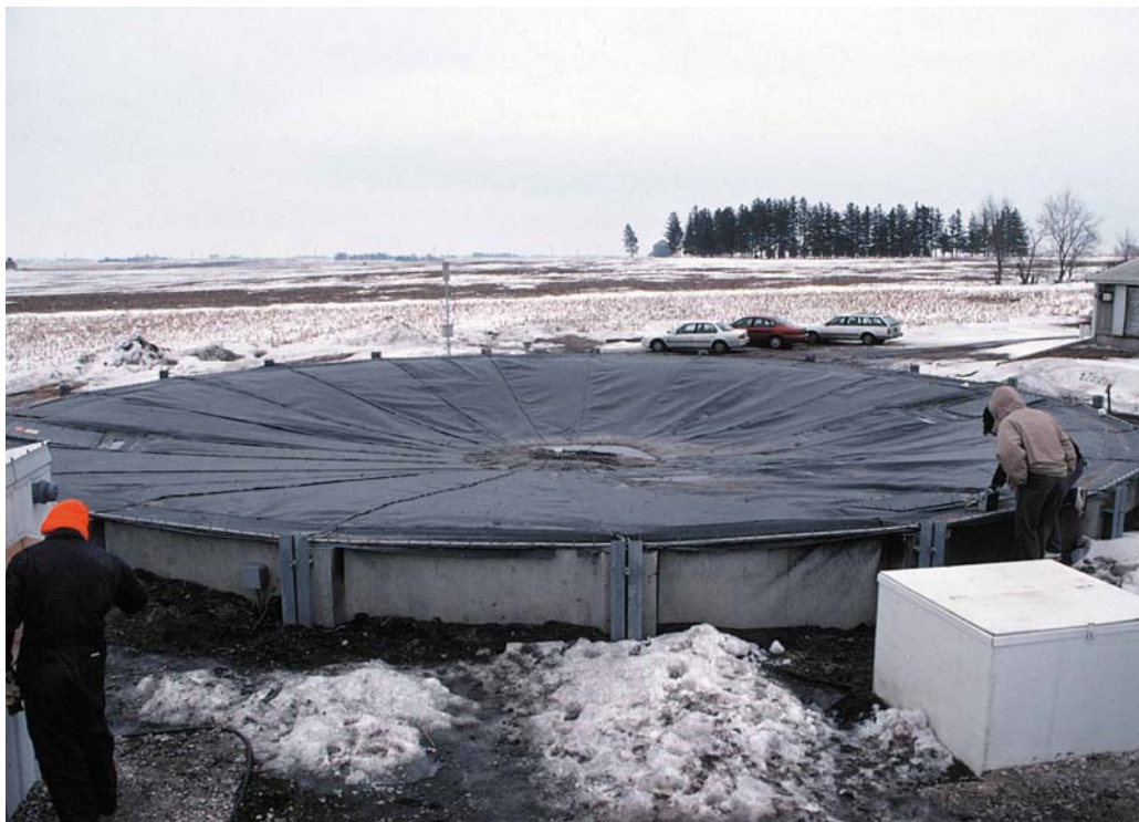
Figure 7.6. Covered manure tank generating methane in Iowa.
