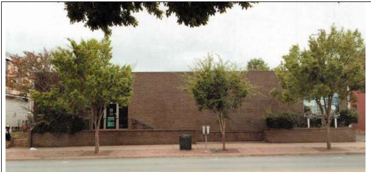
The American Legion Building Existing North Façade 2015
