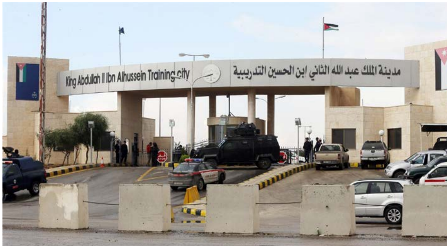
25 Entrance to the International Police Training 26 Center in Amman, Jordan
