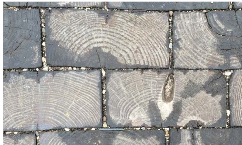
Permeable Pavers on Hessler Court
