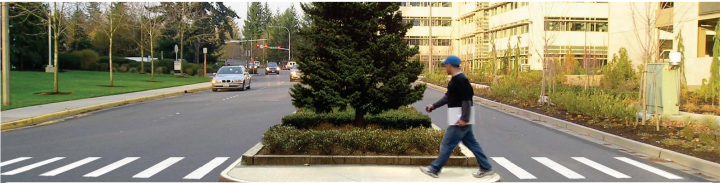
Refuge islands give crossing pedestrians a safe space to wait without having to make it across the entire intersection at once.
