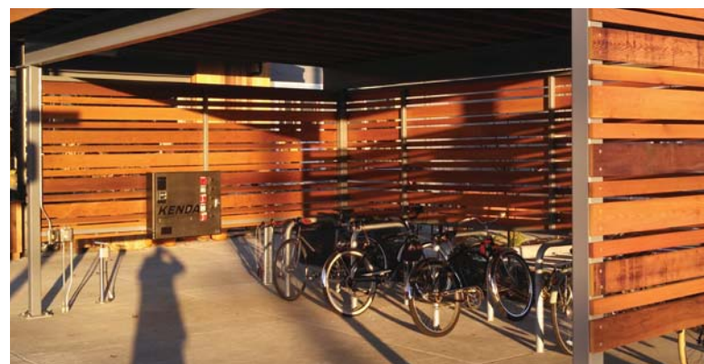
Covered Bicycle Parking with bicycle repair station and inner tube vending machine
