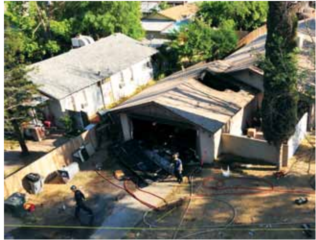
Aerial view of structure from AD corner
