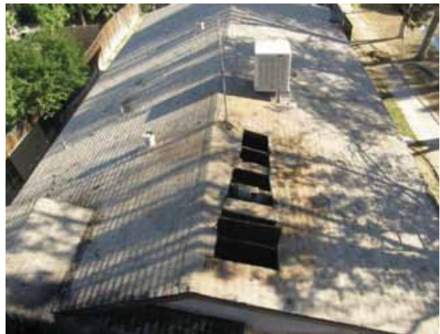
Location of ventilation holes
