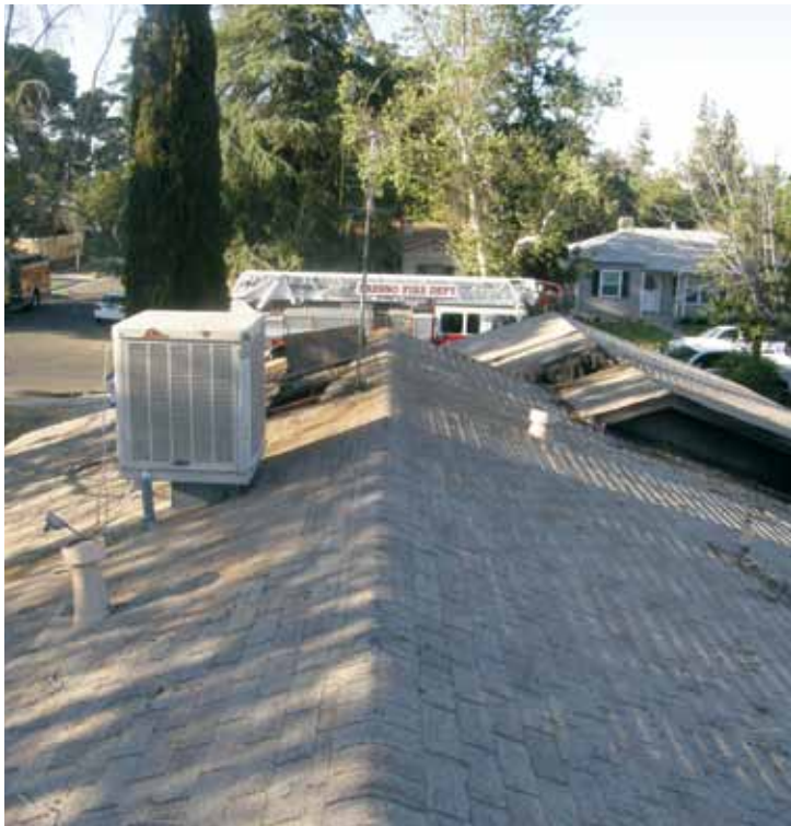
View of roof from the south
