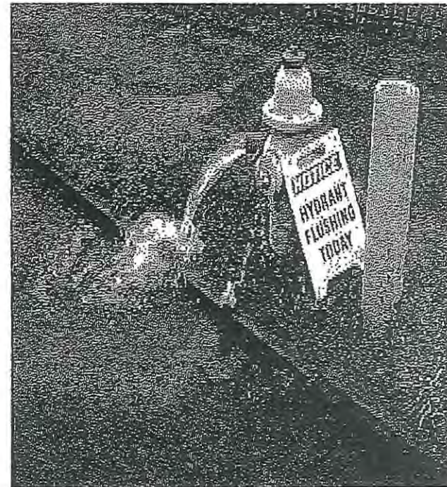
Flushing out discolored water
