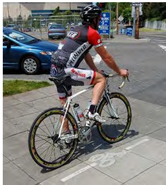
Figures 115 and 116: Signage and pavement markings direct bicyclists to use the pavement detection loop to activate a traffic signal.
