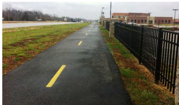
Figure 92: This sidepath incorporates a yellow striped centerline to separate bi-directional traffic.
