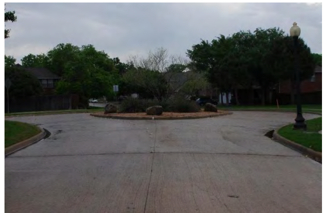
Figure 53: The traffic circle on Waterview Dr slows motor vehicle traffic, creating a safe and calm environment for pedestrians.
