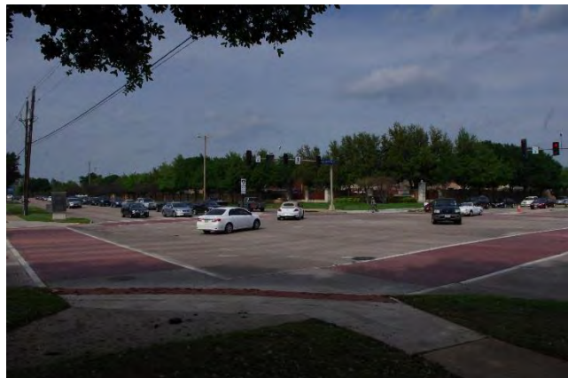
Figure 15: Parkway Blvd and Denton Tap Rd, the City's busiest intersection for pedestrians, includes designated crosswalks across each leg of the intersection.
