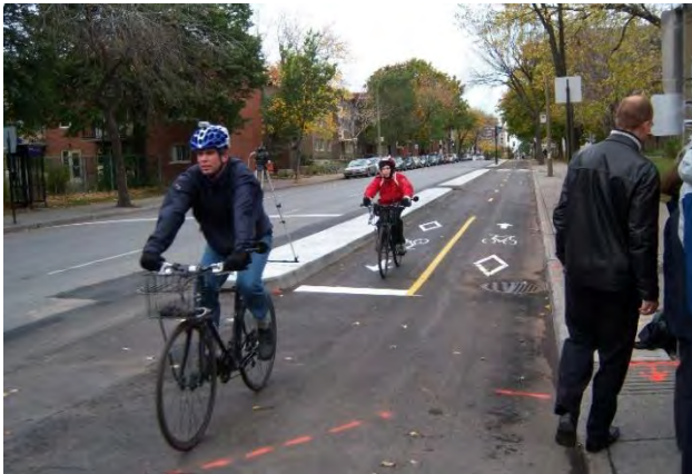
Figure 88: This two-way cycle track is separated from motor vehicle travel lanes by a raised concrete barrier.
