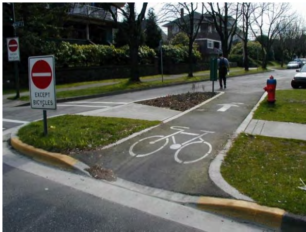
Figures 96 and 97: Traffic diverters allow through bicycle traffic while dispersing motor vehicle traffic onto adjacent roadways.
