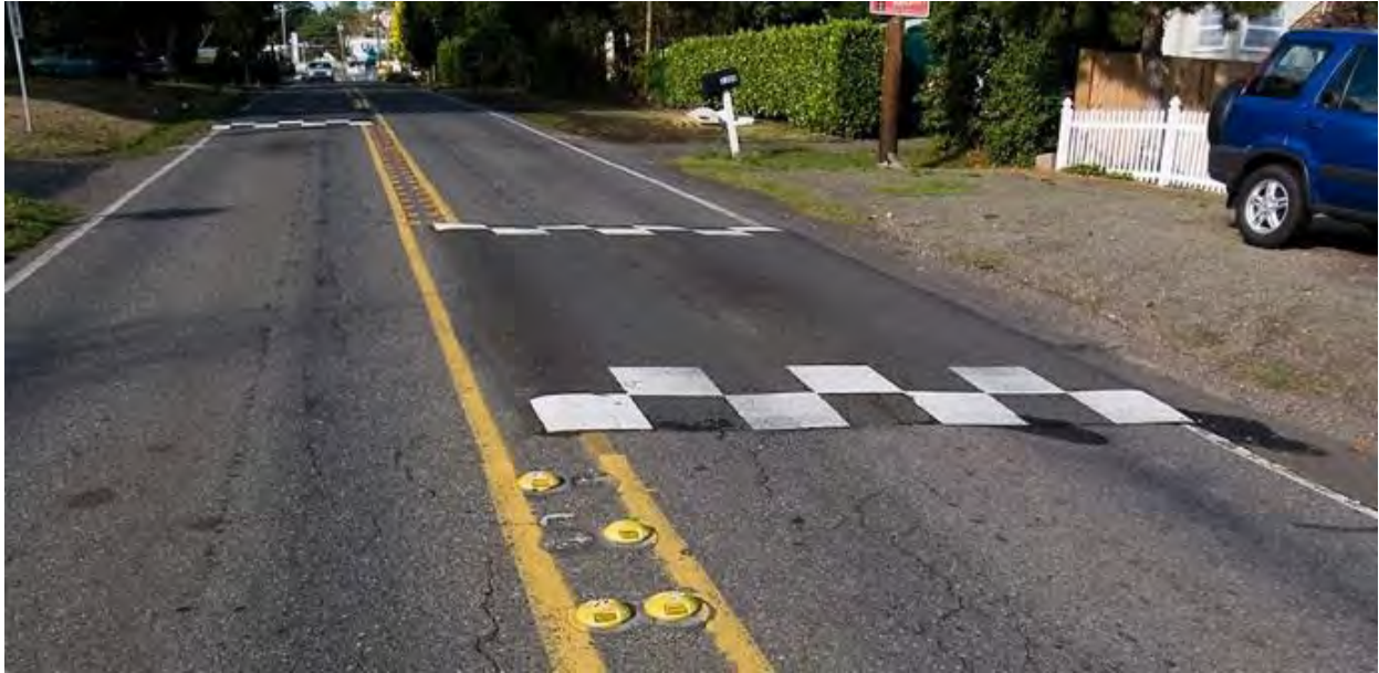
Figure 95: A speed table can effectively reduce motor vehicle speeds, increasing bicycle and pedestrian safety.
