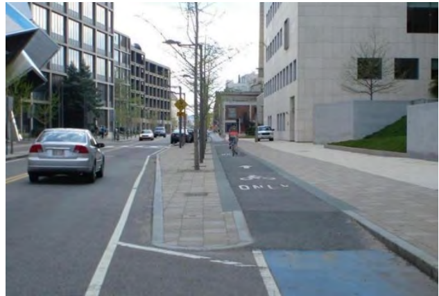
Figure 87: A raised cycle track in Cambridge, Massachusetts.
