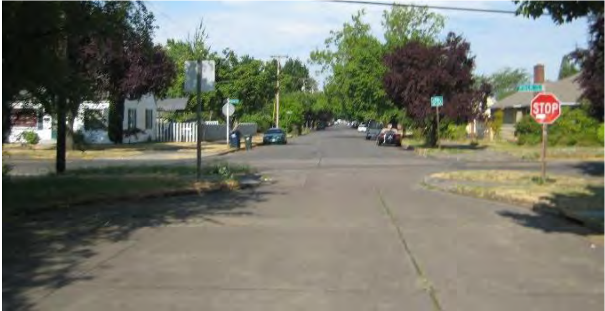
Figure 98: A neckdown reduces the street width at an intersection, decreasing pedestrian crossing widths, limiting turning radii, and slowing down motor vehicle speeds.
