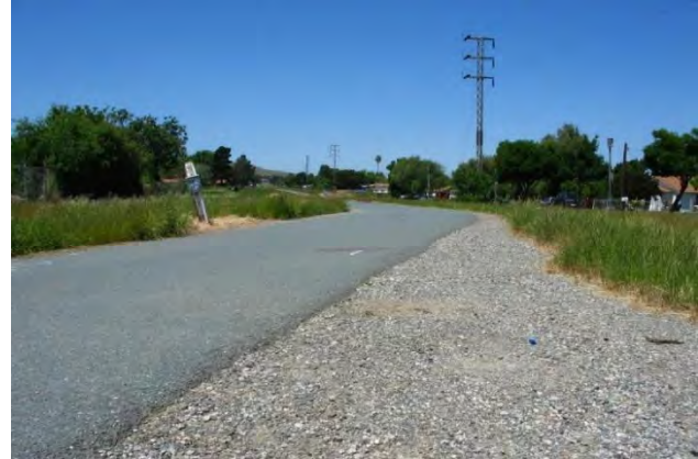
Figure 124: Decomposed granite or crushed limestone can provide an excellent shoulder to meet clearance requirements and provide a desirable surface for walkers and runners.
