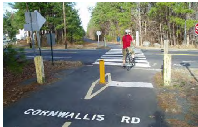
Figure 131: At unsignalized trail crossings, high-visibility crosswalk markings increase motorist awareness of crossing pedestrians.
