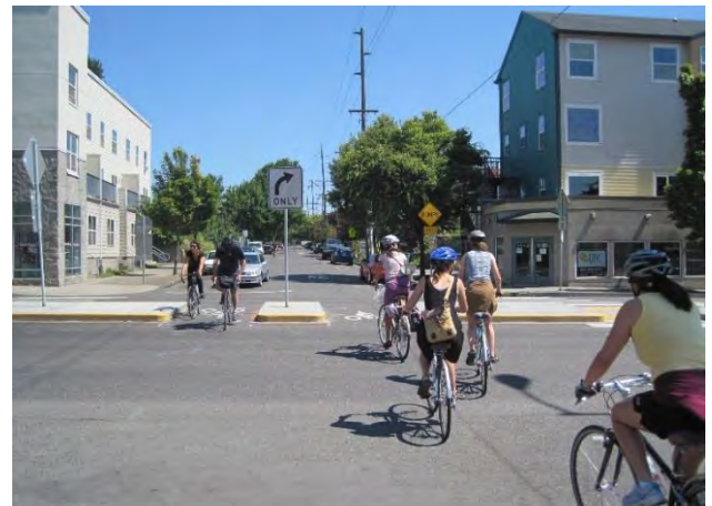
Figure 80: Traffic diverters allow through bicycle movements while restricting motor vehicle traffic.
