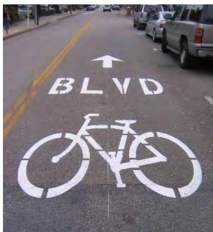
Figures 75 and 76: A combination of pavement markings and distinct signs distinguish bicycle boulevards from other shared travel lanes.
