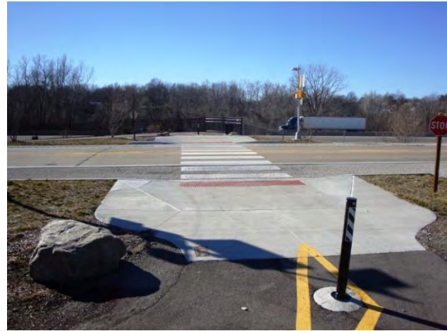
Figure 130: Bollards, ADA compliant curb ramps, high-visibility crosswalk markings, and rectangular rapid flashing beacons help improve user safety at this street crossing.
