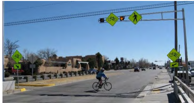
Figures 133 and 134: Full signals (left) and hybrid signals (right) can be used at trail crossings.
