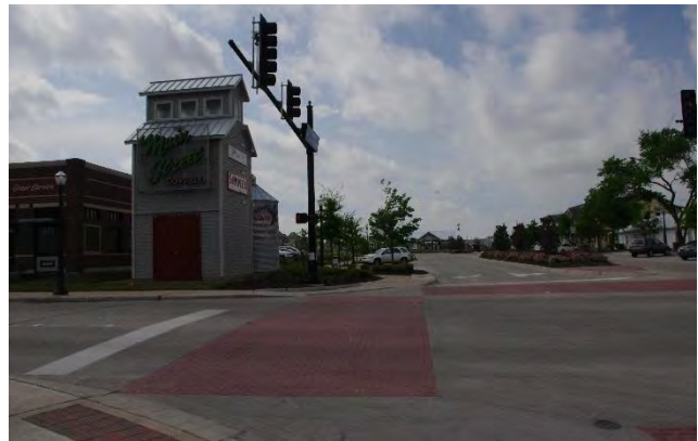
Figure 51: Push button-activated countdown timers, textured crosswalks, and ADA-accessible curb ramps enhance pedestrian safety at Bethel Rd and Coppell Rd.
