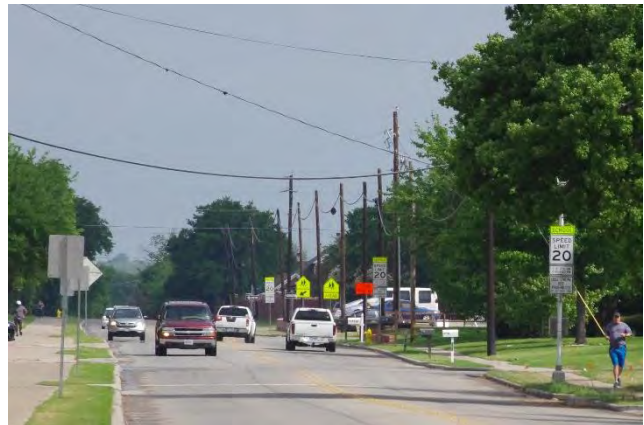
Figure 11: Collector roads like Coppell Road balance mobility and accessibility.
