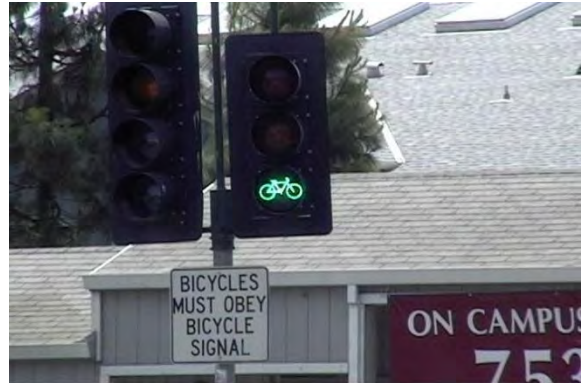
Figure 117: Bicycle signal heads can be used to allow bicyclists to clear the intersection before motor vehicles receive a green light.
