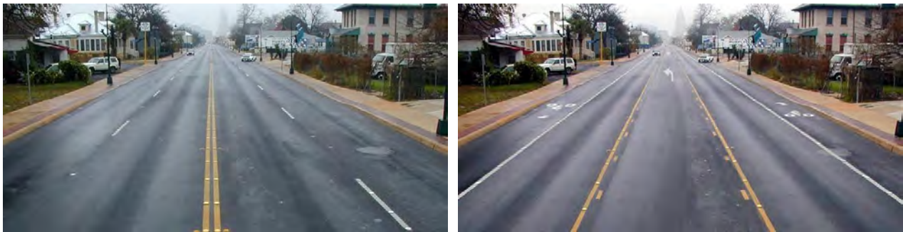
Figures 93 and 94: Before and after images from this road diet show how roadway space can be reallocated to increase space for bicyclists.
