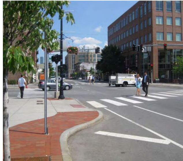
Figure 68: Bulb-outs increase motorists' visibility of pedestrians while also reducing turning speeds.
