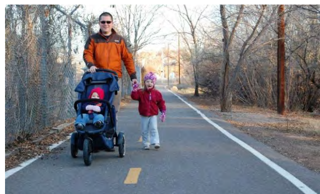
Figure 126: Some shared use paths incorporate both centerline and edge striping.
