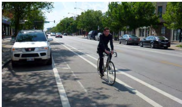
Figure 85: Buffer zones can be provided on both sides of the bike lane, increasing separation from both parked and traveling motor vehicles.
