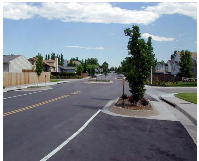
Figures 99 and 100: Chicanes slow motor vehicle traffic, creating a more calm and welcoming environment for both bicyclists and pedestrians.
