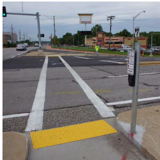
Figure 68: Bulb-outs increase motorists' visibility of pedestrians while also reducing turning speeds.
