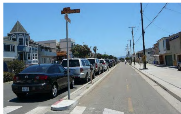
Figure 90: A raised concrete barrier and vehicle parking create adequate separation to provide cyclists with a comfortable facility.
