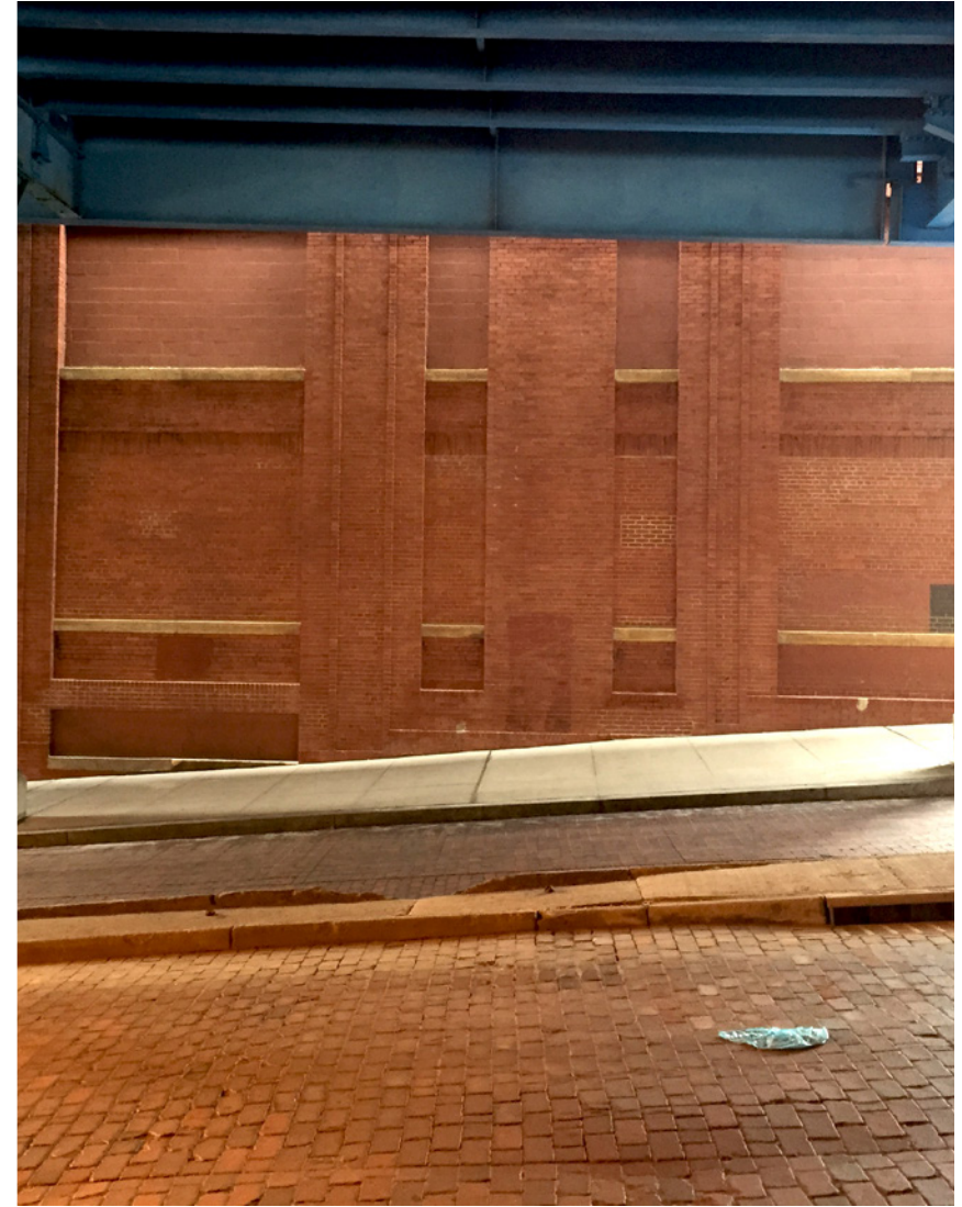
Great Building Stock (Big + Brick)
