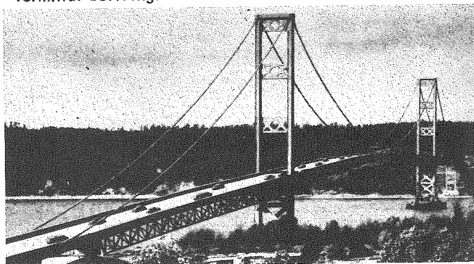
The new Tacoma Narrows Bridge across Puget Sound, connecting Tacoma with the Olympic Peninsula.
