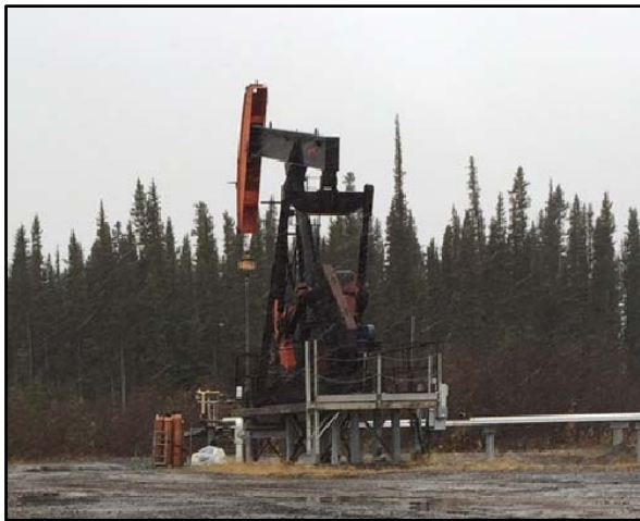
Norman Wells Operations Wellsite Equipped with a Pumpjack
