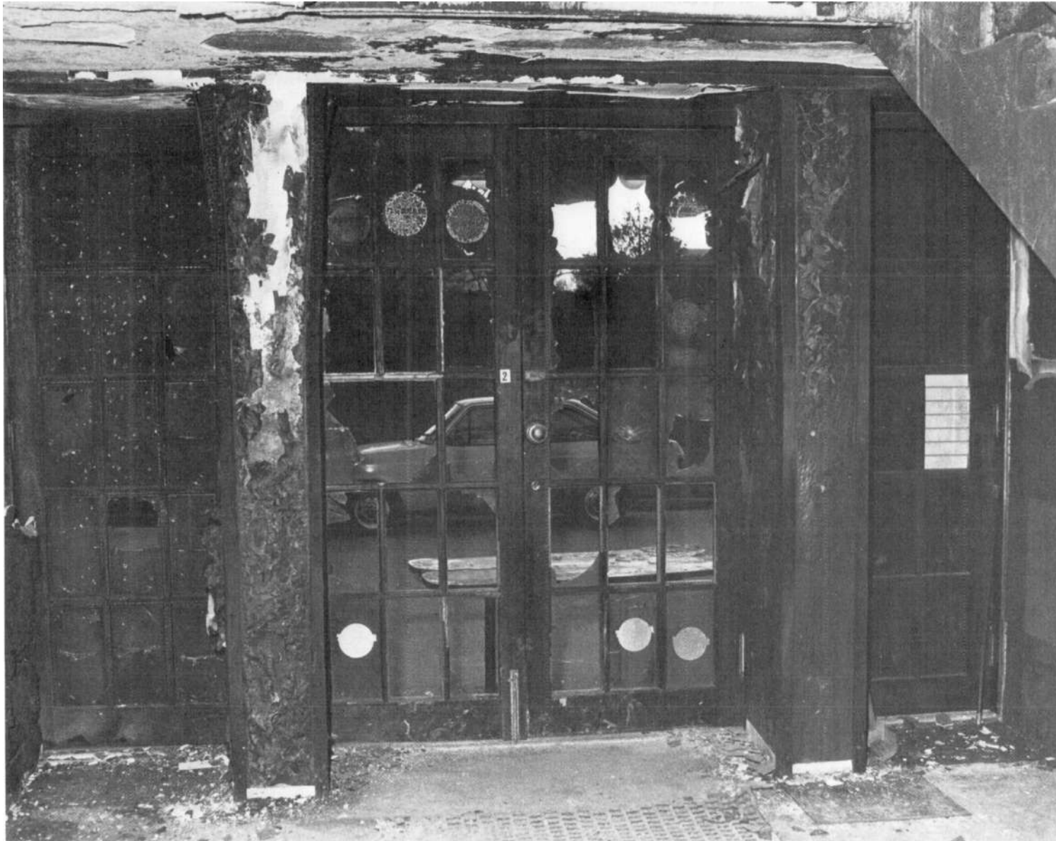
Plate 25 — Internal view of main entrance doors (Exit 2); the locked side-leaves are to be see
