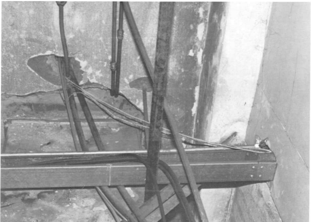
Plate 16 — Photograph showing typical electrical trunking installation-with covers removed; ceiling void over Lantern Room.
