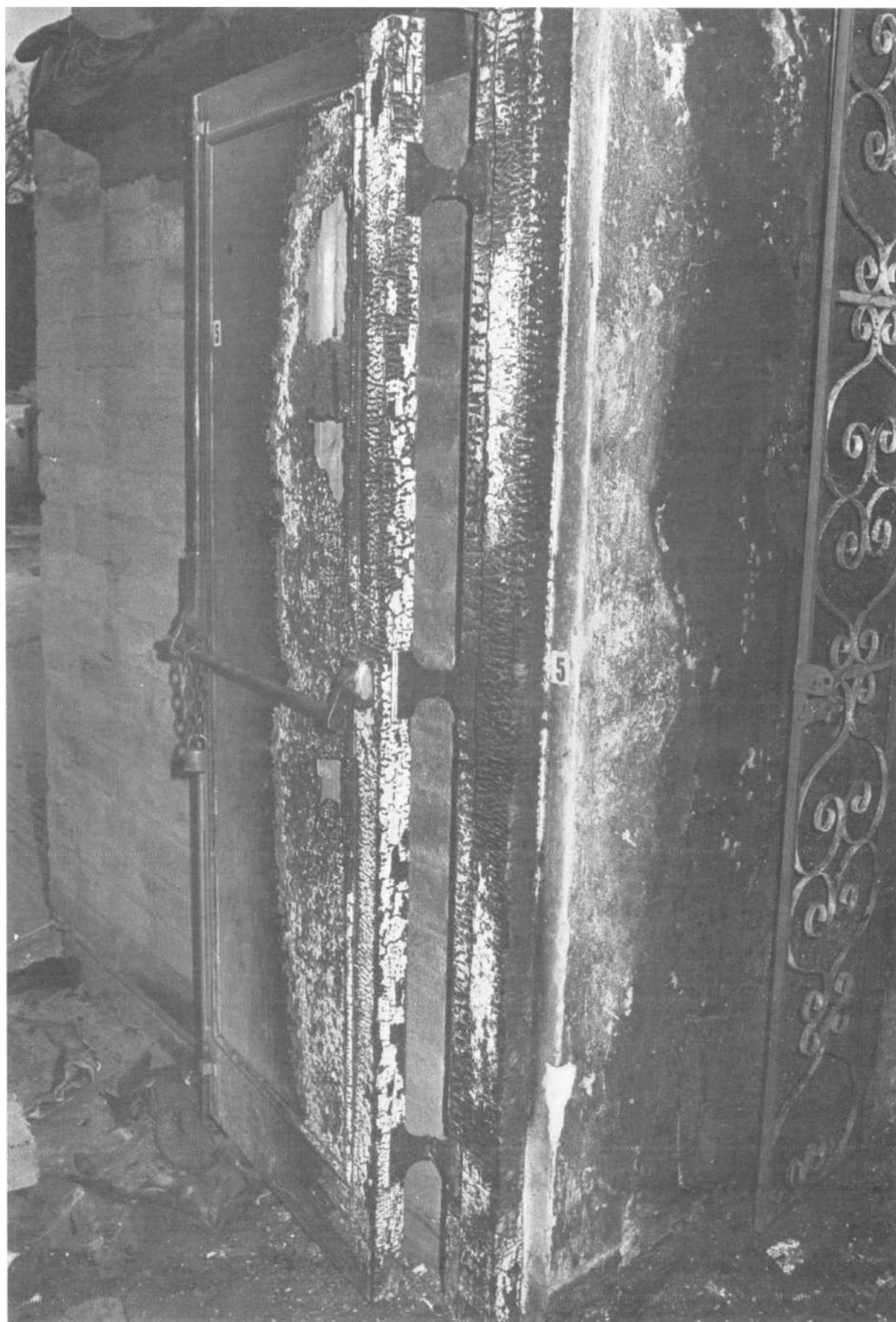
Plate 39 — View of right-hand door and frame of Exit 5; note edges of door and frame fire-damaged; the wall of the store used by the barmen of Bar 2 is visible to left of picture.
