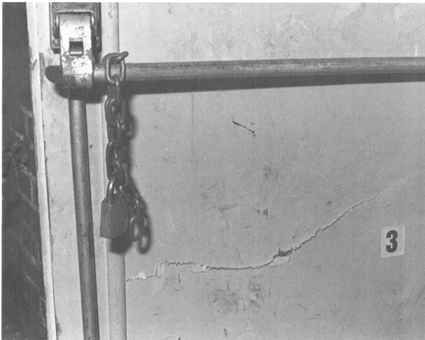
Plate 33 — View of outer Exit 3 showing horizontal bar and damaged plywood. See also chain secured
