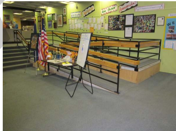
Ramp access to raised classroom level
