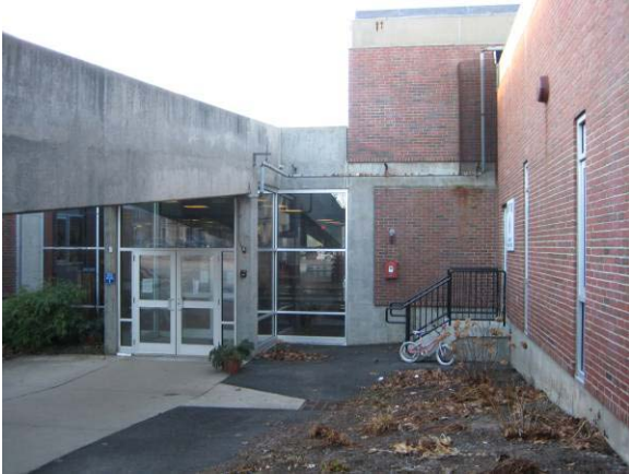
Brackett Street entrance with ramp above
