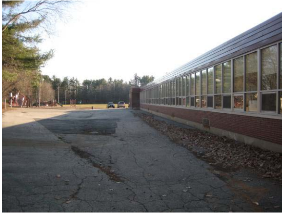
Pavement on north side of building
