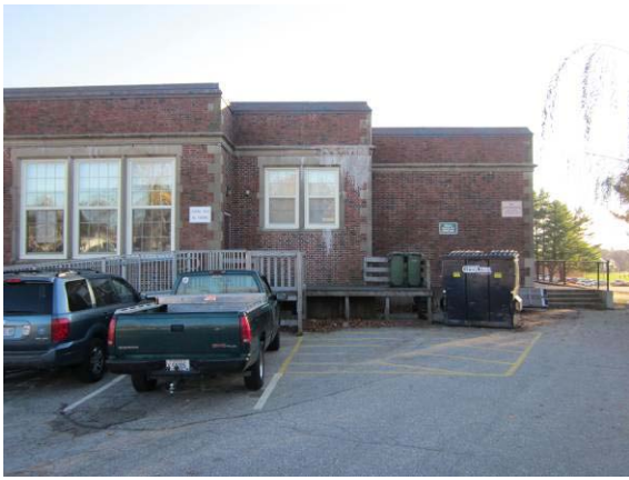
Handicap ramp and delivery entrance
