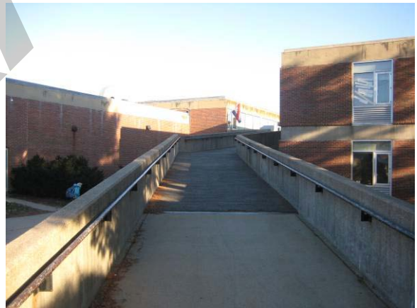
Second floor access ramp (Clark Street side)
