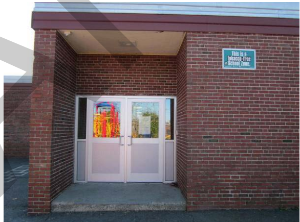
North side of building exit
