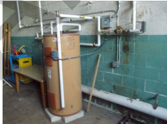
Electric water heater
