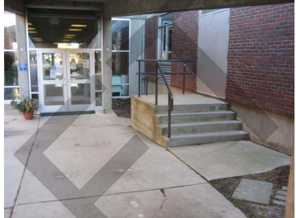
Clark Street entrance with ramp above
