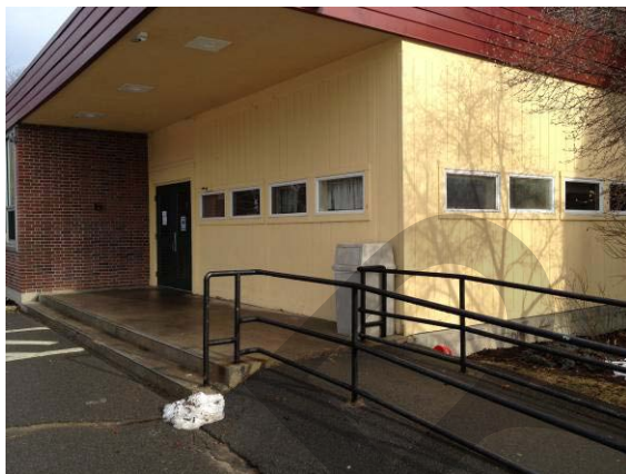
Main entrance and ADA ramp
