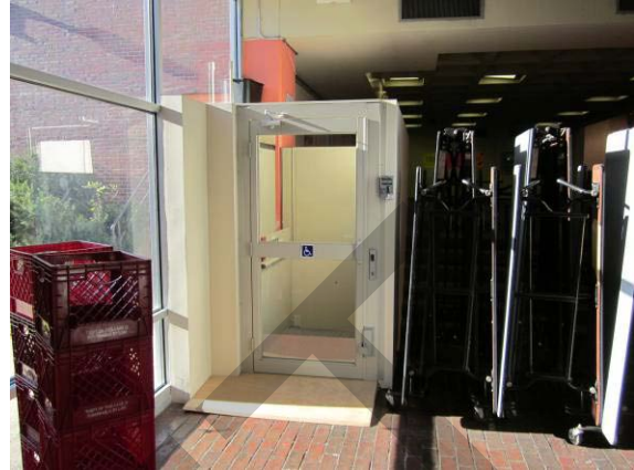
Entrance lift to raised cafeteria/auditorium level
