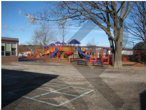
Hard court and playground
