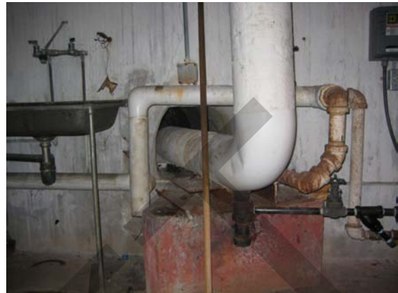
Utility trench beneath building
