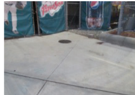
Fig 024. Fairly Recent Concrete Sidewalk/Paving
