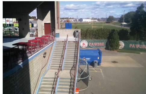
Fig 115. Concourse Stair To VIP Party Tent
