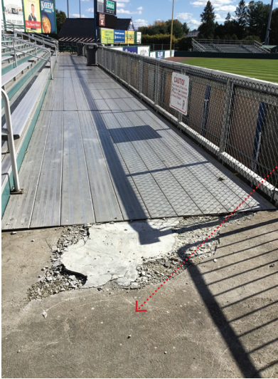
Fig. 031. Bleacher Construction Joint
