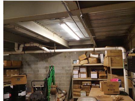
Fig. 060. Exposed PVC Piping Within The Out-Building
