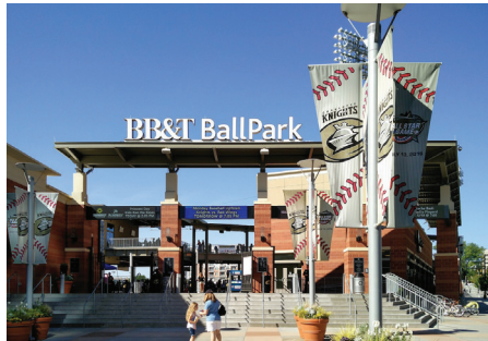
Fig. 233. Main Entry Grand Stair - Urban Edge
