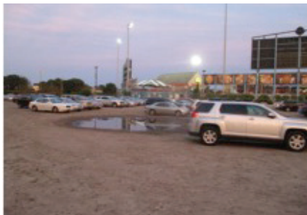
Fig. 020. Example of Ponding Water
