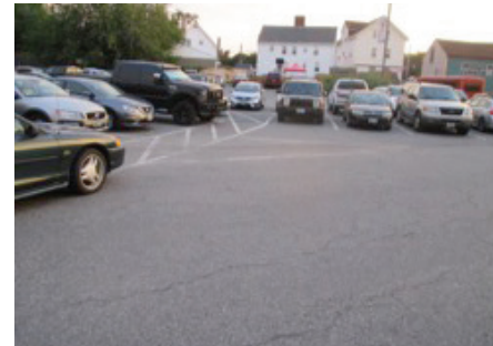
Fig 022. Example of Typical Pavement Cracking
