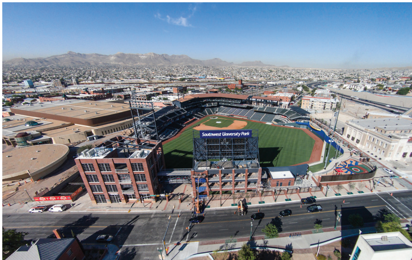
Fig. 212. Southwest University Park Aerial View
