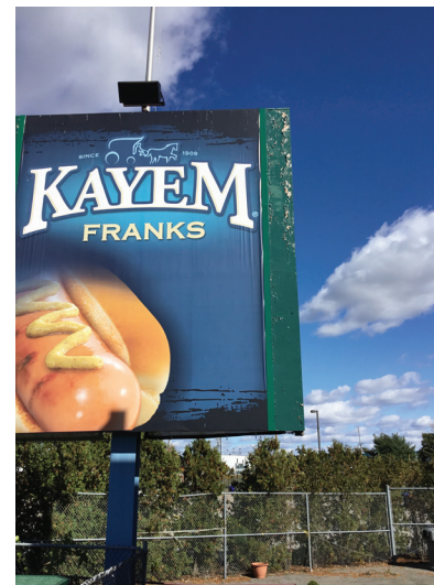
Fig. 170. Deteriorated Sponsor Signage
