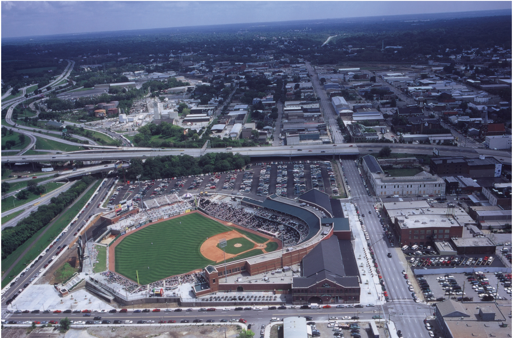
Fig. 183. Slugger Field Aerial View
