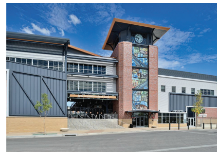
Fig. 221. Home Plate VIP & Administration Entry
