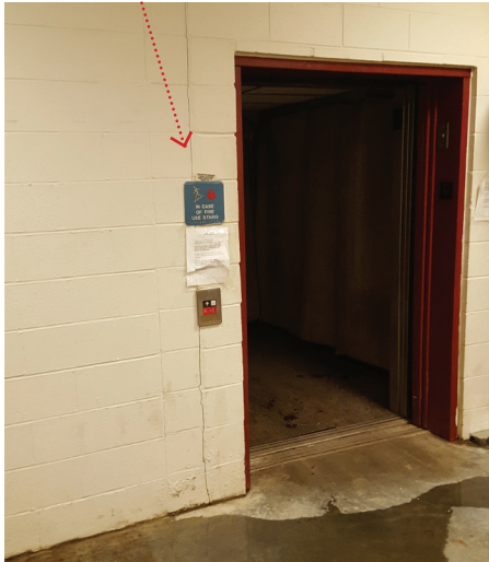
Fig. 066. Areas Of Water Infiltration @ Deck Drains
