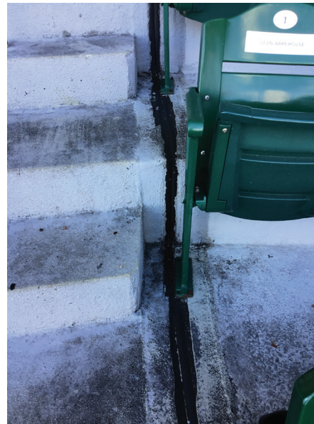
Fig. 102. Seating Straddling Expansion Joint
