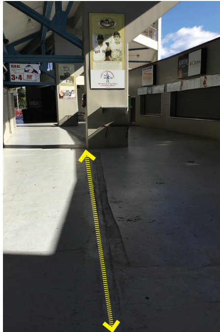
Fig 037. Sample Construction Joint
