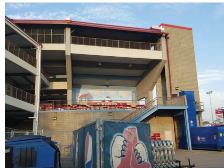
Fig. 072. Trash Adjacent To Public Concourse
