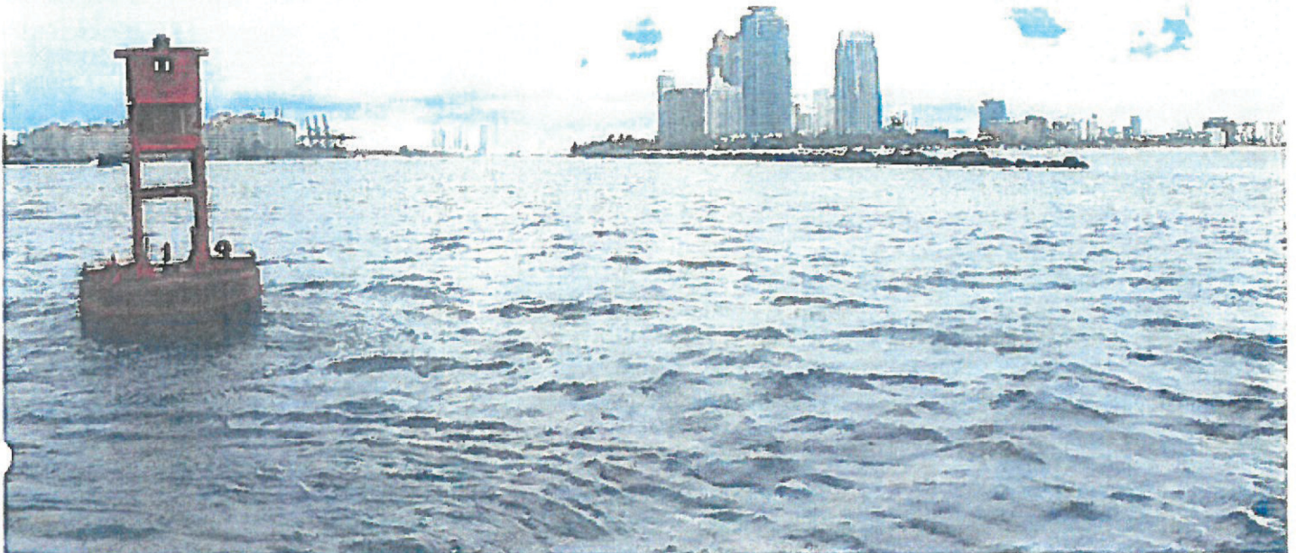
Fig. 17. Red Channel marker #12 and the east tip of the exposed Government Cut jetty.
