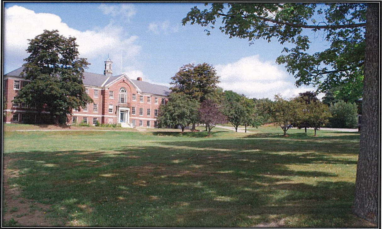
Historic Stevens Building and Preserved Open Quad
