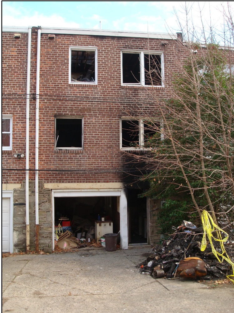
Photo 2. Rear of row house. (NIOSH photo.)
