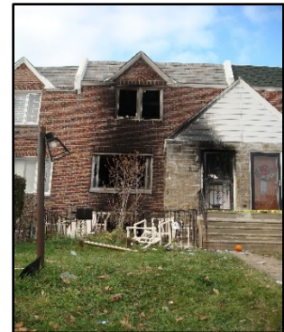
Side Alpha of the fire building (NIOSH photo.)
