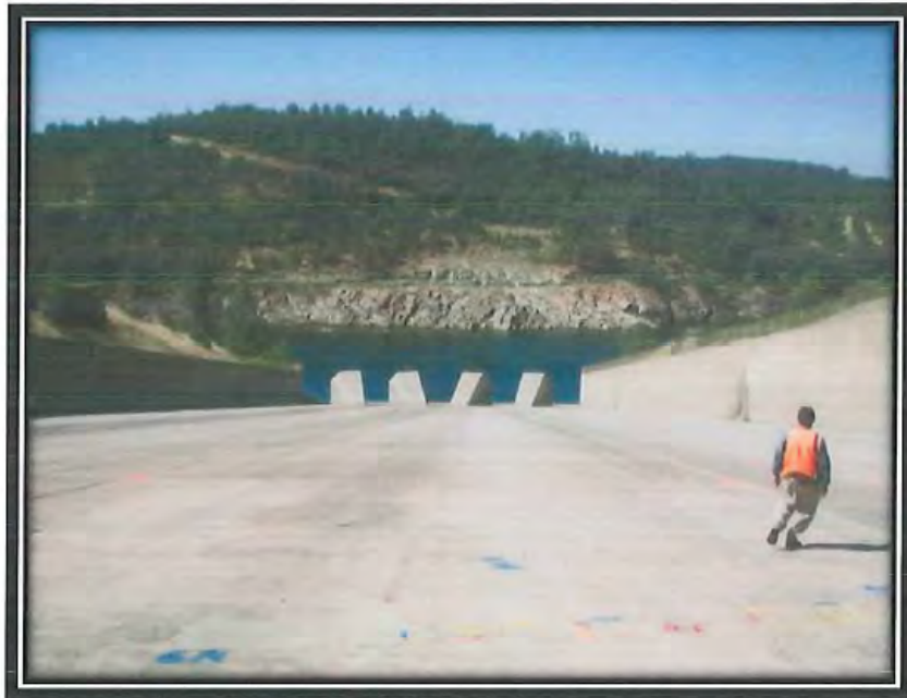
21. The lower flood control outlet chute is shown. Not the markings for the upcoming chute repairs. 6/25/10 Inspection Report
