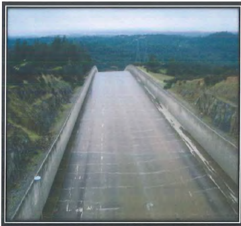
12. The concrete along the spillway chute has been repaired. The repaired herringbone crack pattern is said to reflect the underlying drain system.
