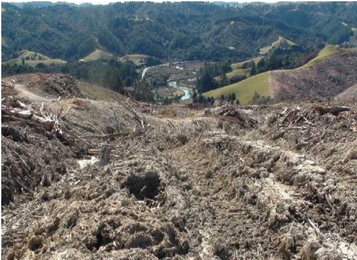
Figure 9: Example of a forestry road in Ngunguru forest showing potential run-off and sedimentation issues associated with road design and steepness. Photo Wade Doak. 28/08/2011
