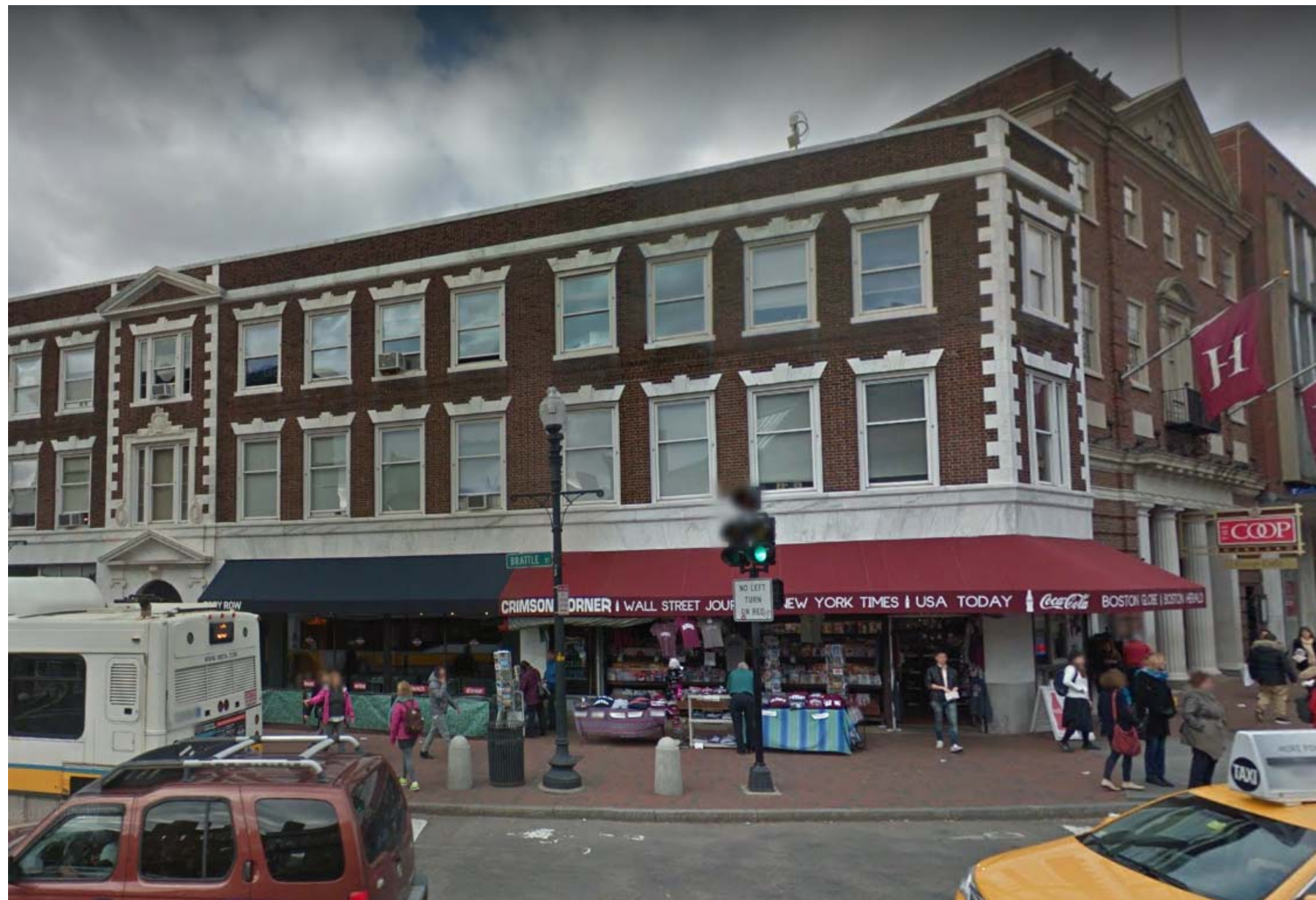
EXISTING EXTERIOR FACADE
