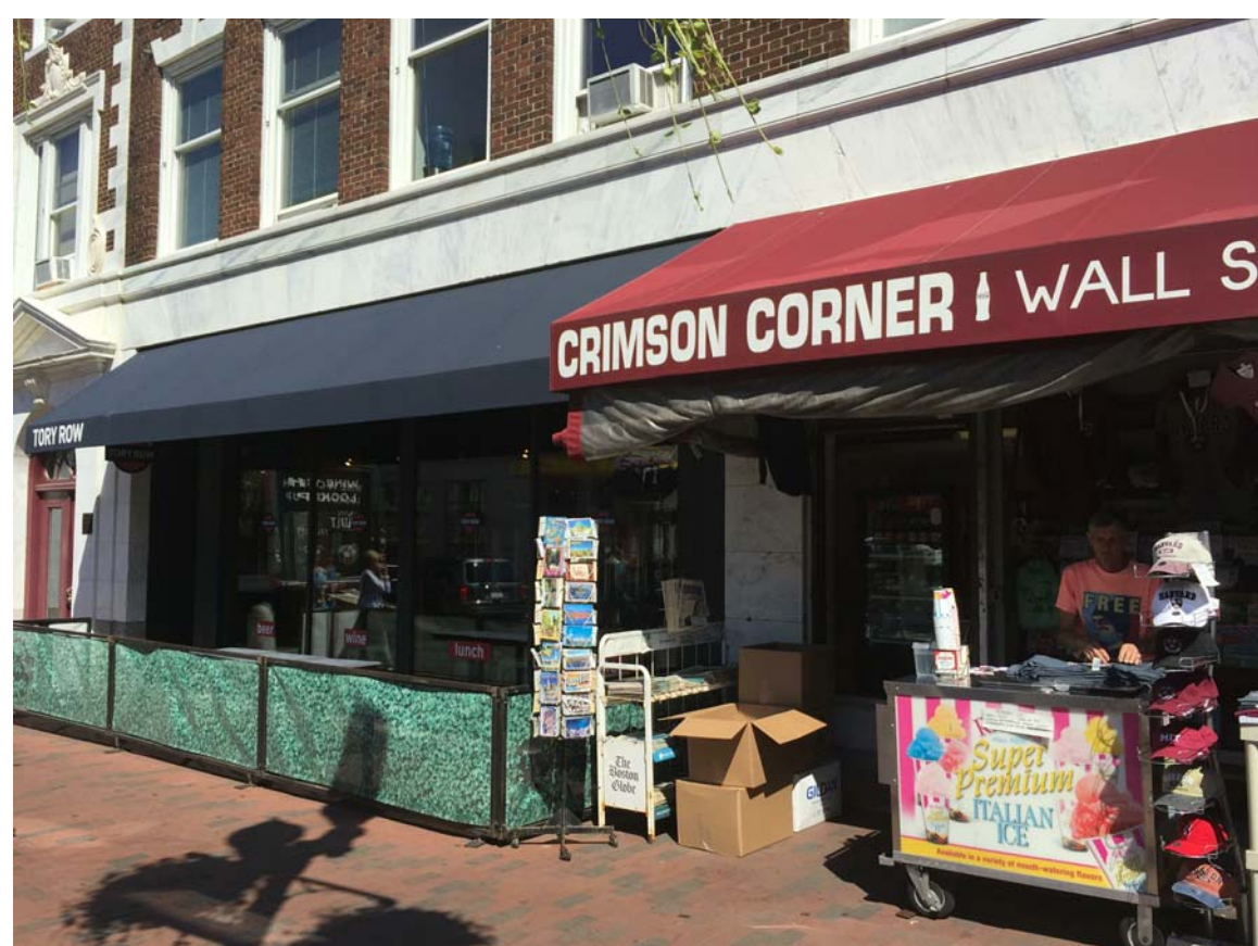
EXISTING TORY ROW AND CRIMSON CORNER FACADE CONDITIONS
