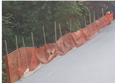
ORANGE SAFETY FENCING
