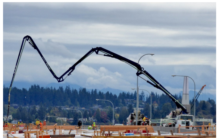
CONCRETE BOOM PUMP
