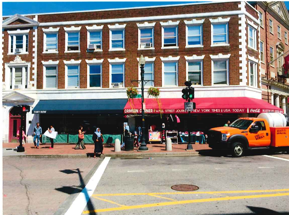
EXTERIOR FACADE AND STREET CONDITIONS. BIRCK AND MARBLE TO REMAIN AS IS
