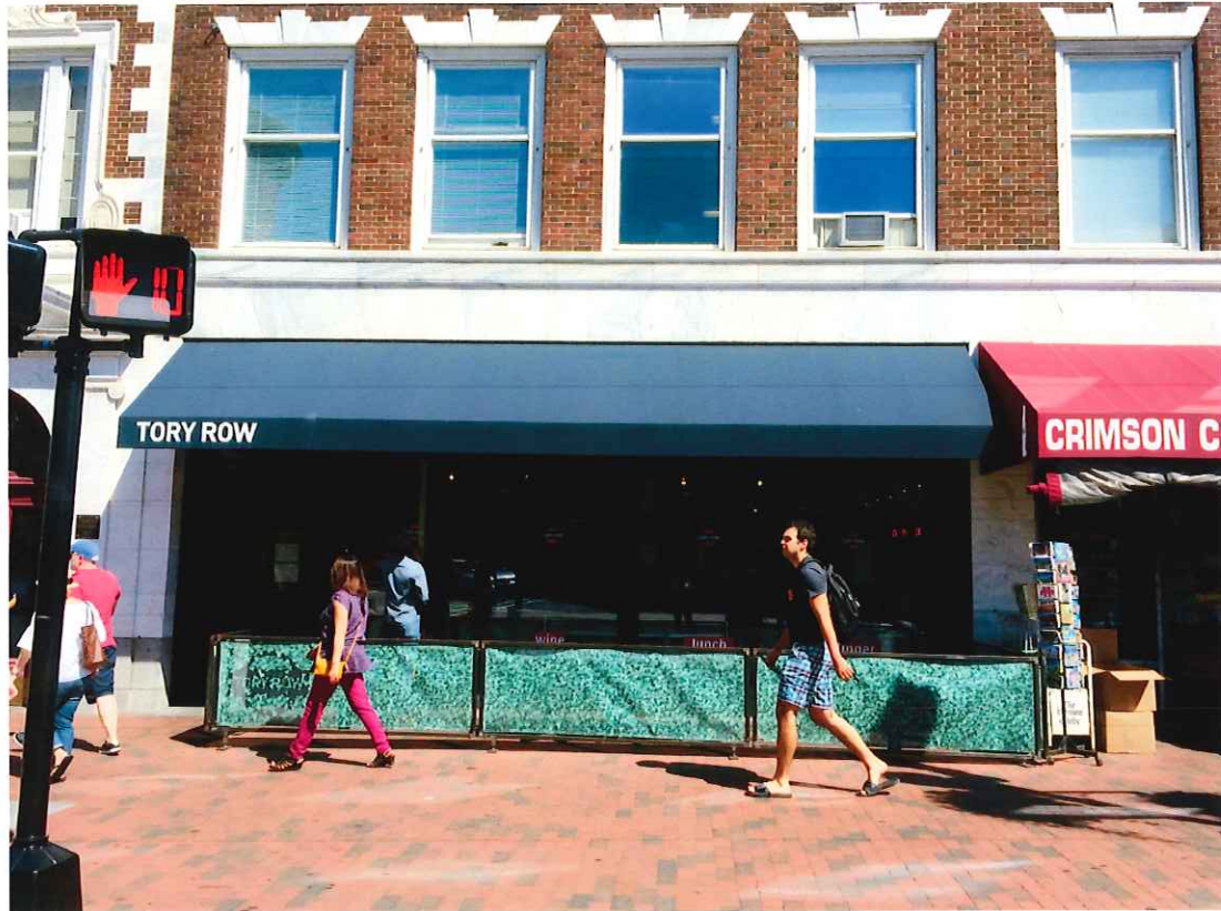
EXISTING TORY ROW FACADE AND PATIO CONDITIONS
