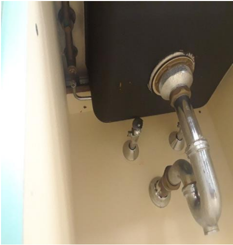
Sink with the water lines disconnected.
