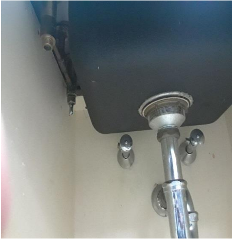
Sink with the water lines disconnected.
