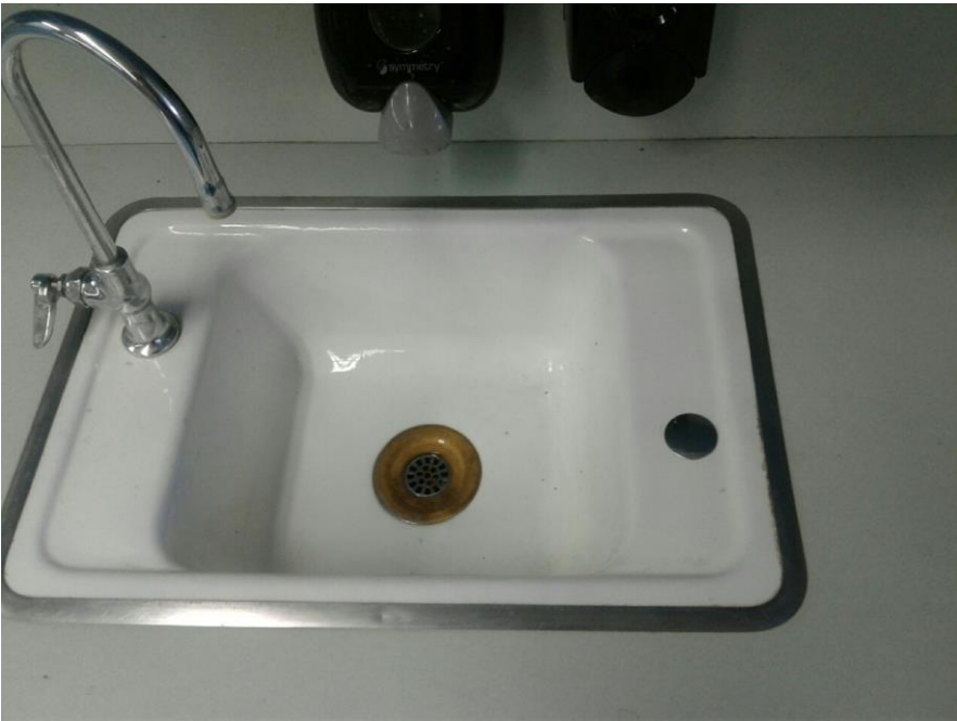
Bubbler with the bubbler removed.
