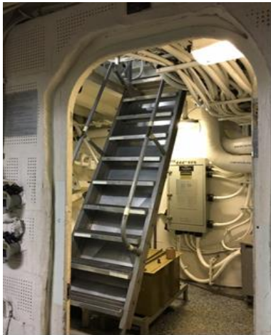
Figure 11 – Sample Berthing 2 Starboard Side Egress – Ladder Up
