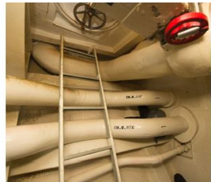
Figure 10 – Sample Berthing 2 Port Side Ladder through Escape Scuttle
