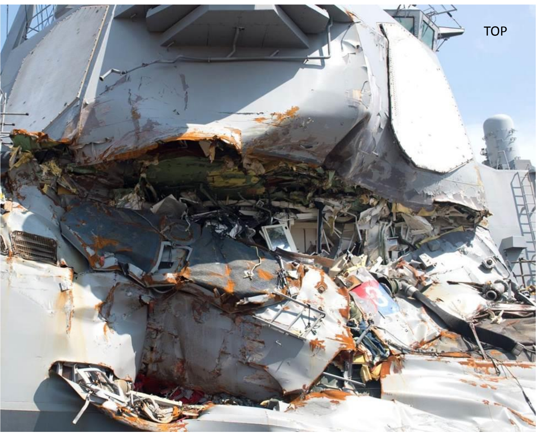
A1 : Commanding Officer's Stateroom on FTZ - Exterior View
