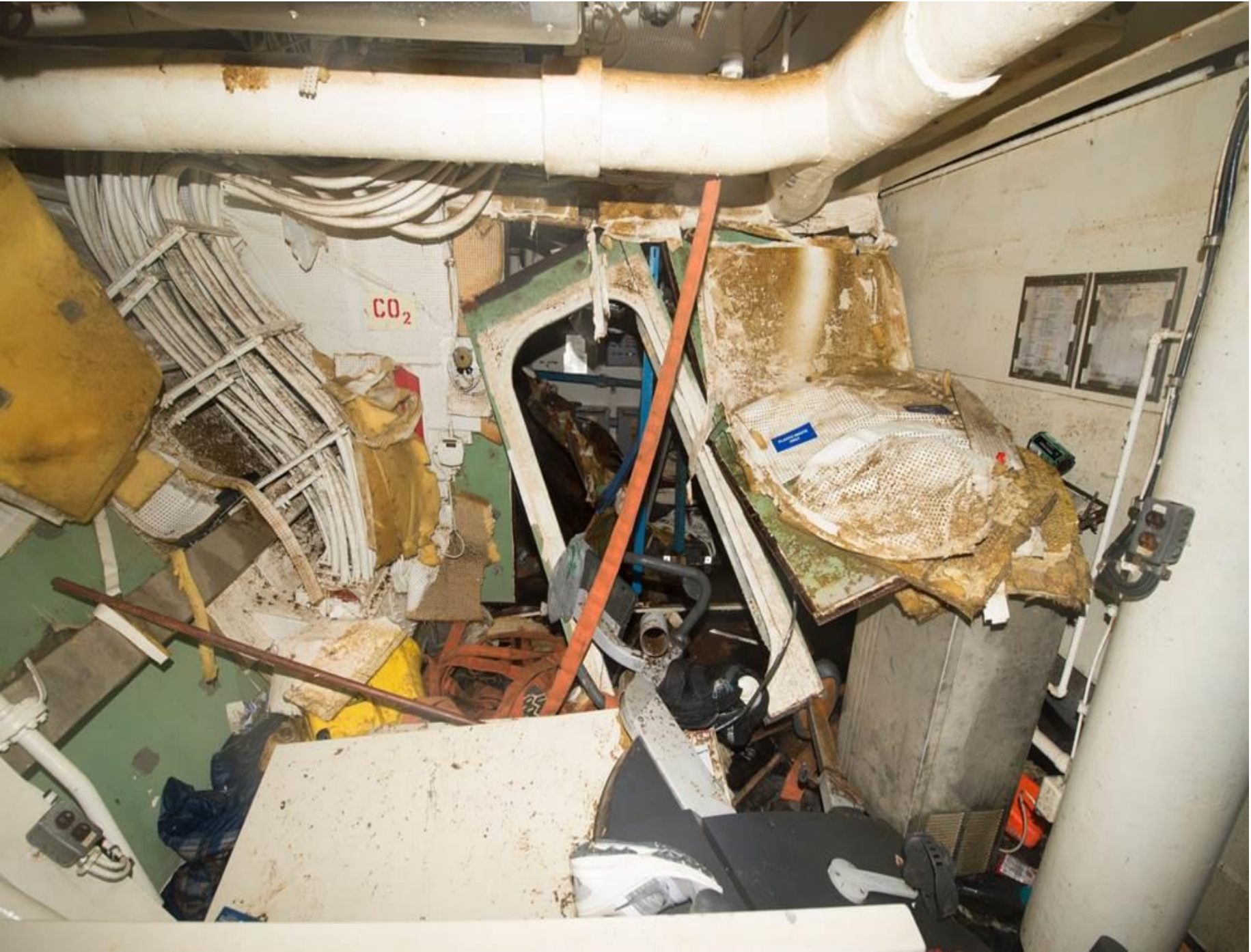
A5: Lounge in Berthing 2 - View from lounge facing egress
