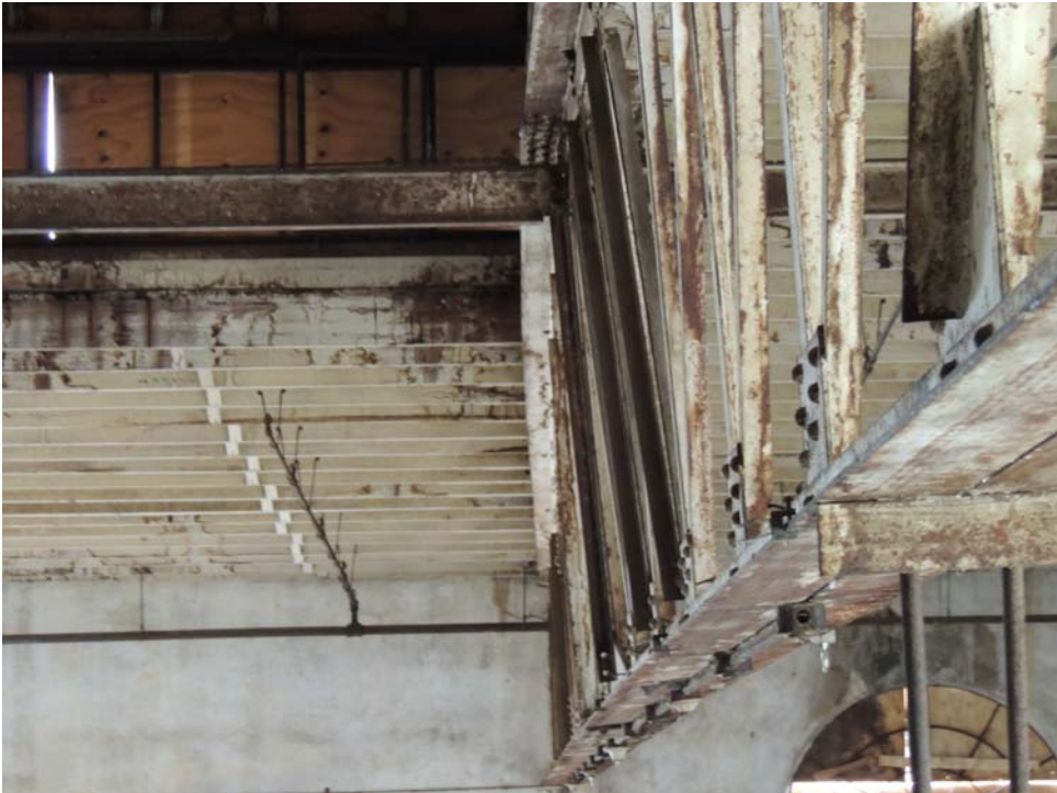
Figure 3: First Truss from West End 09-25-2017
