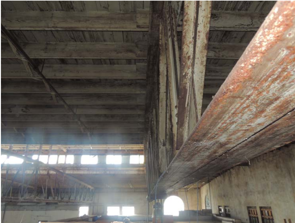
Figure 4: First Truss from West End 09-14-2015
