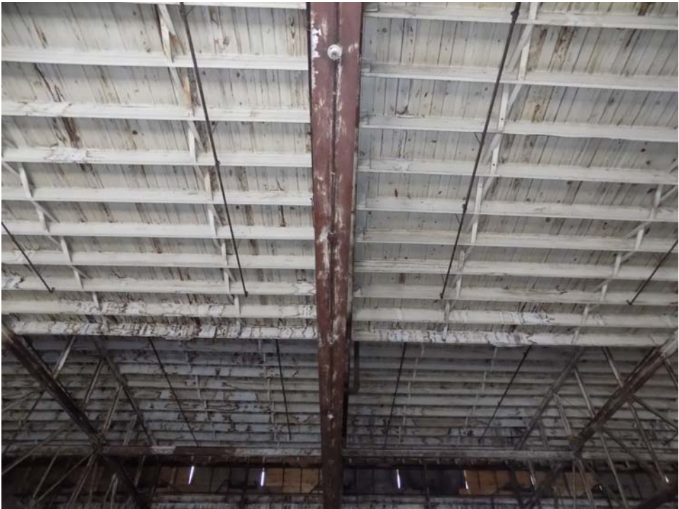
Figure 7: Third Truss from West End 09-25-2017
