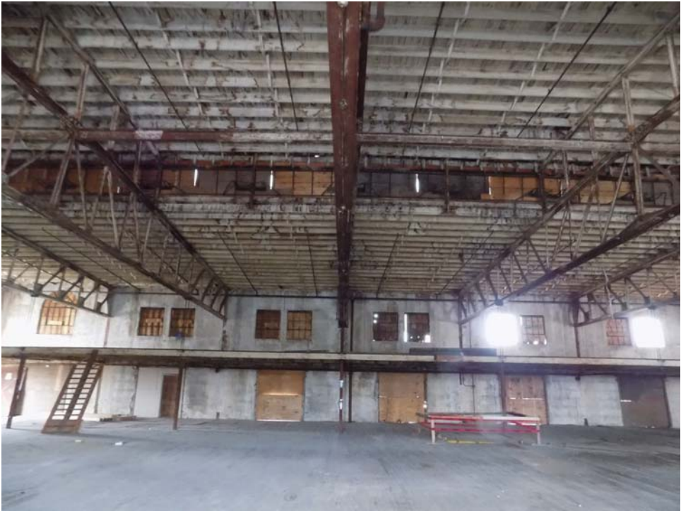
Figure 6: Third Truss from West End 09-25-2017
