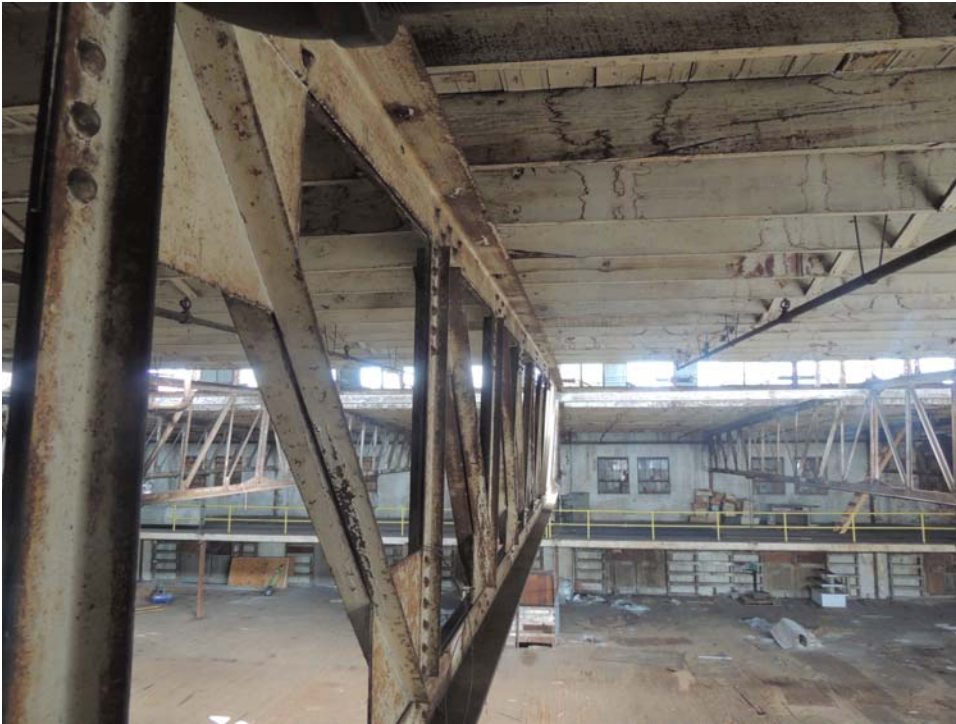
Figure 6: Third, Fourth & Fifth Truss from West End Looking N 09-14-2015
