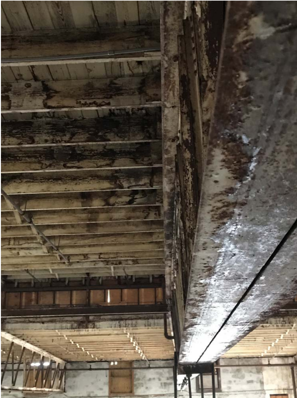
Figure 8: Third Truss from West End 09-25-2017
