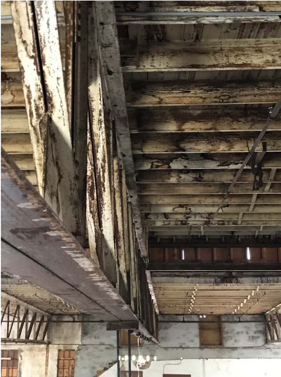
Figure 10: Fourth Truss from West End 09-25-2017
