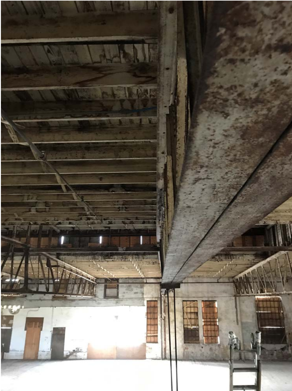
Figure 5: Second Truss from West End 09-25-2017
