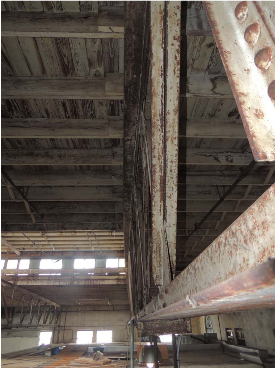
Figure 3: First Truss from West End 10-27-2015
