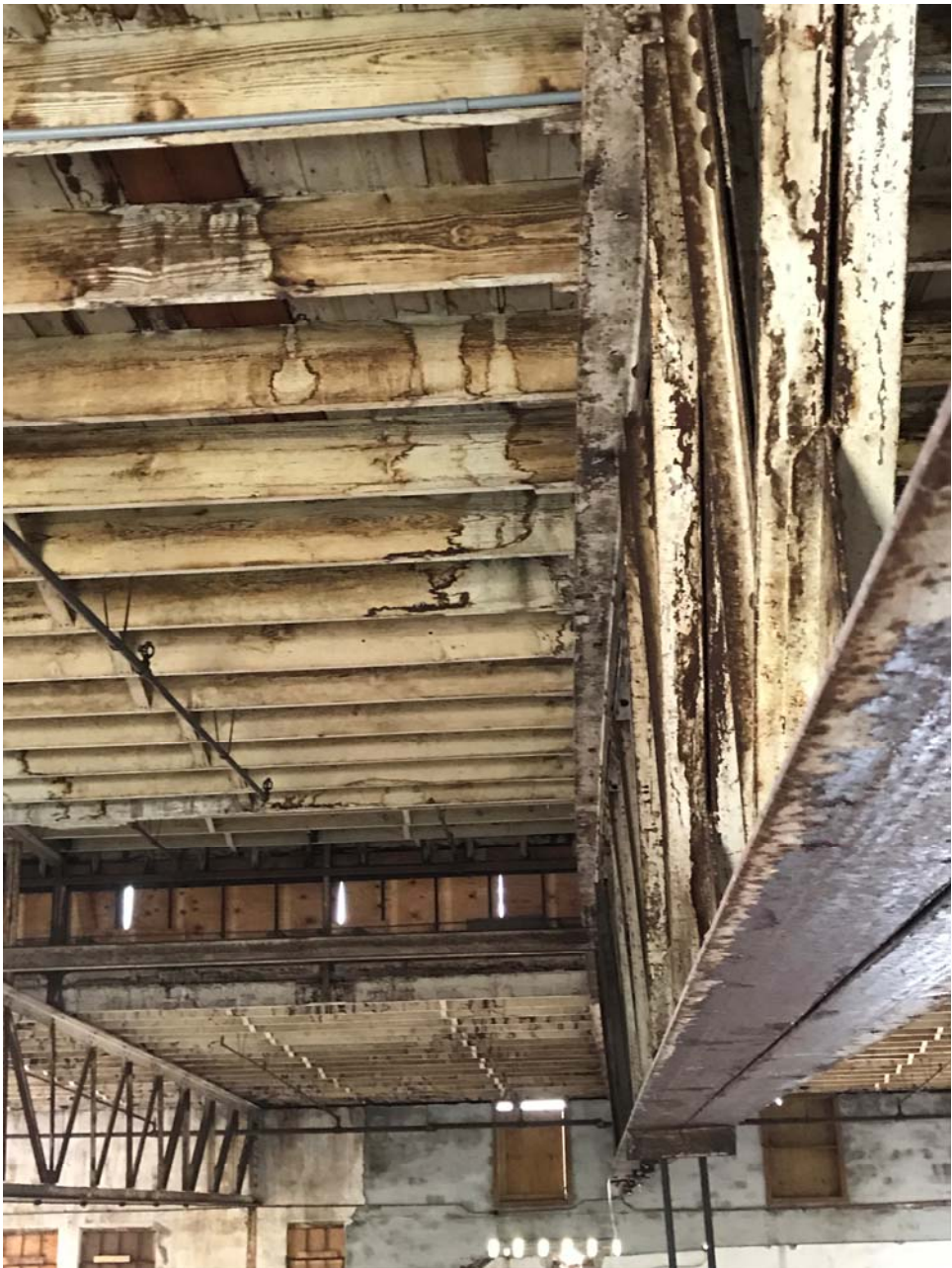
Figure 9: Fourth Truss from West End 09-25-2017
