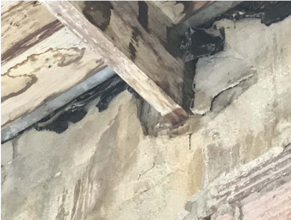
Figure 17: Timber roof rafter bearing at West Wall 09-25-2017
