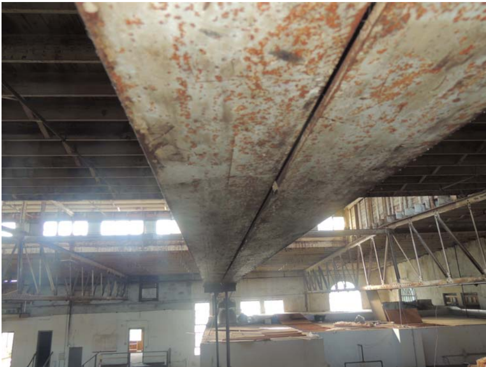
Figure 5: Second Truss from West End 09-14-2015
