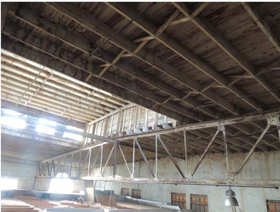
Figure 2: First Truss from West End 09-14-2015
