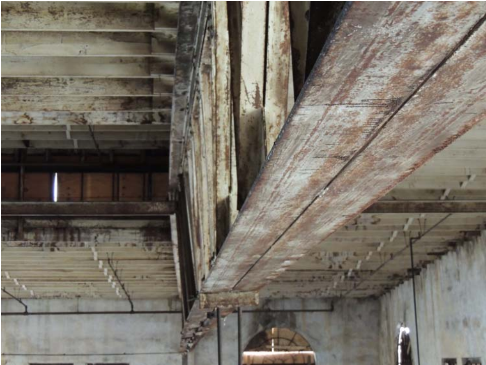
Figure 2: First Truss from West End 09-25-2017
