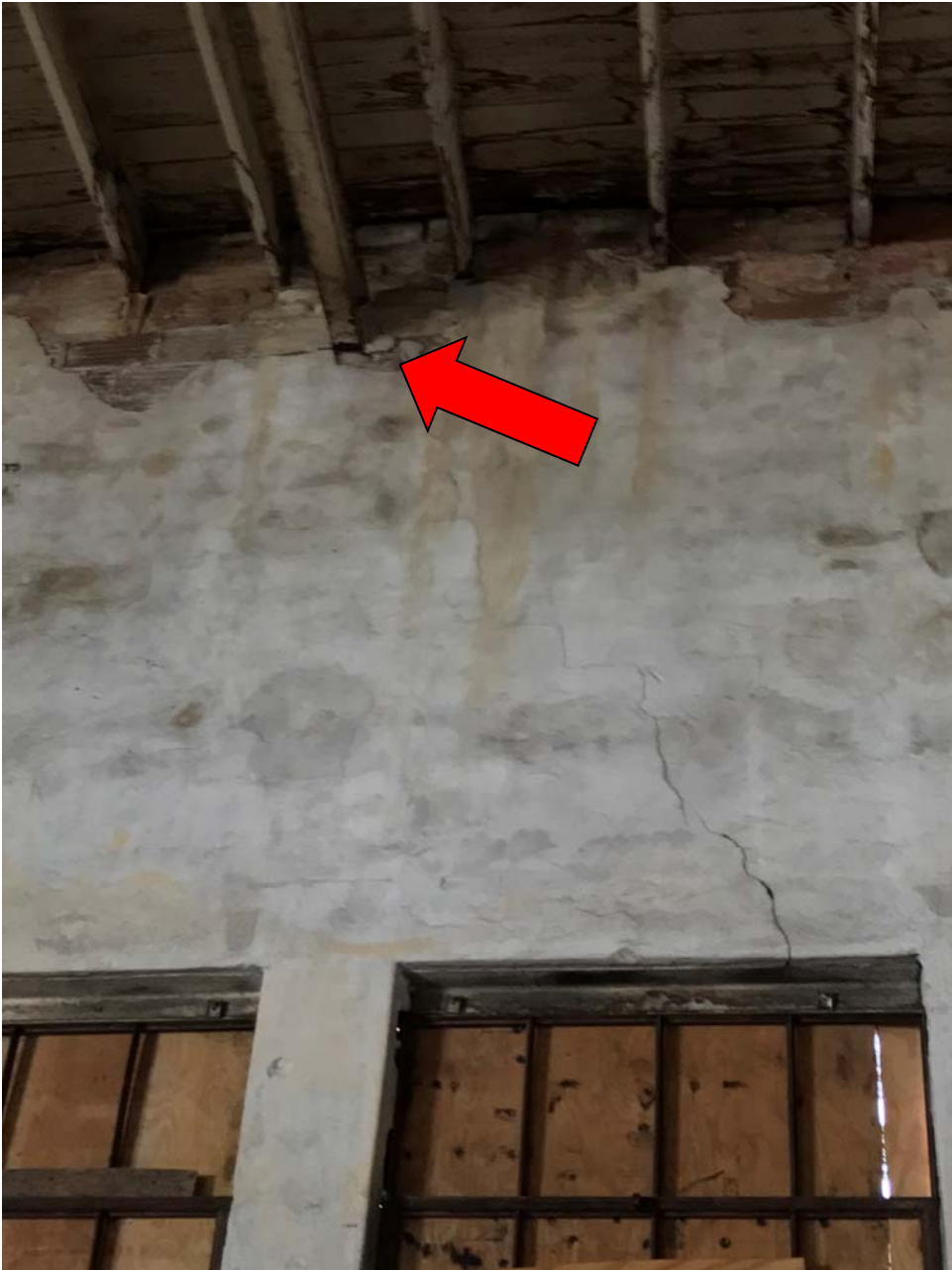
Figure 1: West Wall interface at single top chord truss brace 09-25-2017
