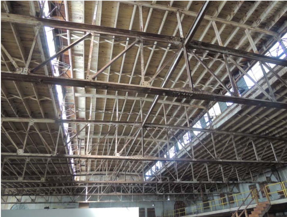
Figure 1: Roof Trusses 09-14-2015
