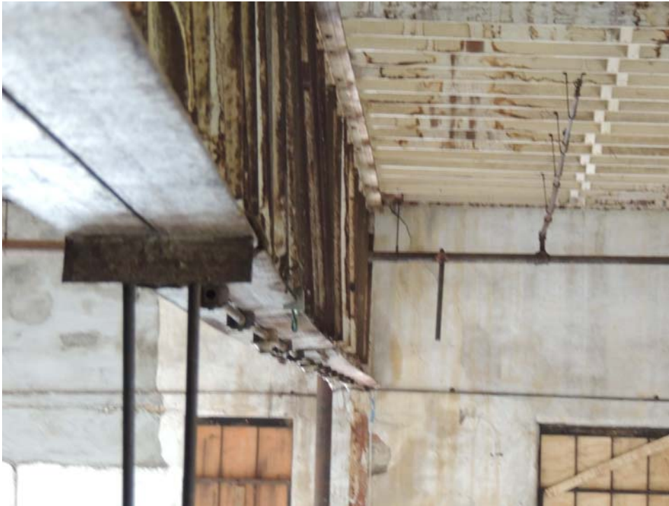
Figure 4: First Truss from West End 09-25-2017
