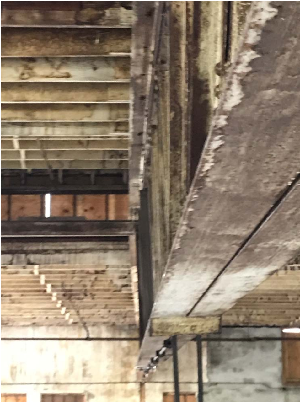
Figure 11: Fifth Truss from West End 09-25-2017
