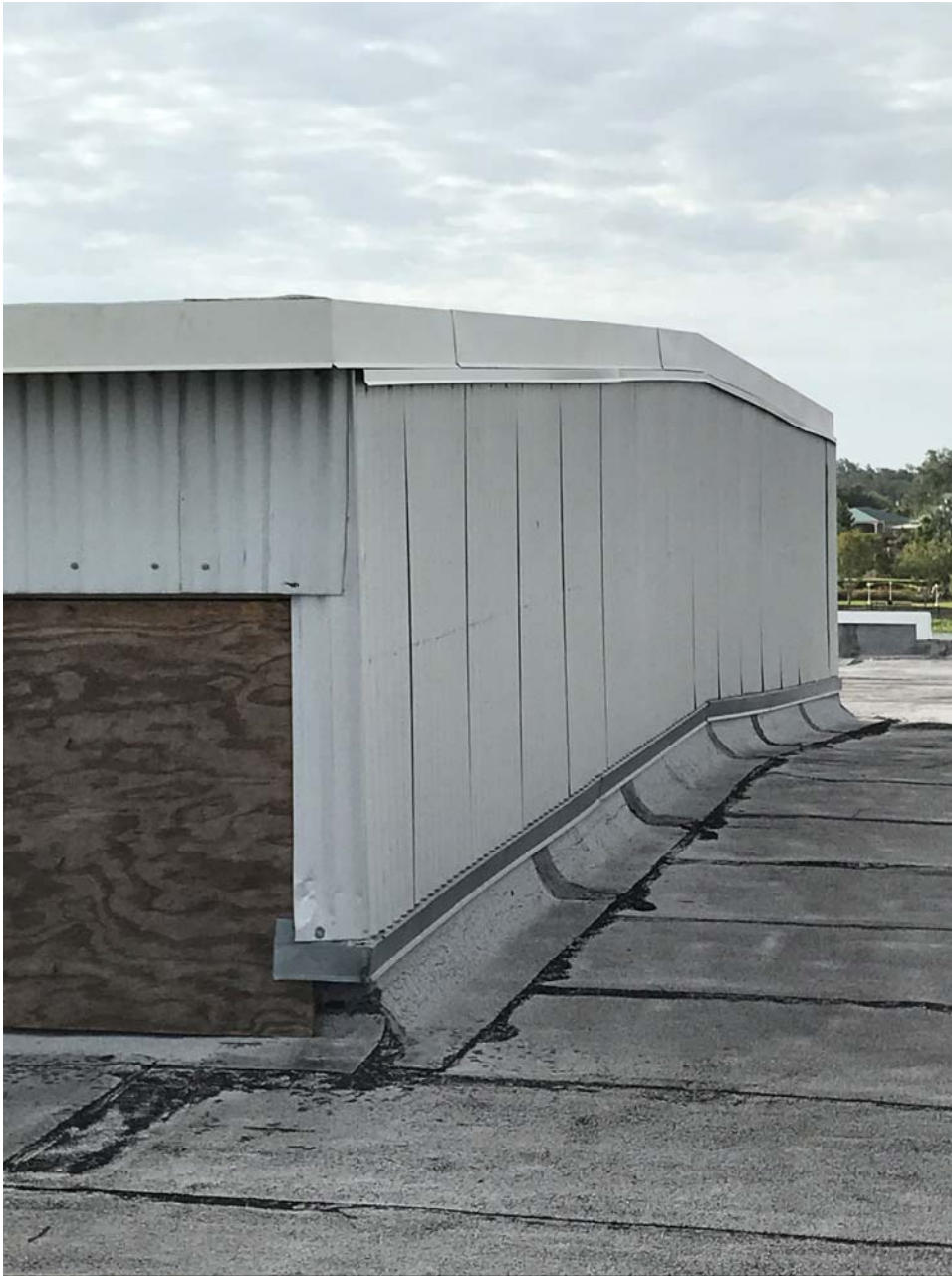
Figure 15: West end of Clearstory 09-25-2017
