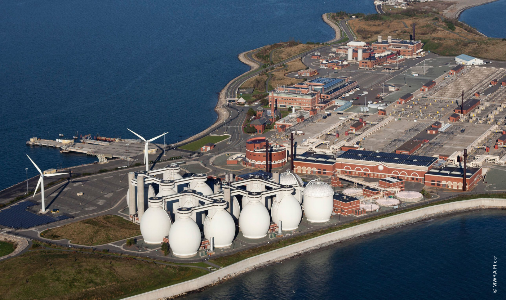
Anaerobic digesters, Deer Island
