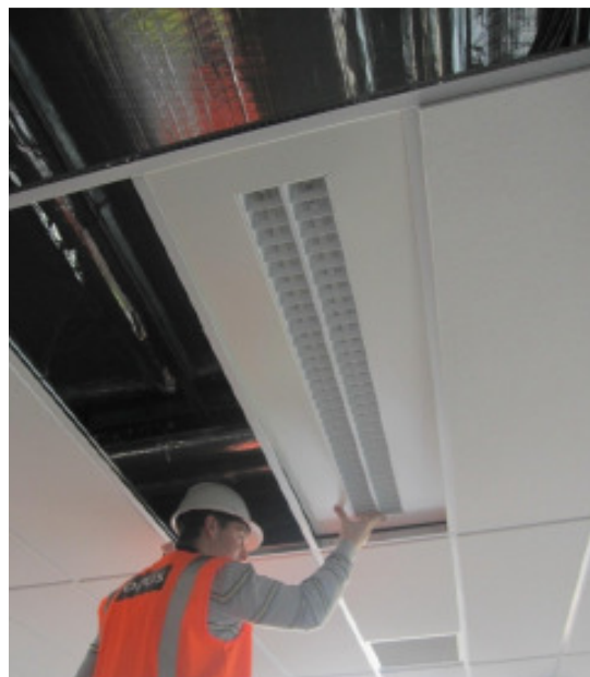
Figure 8: Unsecured recessed luminaires
