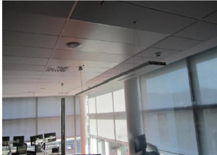
Figure 9: Typical suspended luminaire
