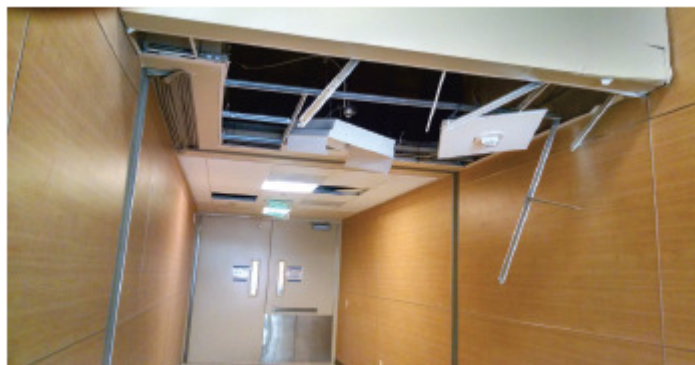
Figure 13: Ceiling damage in hospital corridor link
