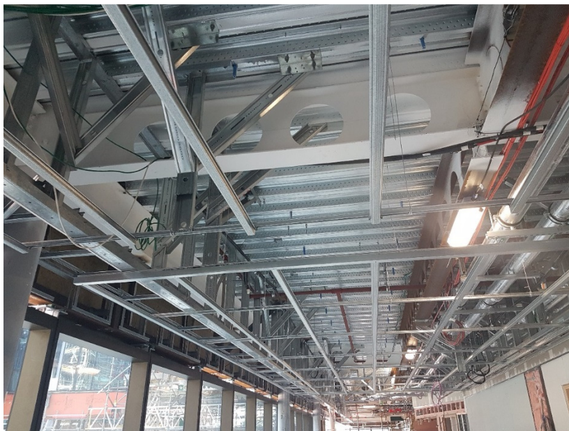
Figure 2: Seismic Restraint of Services and Ceilings
