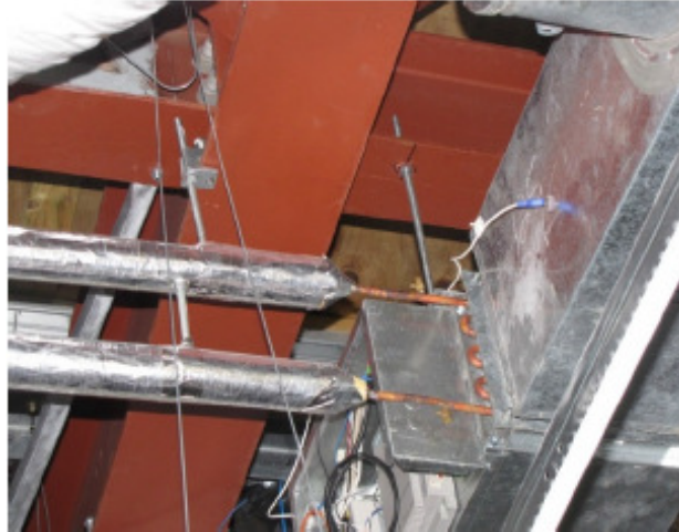
Figure 5: Lack of flexible connections to mechanical plant
