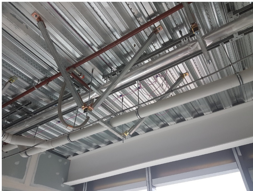
Figure 3: Seismic Restraint of services
