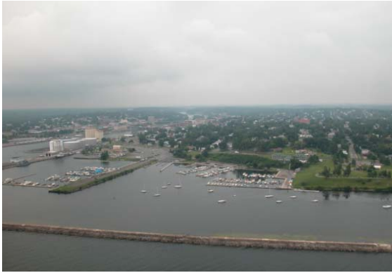
340 – Commercial / Industrial Docks/Piers/Wharves.
