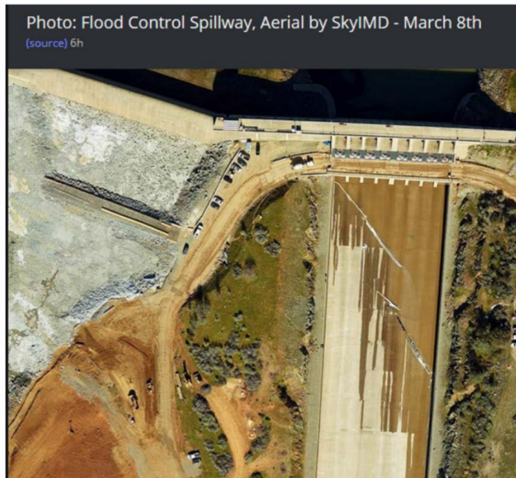
Figure F1-11: Aerial View of Service Spillway following the Incident
