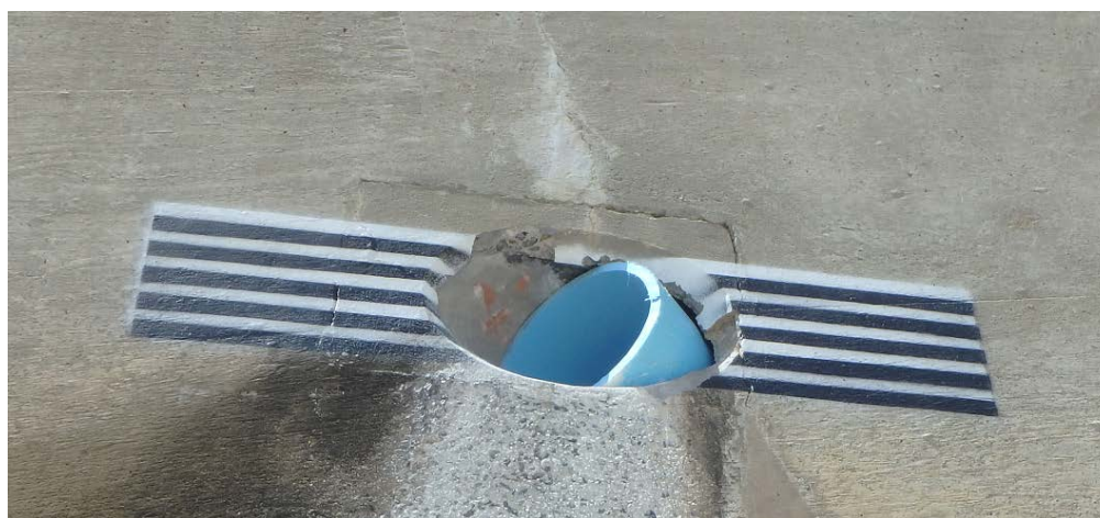
Figure D-39: Collector Pipe Outfall
