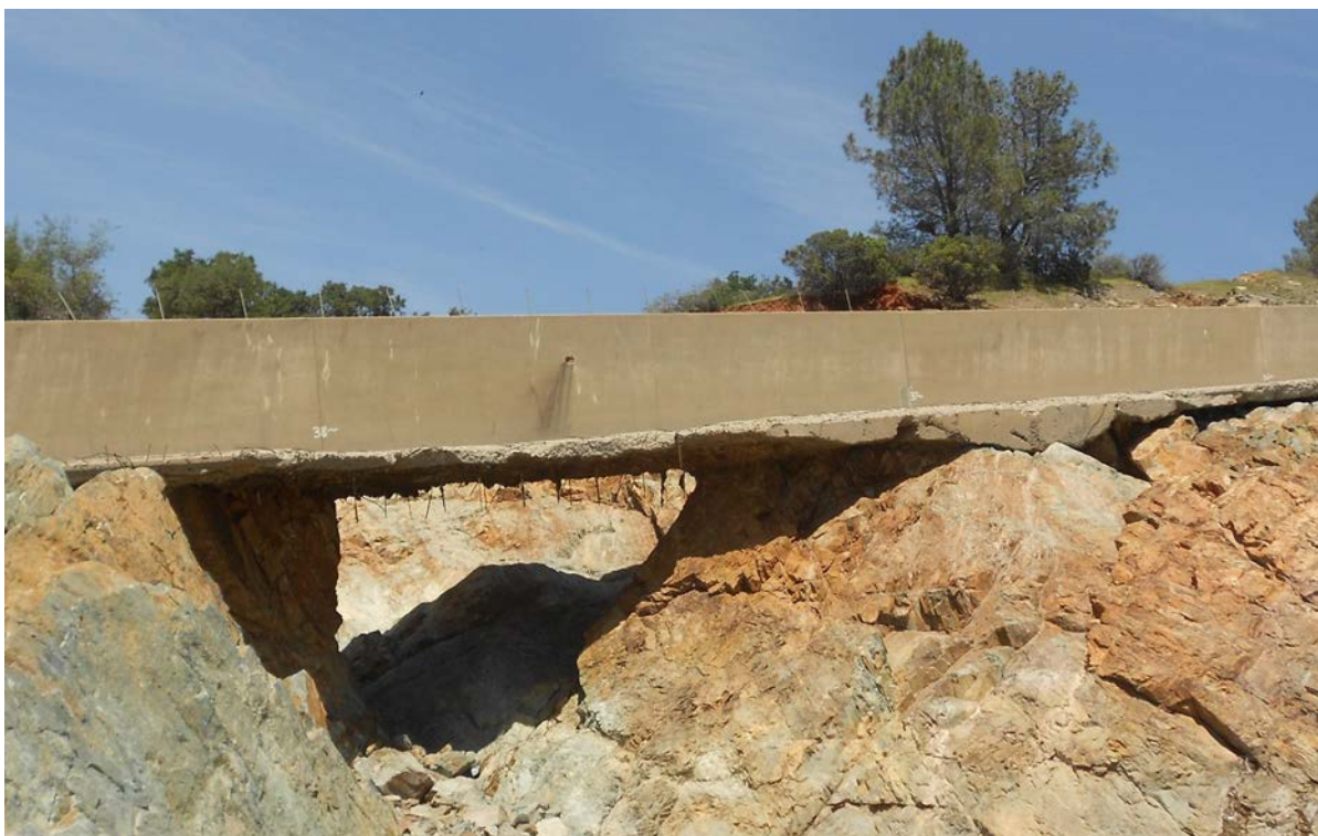
Figure D-12: Photograph of Erosional Feature Between Sta. 37+00 and Sta. 38+50 on Left Side of Lower Chute
