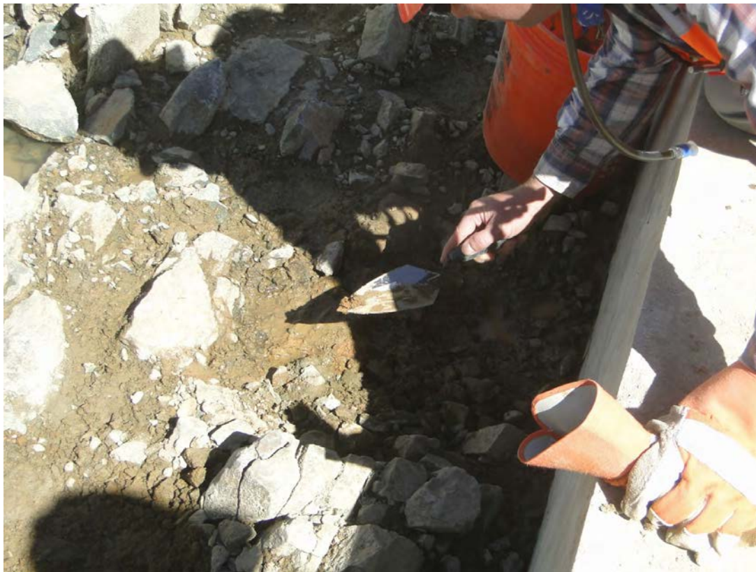
Figure D-7: Photograph Showing “Compacted Clayey Fines” in Forensic Trench 27C in Area D (approximately Sta. 26+85)
