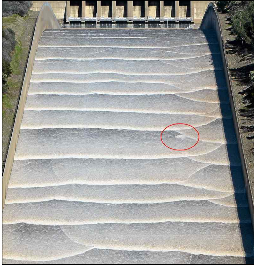
Figure B-2: Slug Flow in Spillway Chute. The circled area shows a flow disturbance at Station 33+00 for very low discharge. Reference [B-4]
