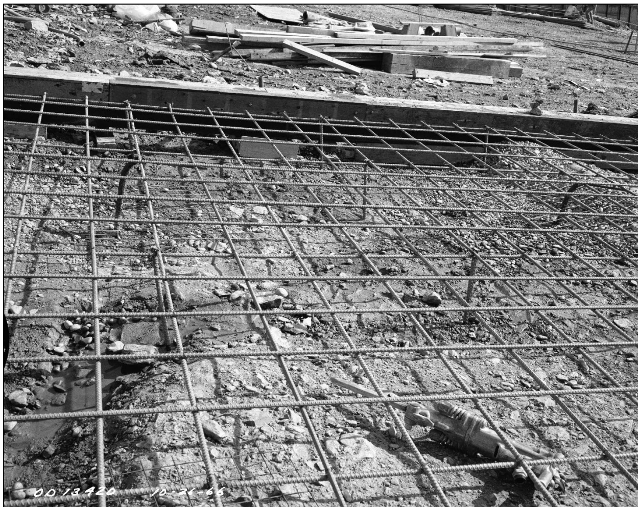
Figure A-16: Clean-up effort for the spillway chute prior to placement. Note that foot prints appear in the material left in place, and numerous rock fragments are present. This is believed to be in an area that required additional cleanup just upstream from Sta. 33+00. (Photo OD_13420_10_26_1966)
