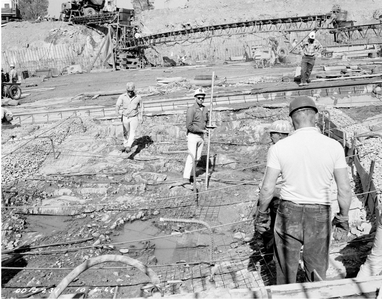
Figure A-13: Anchor Bars Installed on Uneven Rock Surface (Photo OD_13231_10_06_1966)
