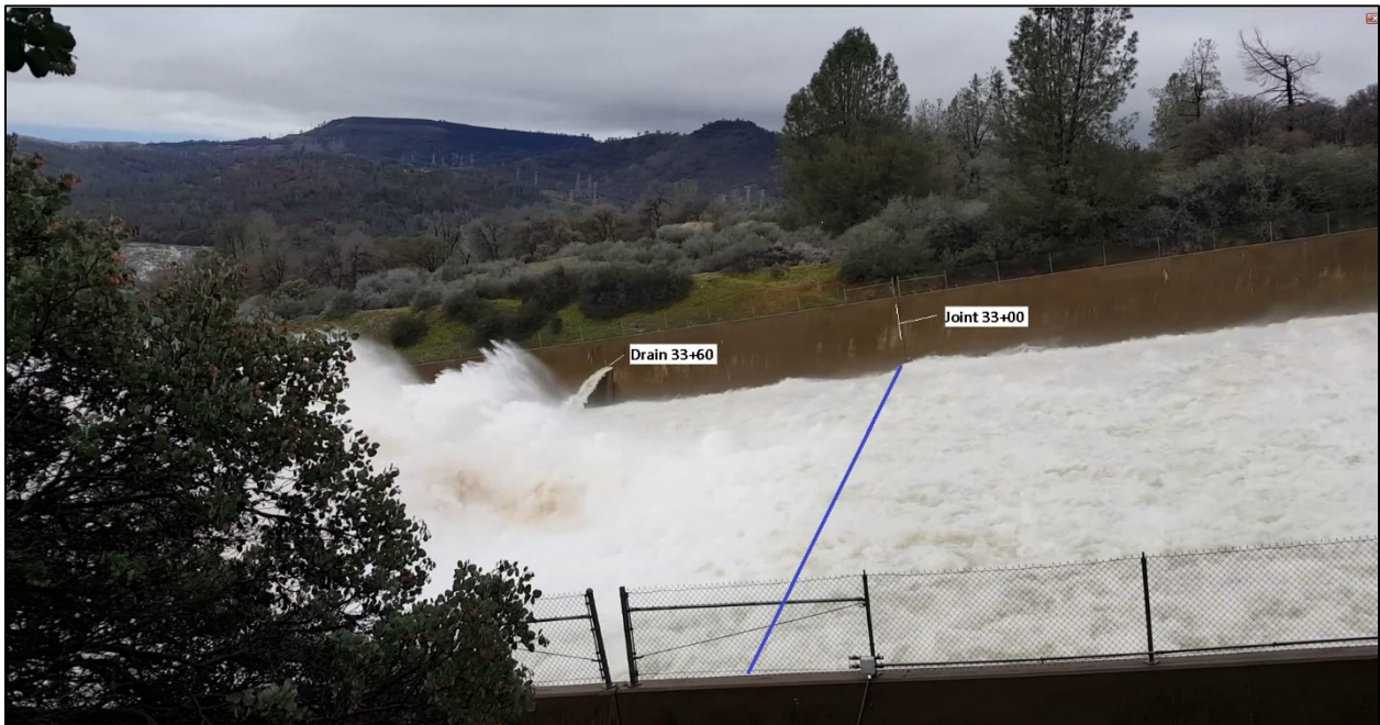
Figure I-5: Flow in Chute at 10:32 [I-2]
