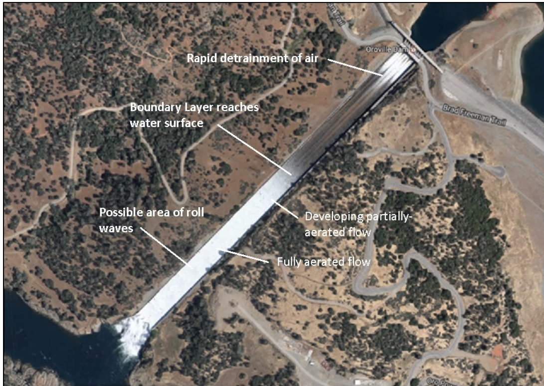
Figure B-5: Satellite Photo of Spillway Modified from Google Earth
