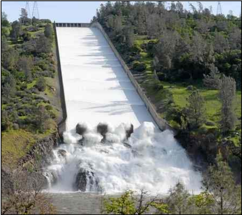
Figure 3-2: Oroville Dam service spillway
