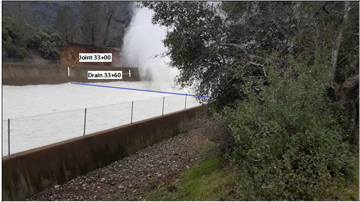
Figure I-8: Flow in Chute at 12:07 [I-2]
