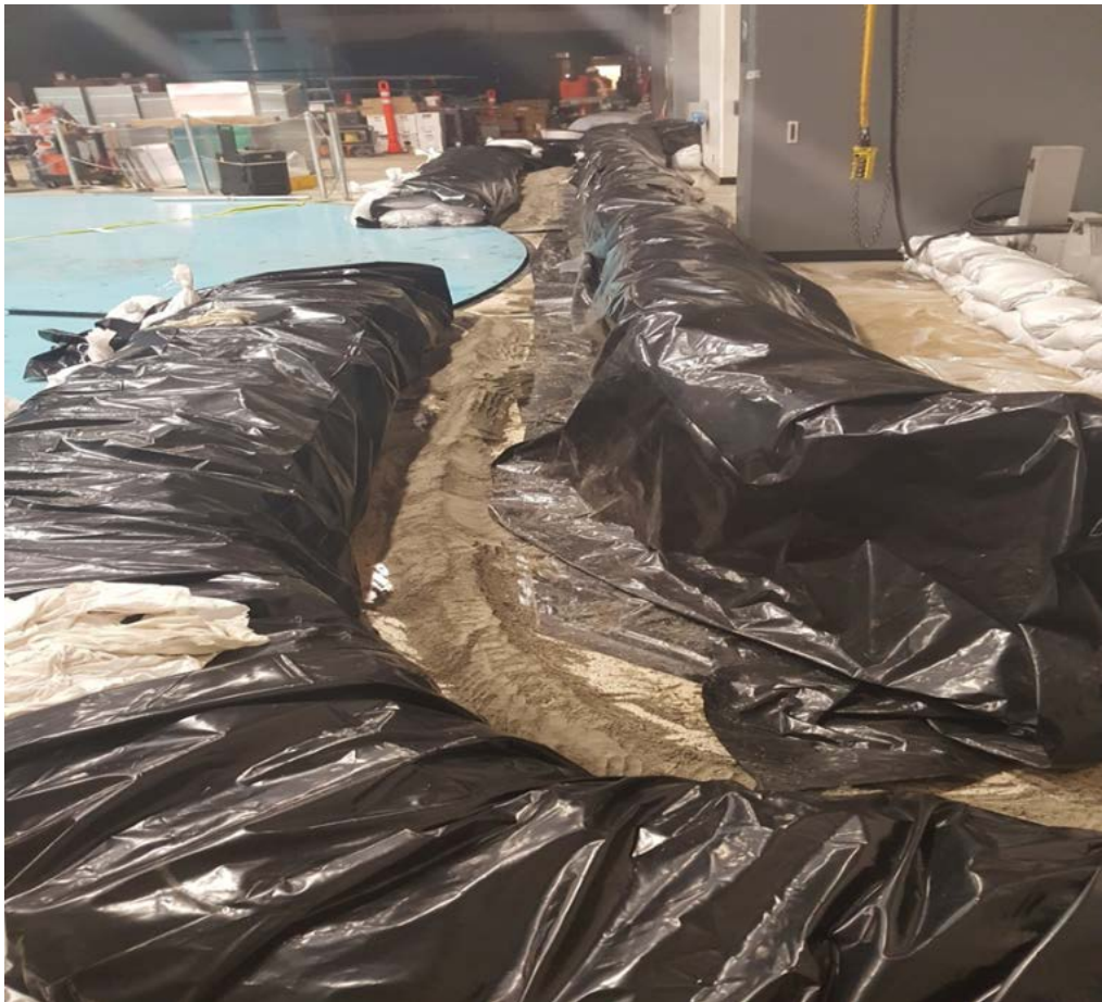
Figure L-3: Sandbags in Hyatt Powerhouse [L-4]
