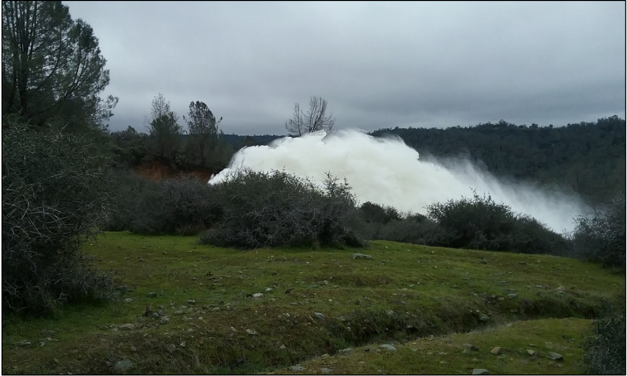
Figure I-6: Flow in Chute at 11:28 [I-3]
