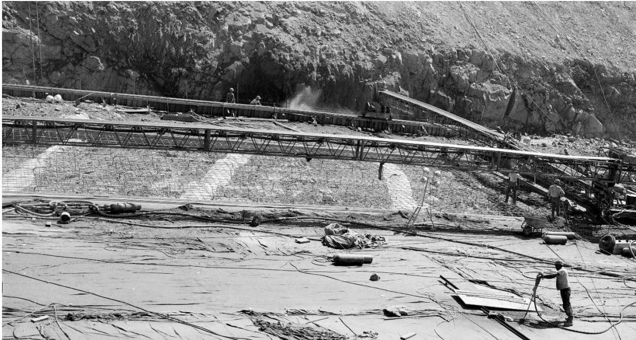
Figure E-4: Photo Showing Plastic Sheetting Over Drains (Dated 9/30/1966)
