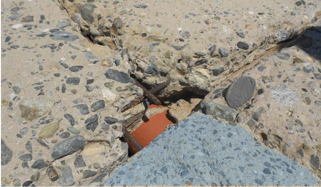
Figure D-14: Example of area of congested large-size aggregate over herringbone drain and reinforcement. Location at Sta. 42+00 and centerline. Area of repair patch concrete shaded (note smaller aggregate).
