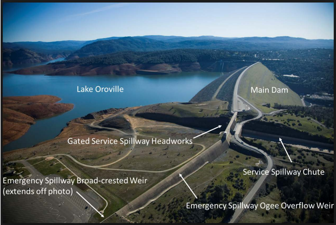
Figure 3-3: Oroville Dam emergency spillway ogee crest structure
