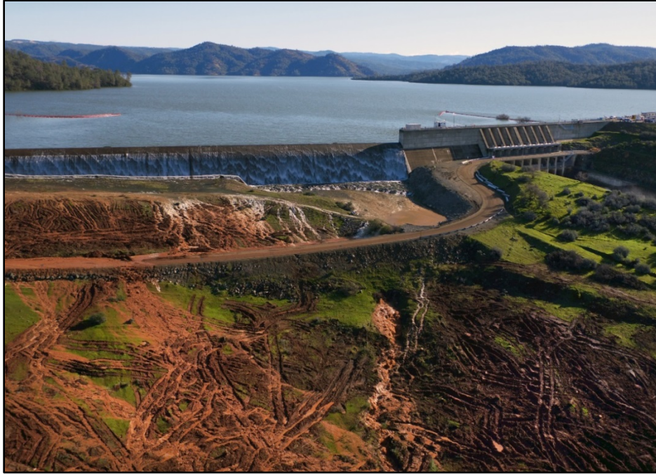
Figure 4-9: Oroville Dam emergency spillway as overflow began on February 11 (from DWR)
