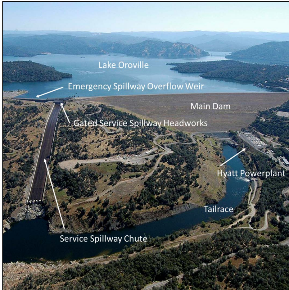
Figure 3-1: Overview of Oroville Dam facility prior to the February 2017 incident
