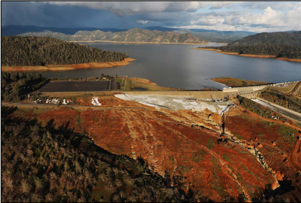
Figure 4-11: Emergency spillway after the incident (from DWR)
