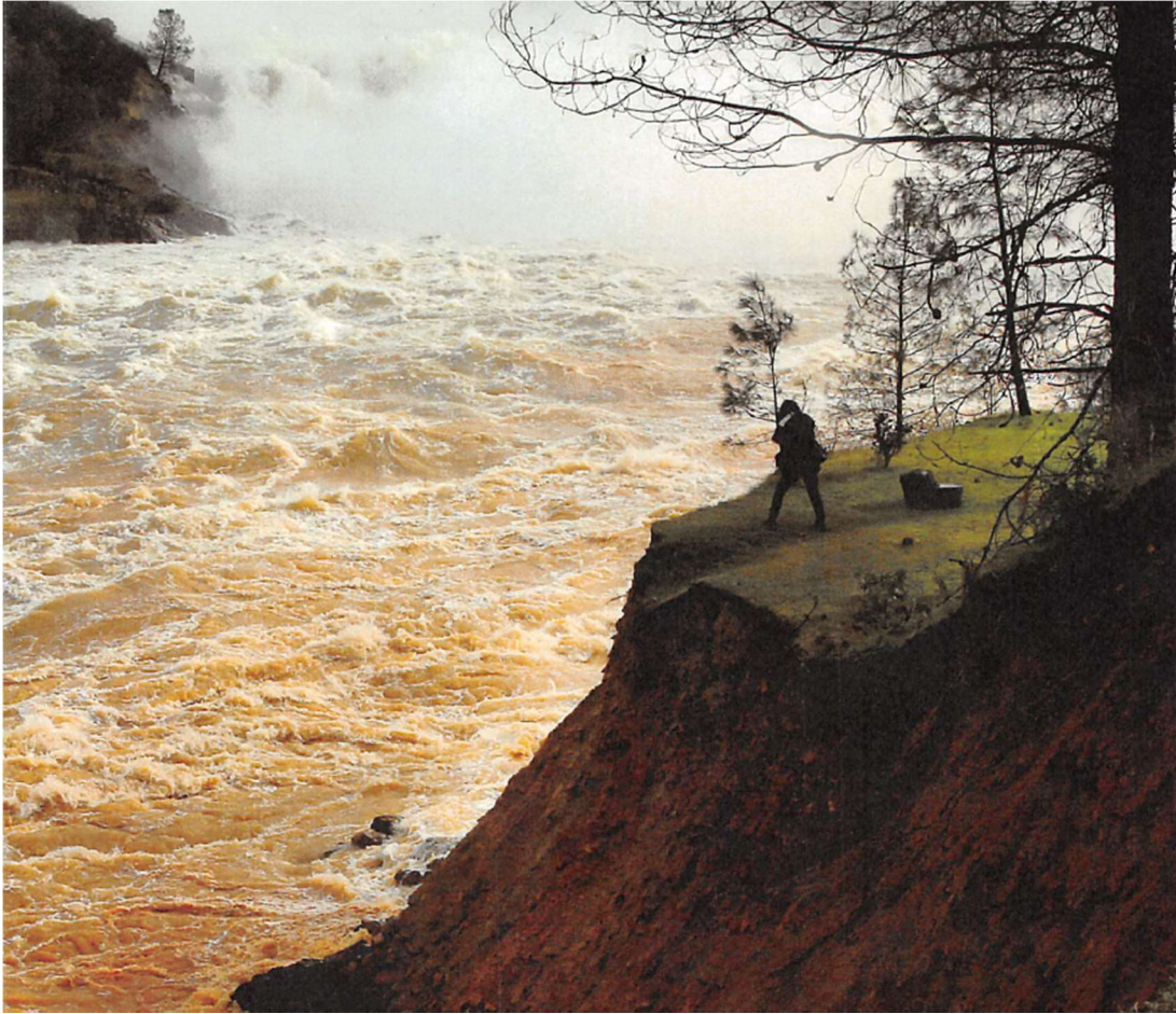
3 4 5 6 7 8 9 10 11 12 13 14 15 16 17 18 Water released down Oroville Dam spillway into the Feather River, February 13, 2017 Source: San Francisco Chronicle
