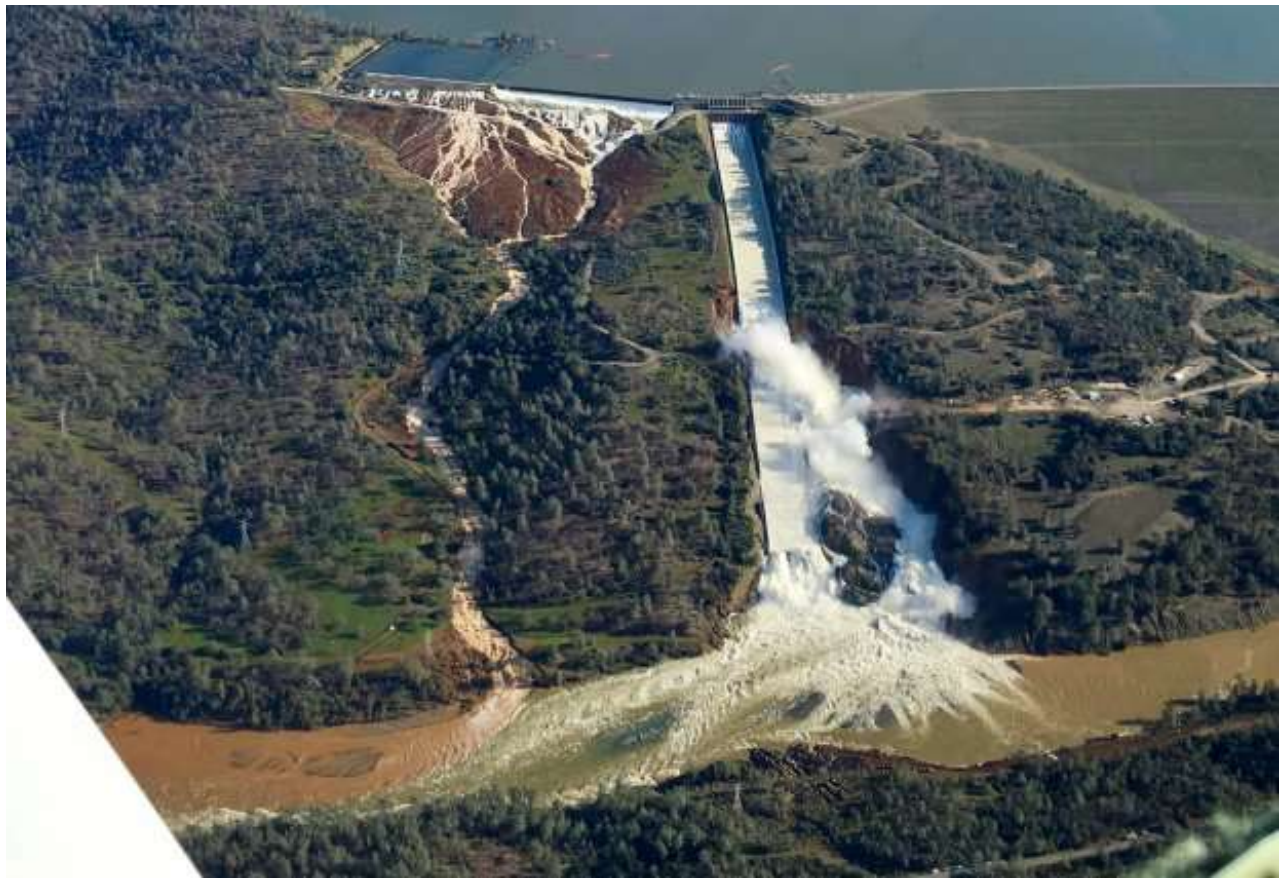
13 14 15 16 17 18 19 20 21 22 23 24 25 26 27 Water rushes down Oroville Dam’s spillways on February 12, 2017 28 Source: Chico Enterprise Record
