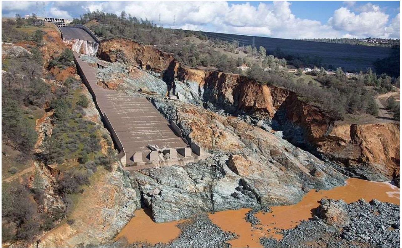
Oroville Dam spillway damage, February 27, 2017
