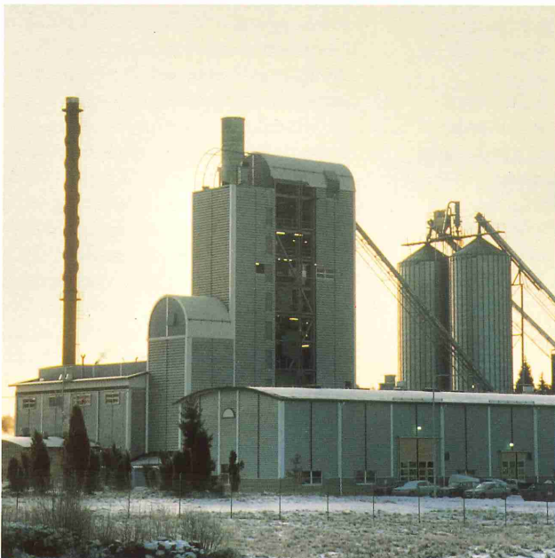
Sydkraft's BIG-GT Demonstration Plant at Varnamo, Sweden
