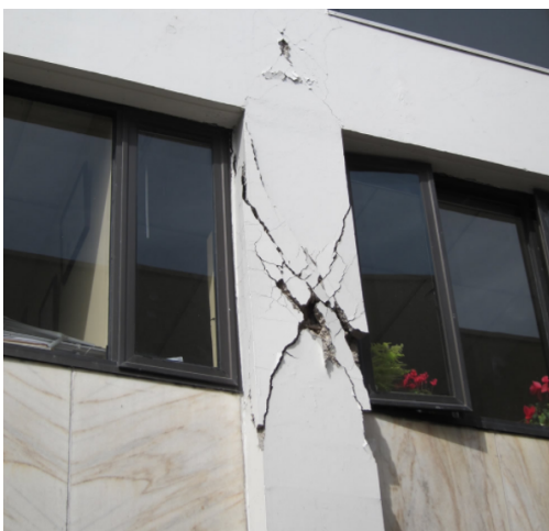
Figure 3.1: Example of shear failure of a short column, caused by influence of adjacent partial height infill (Kam, 2011) (L) and illustration of a 'short column' (R).
