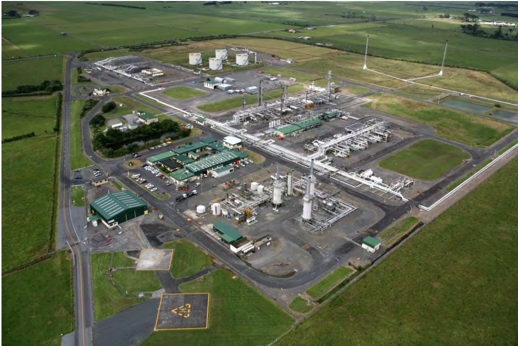
Photo 1 Maui Production Station
