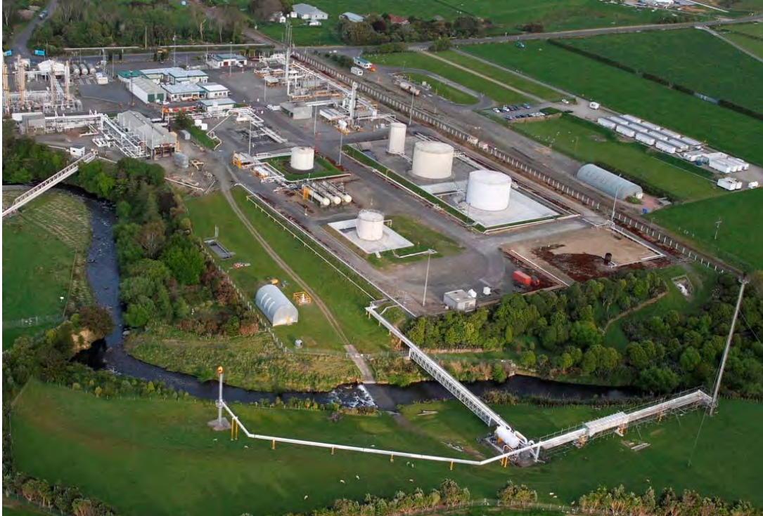
Photo 4 Kapuni Production Station
