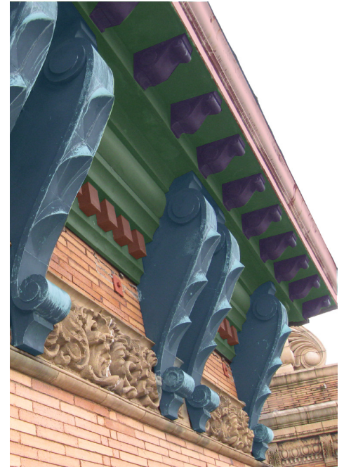
TYPICAL CORNICE ASSEMBLY SHOWN FASCIA CORBELS ENTABLATURE BRACKETS SQUARE DENTILS
