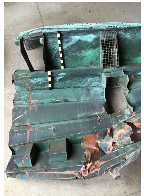
REMOVED AND DAMAGED SEGMENT OF CORNICE FRAGMENTS OF CORBEL ON TOP OPENING IN MIDDLE IS BRACKET ATTACHMENT INTACT AND MISSING DENTILS AT BOTTOM
