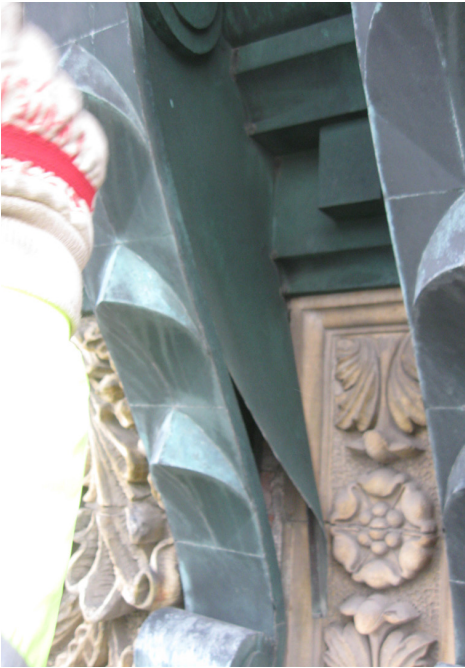
SPOT SOLDER FAILURES AT OUTSIDE CORNER SIDE COPPER HAS SEPARATED FROM FACE AND IS IN DANGER OF FAILURE
