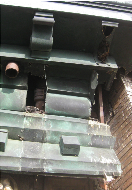
FAILED CORBEL AT TOP RIGHT TWO FAILED BRACKET LOCATIONS IN MIDDLE LOOSE DENTIL AT THE BOTTOM
