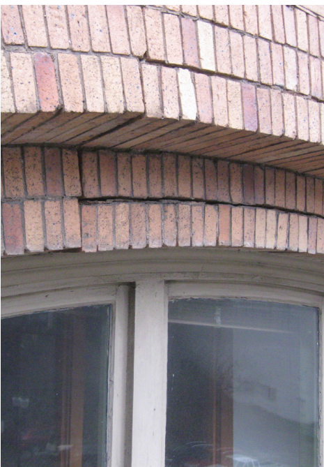
ENLARGED DETAIL OF DEFORMATION / SETTLEMENT GROUT HAS FAILED AND BRICKS HAVE SEPARATED INSIDE ARCH IS SUPPORTED BY THE WINDOW FRAME
