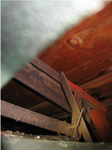
STEEL STRUCTURE AT TOP OF CORNICE SUPPORTS WOOD DECKING WITH ROOFING ABOVE
