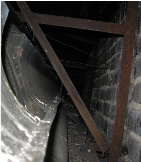
VIEW INSIDE CORNICE CAVITY STEEL BRACING FROM TOP OF CORNICE TO STRUCTURAL TIE TO MASONRY WALL
