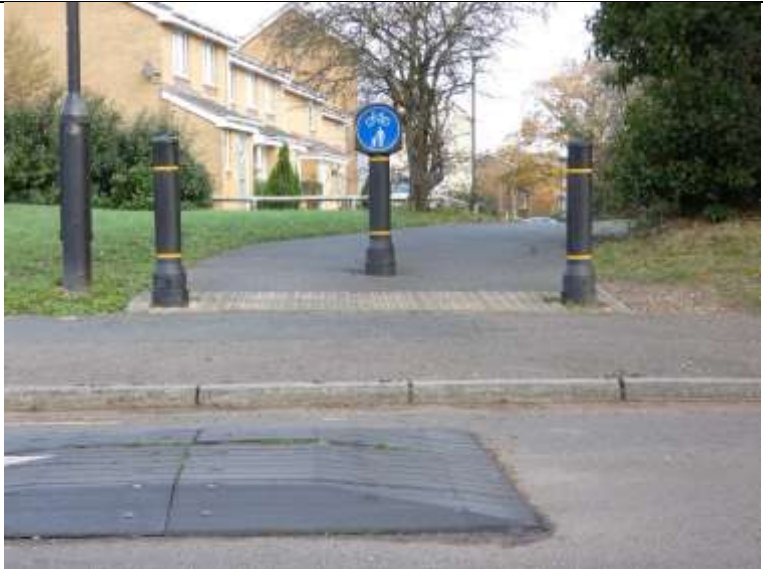
Hazel Close. Shared path joins road with no corresponding dropped kerb and “bolt on” speed hump in line. Triangle of bollards creates difficult environment to navigate, and makes it difficult to approach “tram line” tactile paving straight on.
