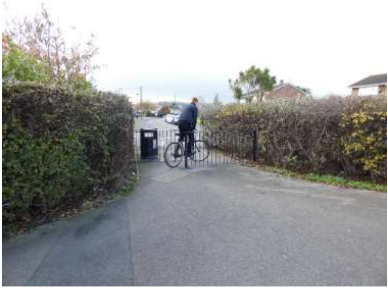
Filtered permeability at end of Kitbridge Road. Chicane barriers set <1.2m apart
