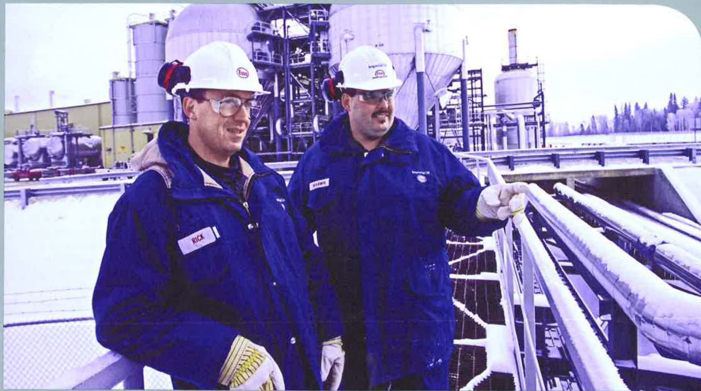
The company's Cold Lake development is one of the largest thermal heavy-oil-recovery operations in the world.
