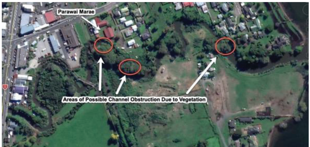
Figure 17: 2017 Aerial Photograph Ngongotahā Road Bridge to Lake Rotorua (Source - Google Earth)
