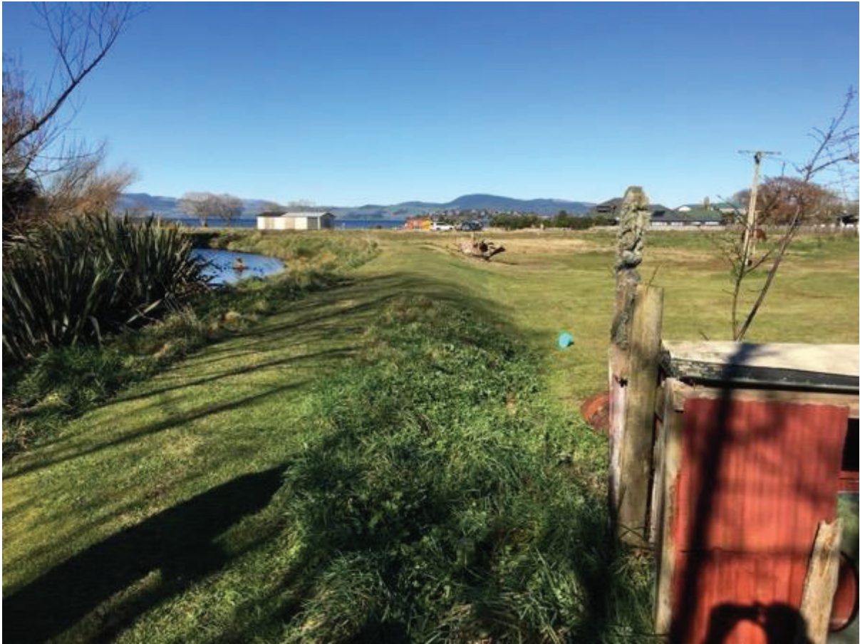
Figure 34: Right bank stopbank near Lake Rotorua
